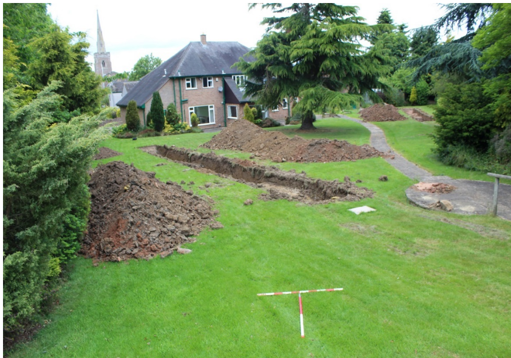
Plate 2: West facing shot of rear of site with existing building and Trenches 2 and 3 visible
