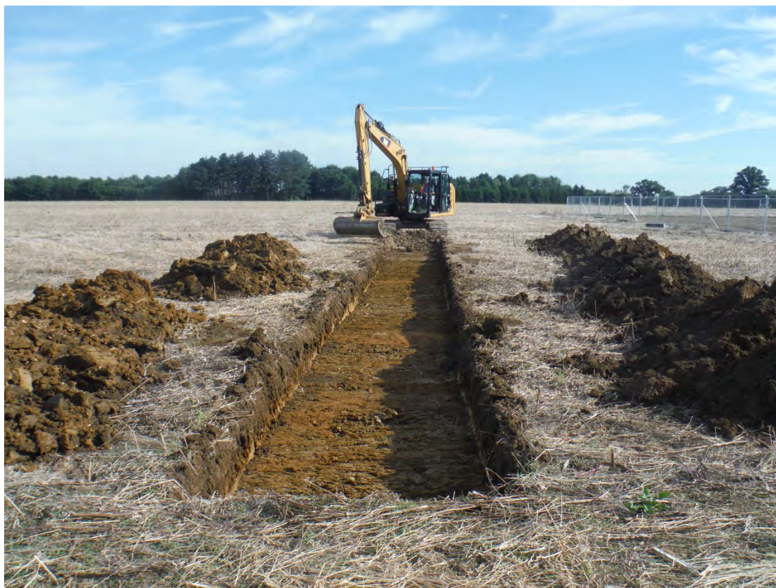
Plate 5: North facing view of the Machining of Trench 3
