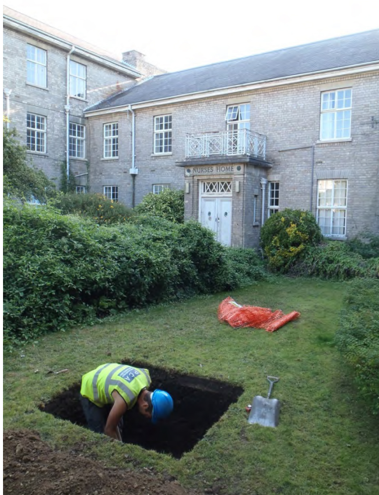
Plate 6: Test Pit 6, view north-west mid excavation
