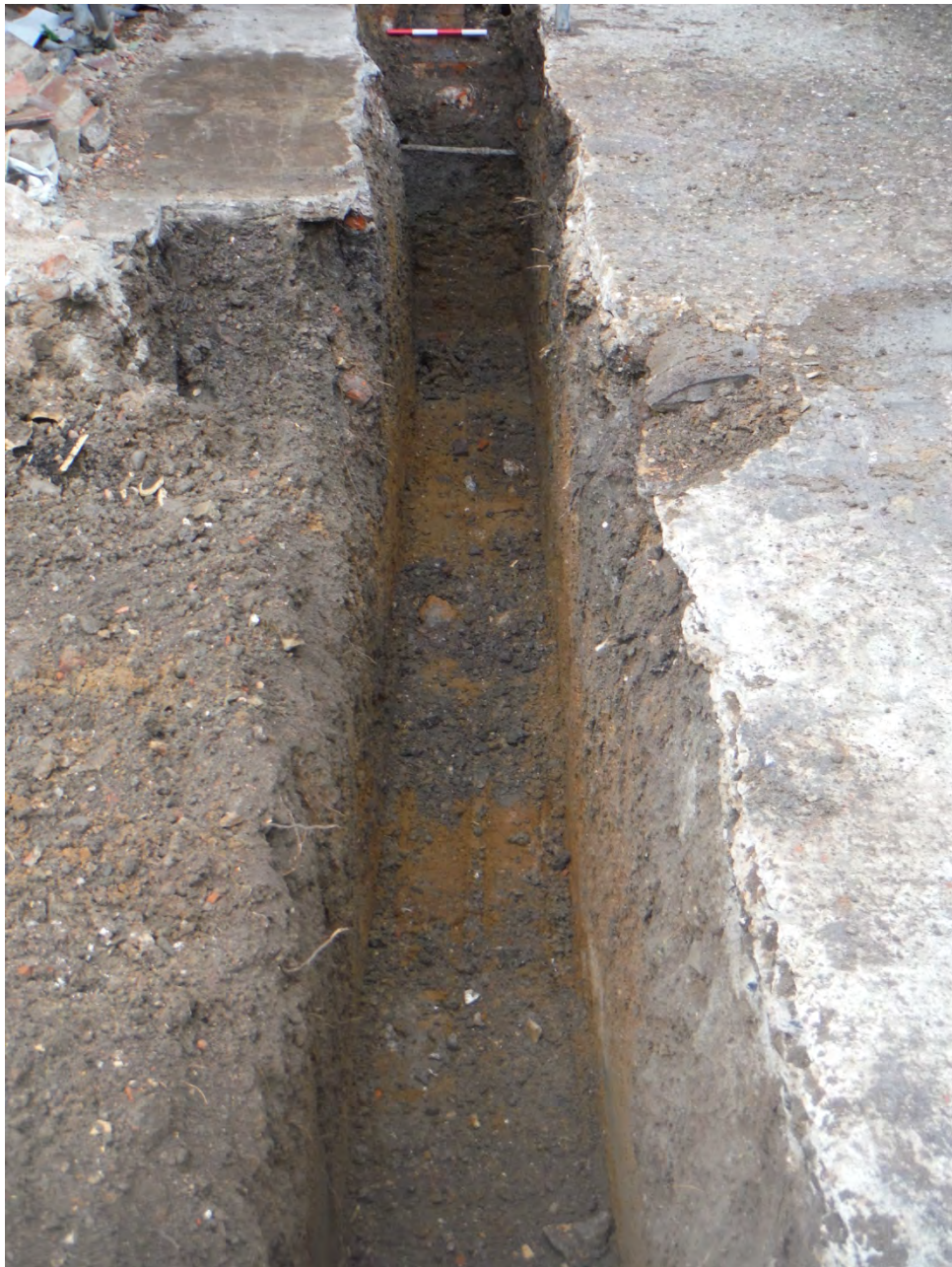
Plate 4: Southern foundation footing, view east
