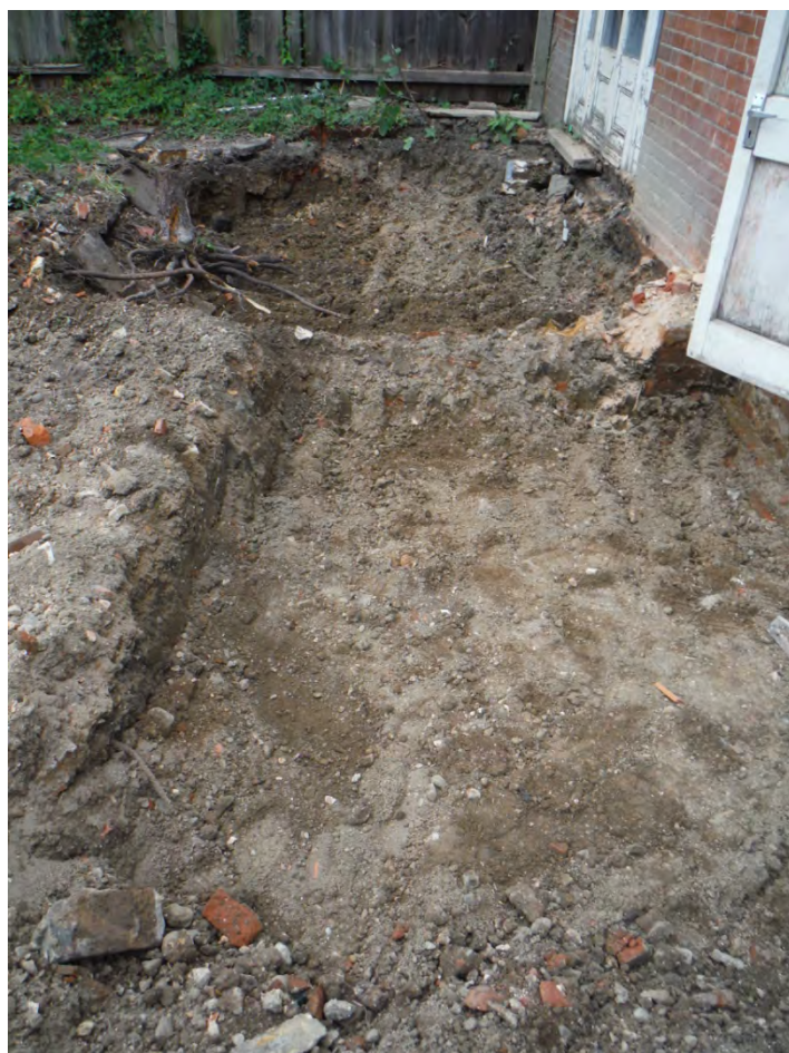
Plate 2: Initial ground reduction, view north
