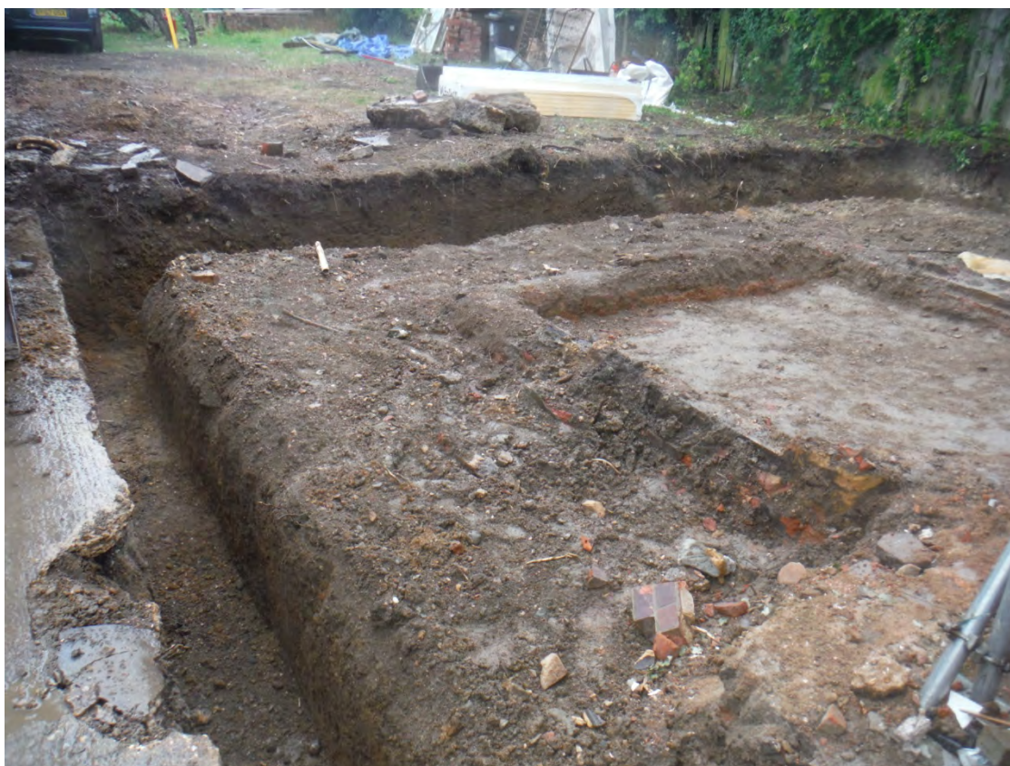
Plate 7: The site following ground reduction, view north-west
