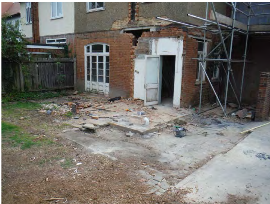
Plate 1: The site prior to groundworks, view north-east
