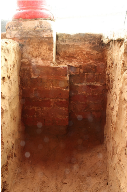
Plate 5 – Brick column base [14] for column
