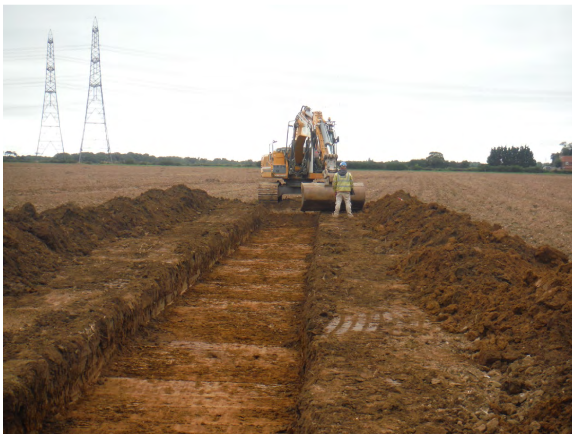
Plate 2: Trench 6, South facing view during machining
