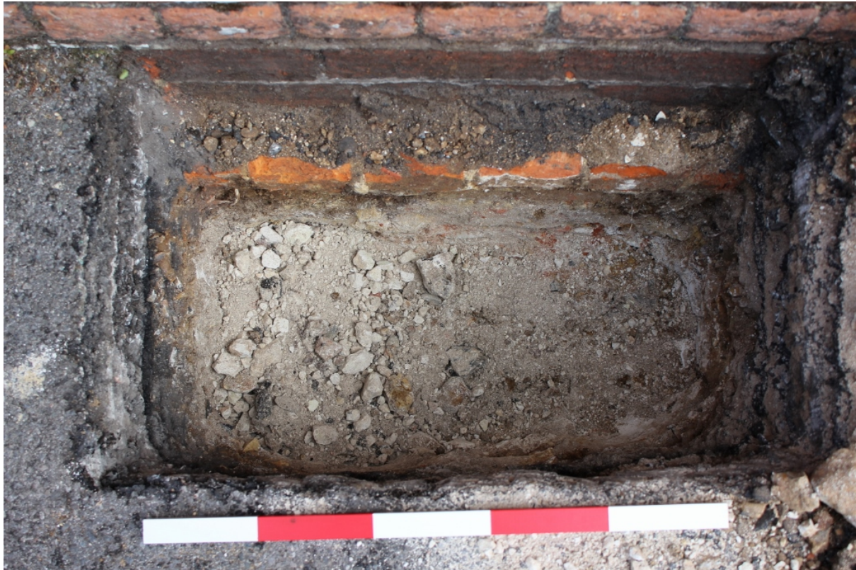
Plate 2: Geotechnical pit HP2 against south-west wall of School hall.
