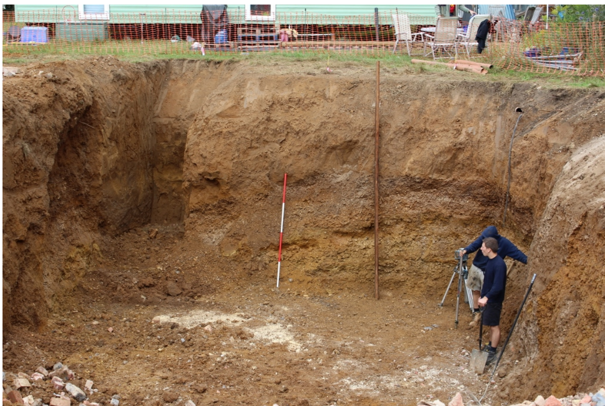
Plate 3: Basement excavation showing natural deposit sequence. View to north-west.
