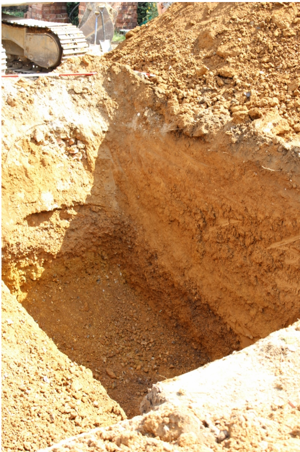
Plate 2: View of natural deposits exposed during basement excavation. View to south-east.
