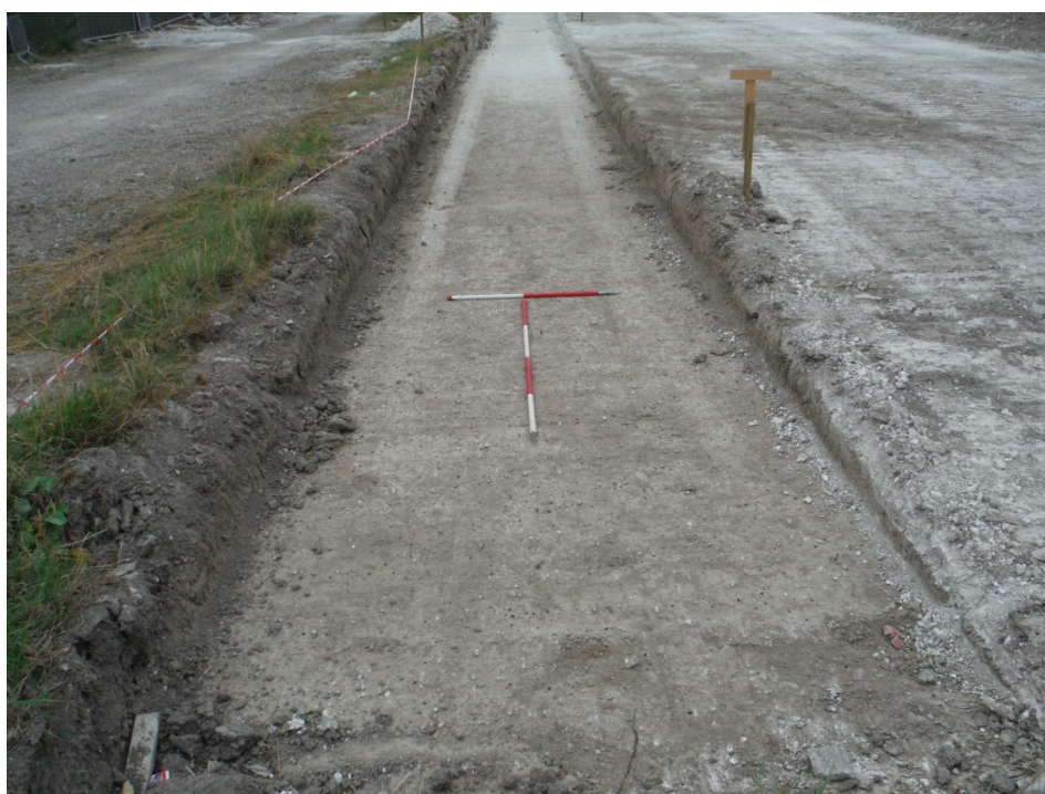
Plate 2: Post stripping of topsoil, southern area, looking northeast
