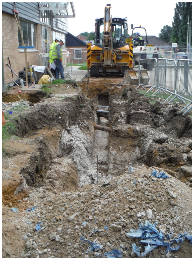
Plate 5: Excavation of drainage trench in western area, looking north
