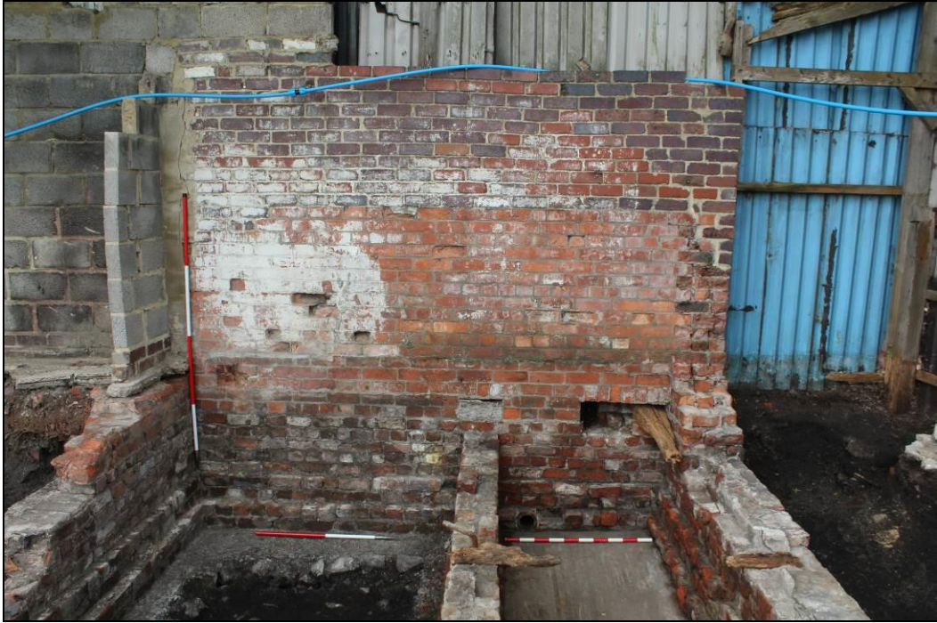
Plate 15. Internal elevation of signal box, looking ESE (2 x 1m and 1 x 2m scales)
