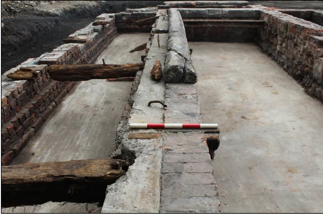
Plate 25. Iron joists in 20th-century locking room wall bonded into 19th-century signal box partition wall [254] looking north-west (0.5m scale)
