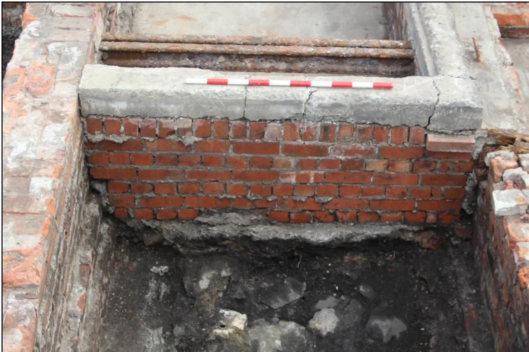
Plate 22. View of construction cut [235] for 20th-century locking room [220], looking south-east (1m scale)
