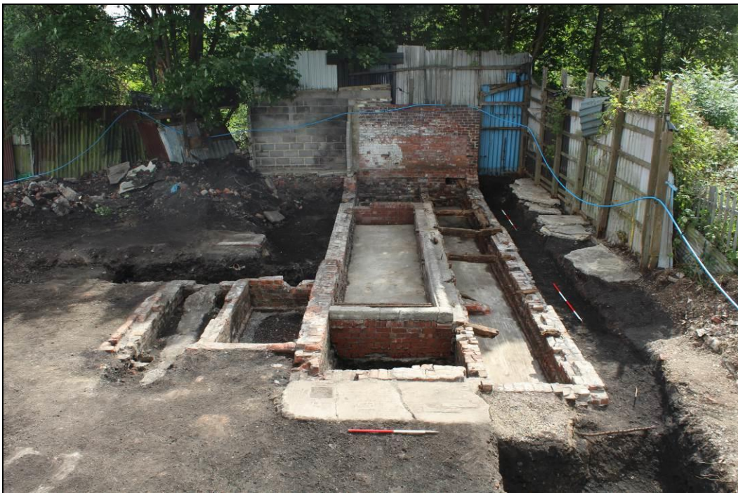
Plate 12. Overview of Trench 2, showing footprint of signal box looking south-east; the 19th-century locking room with timber beams is on the right and the smaller 20th-century locking room is on the left (1m and 2 x 2m scales)
