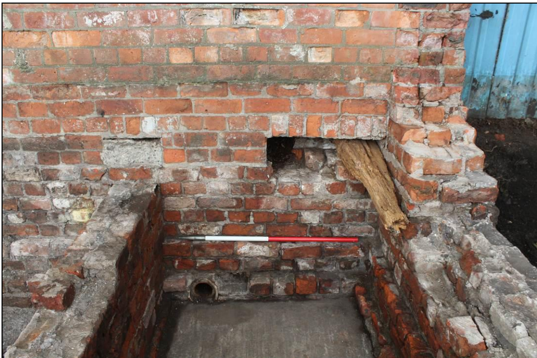
Plate 20. Timber slots within internal elevation of signal box and timber [256] looking south-east (1m scale)
