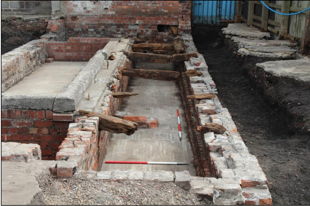
Plate 17. Overview of 19th-century locking room with timber frame, looking south-east (2 x 1m scales)
