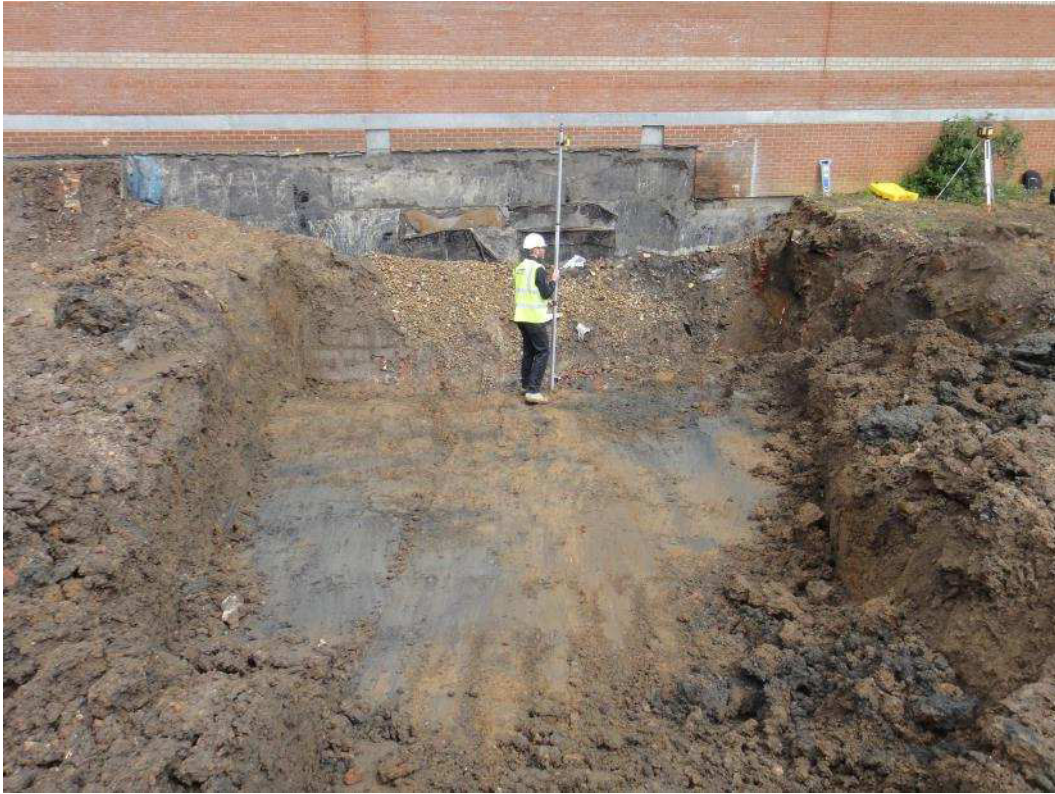
Plate 1. General view of base of northern end of Trench 6
