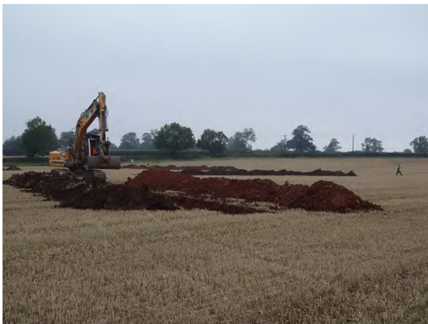
Plate 3: General view of site, view north-west.
