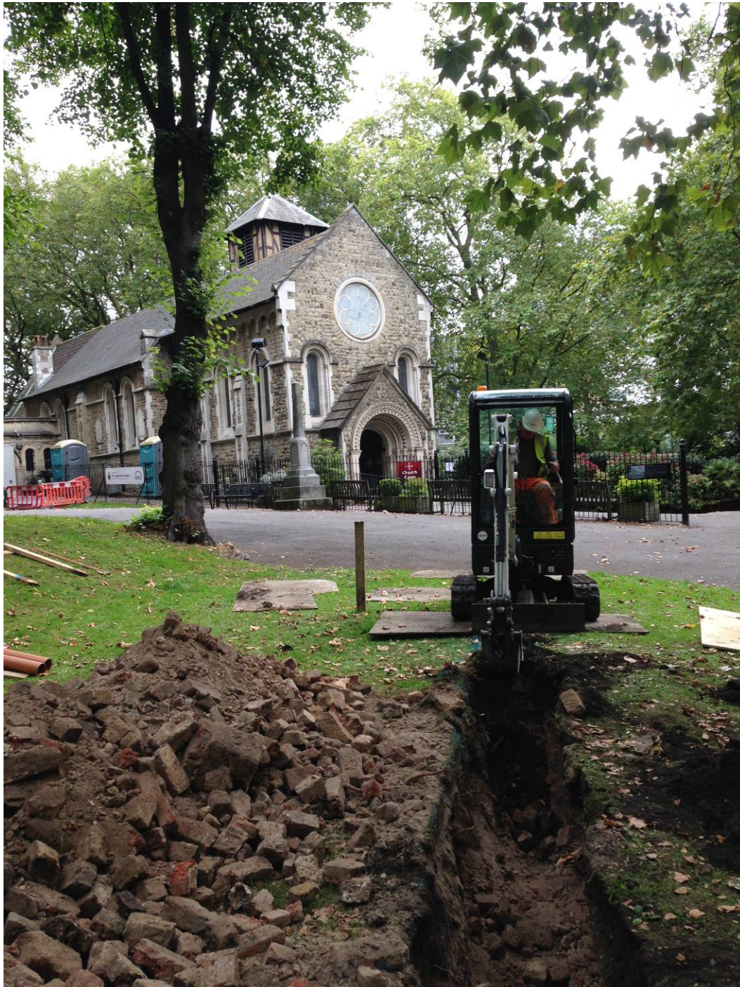
Plate 1: Trench looking south-east
