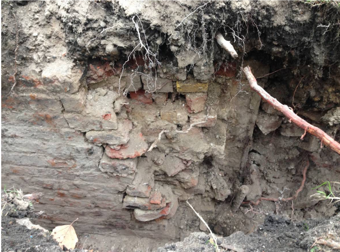
Plate 5: Wall [8] in trench section facing south
