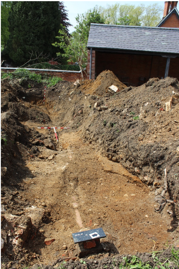
Plate 2. Trench 1, looking west. Scales 2 x 2m.
