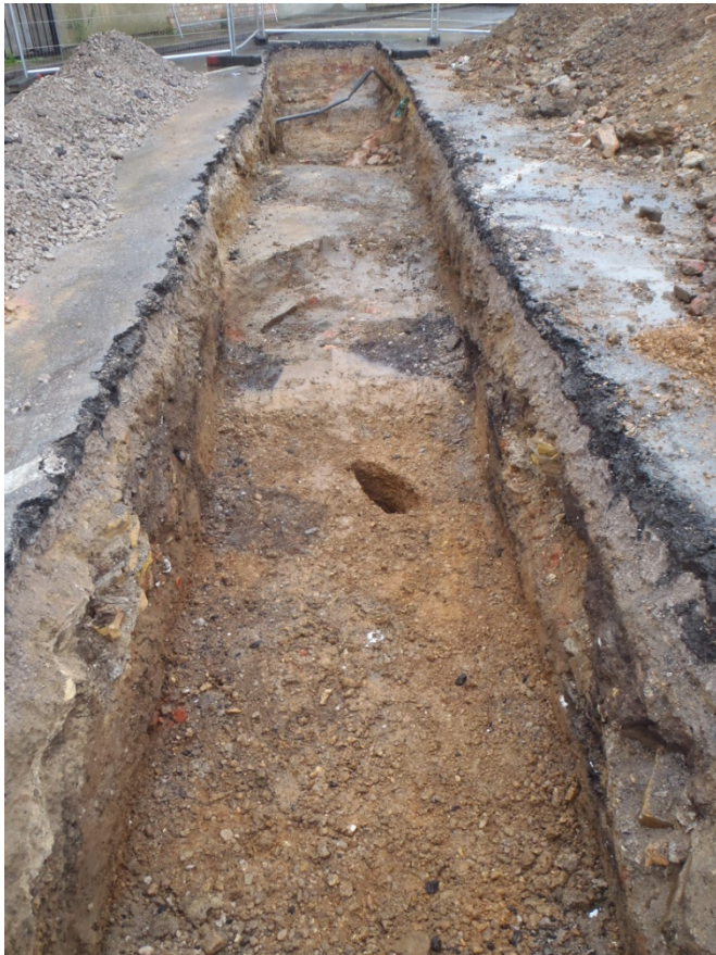
Plate 3: Trench 3, facing southeast.
