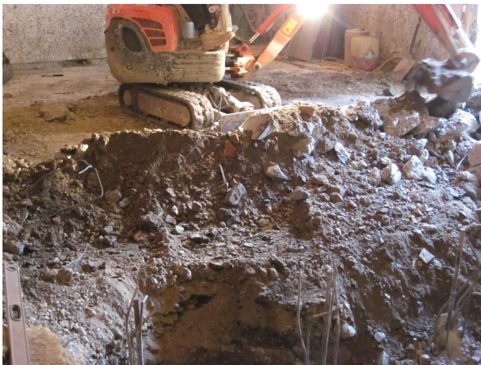
Plate 1: North West Facing View of Modern Layers being removed in Trench 1
