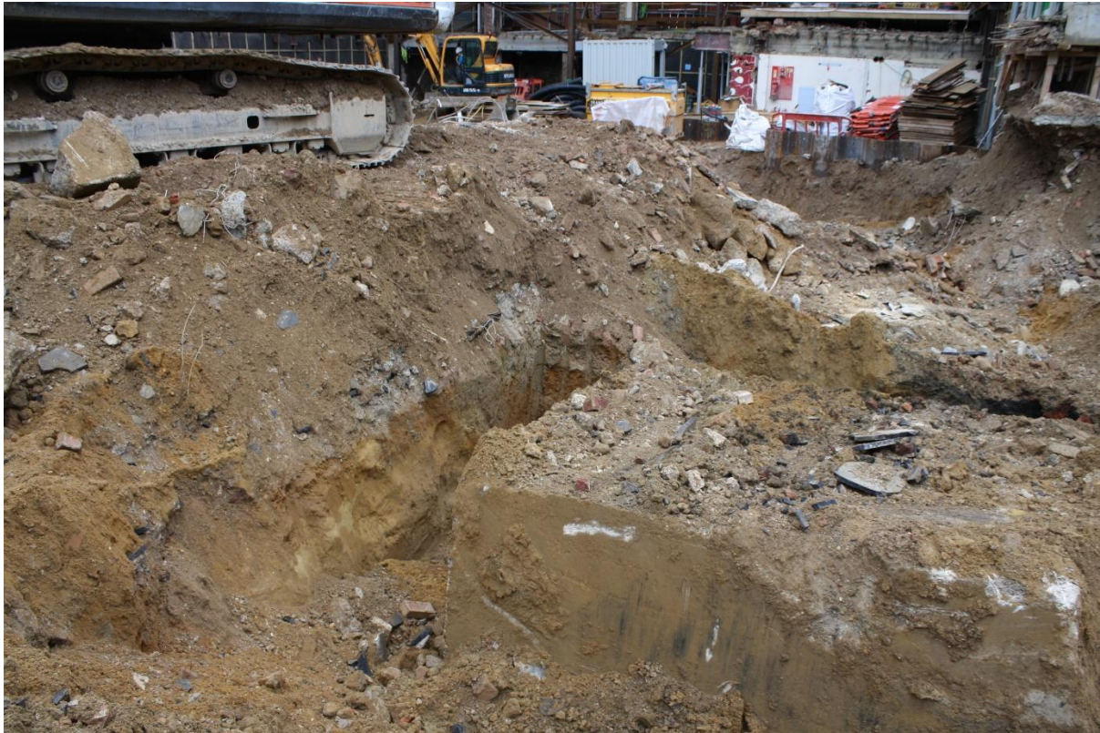
Plate 1: View South West Showing Made Ground Over Natural
