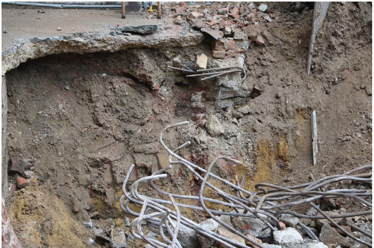
Plate 2: View North West Showing Made Ground over Natural
