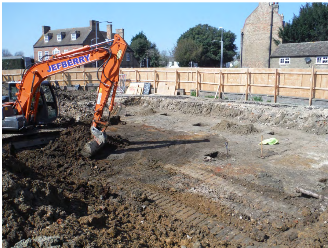
Plate 1: Test pit excavation of Layers 2 and 3, view north-west
