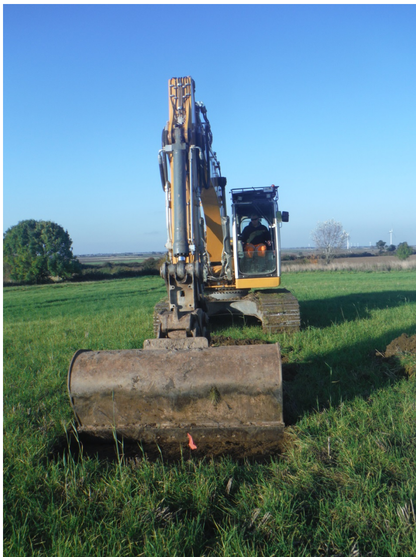
Plate 2: The site, machining, view north
