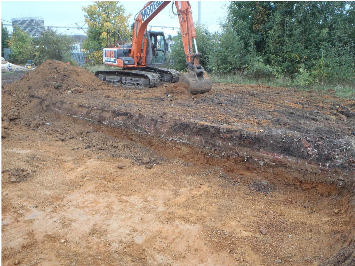
Plate 4: Railway siding [7] and natural [5] in foreground, Looking southwest
