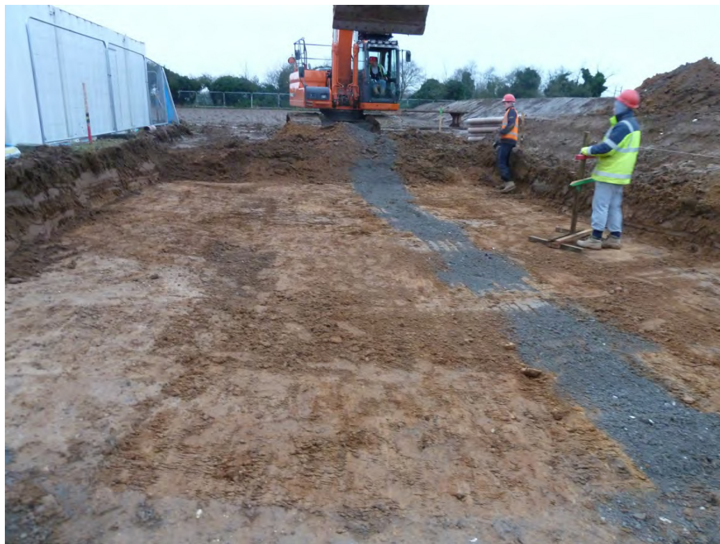
Plate 9: Monitoring of stripping for access road, view southwest.
