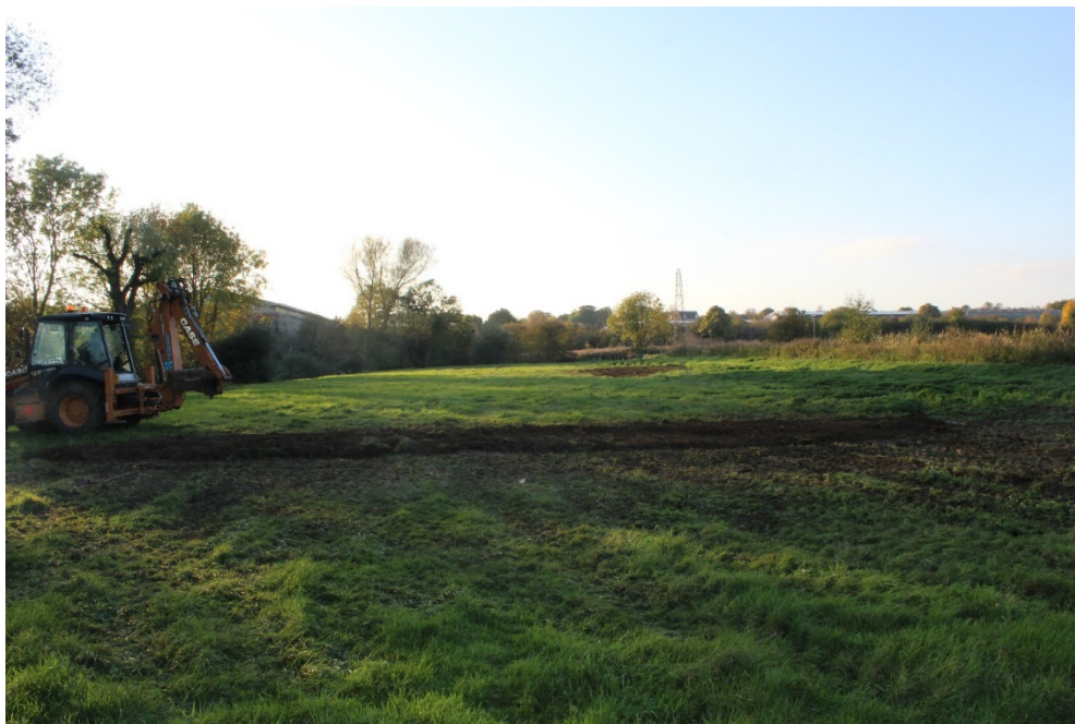
Plate 5: Machine on site after backfilling
