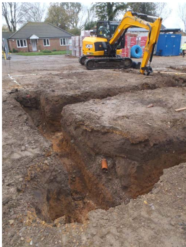
Plate 1: Excavation of footings, view north.
