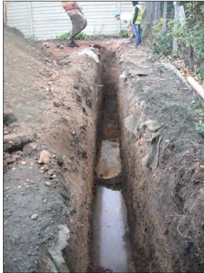
Plate 1: Southern Foundation Trench, Looking East
