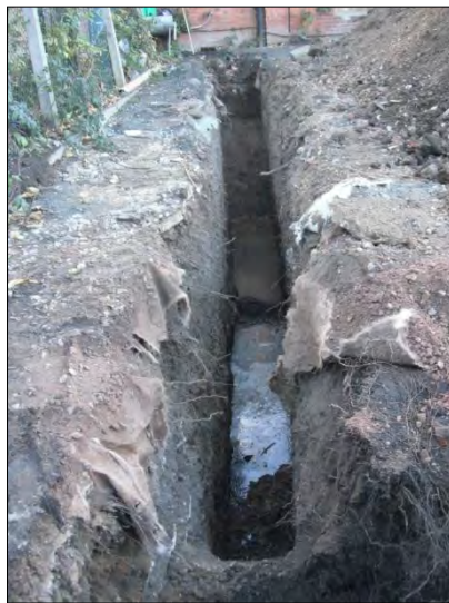
Plate 2: Southern Foundation Trench, Looking West
