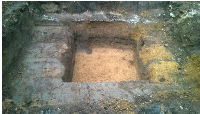
Plate 3: Trench 3 (Looking North) Showing Made Ground Over Natural
