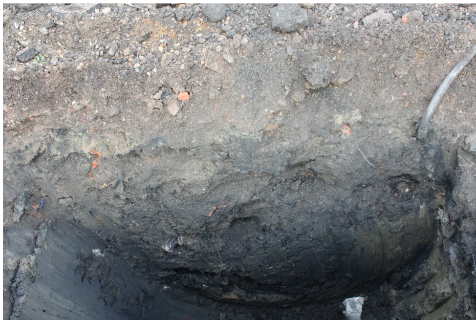
Plate 6: TP6, Looking SE
