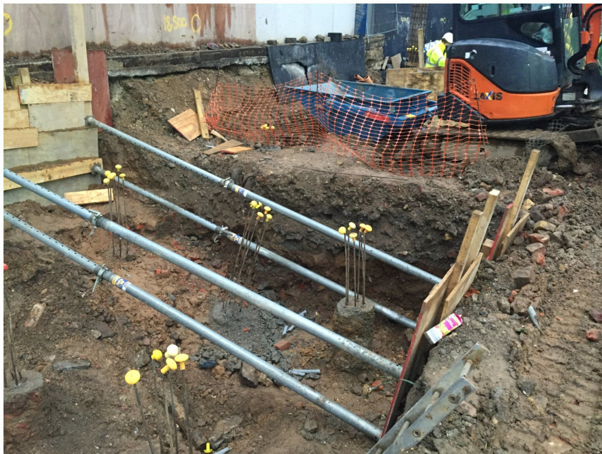
Plate 5: Pile Cap 10, northwest facing
