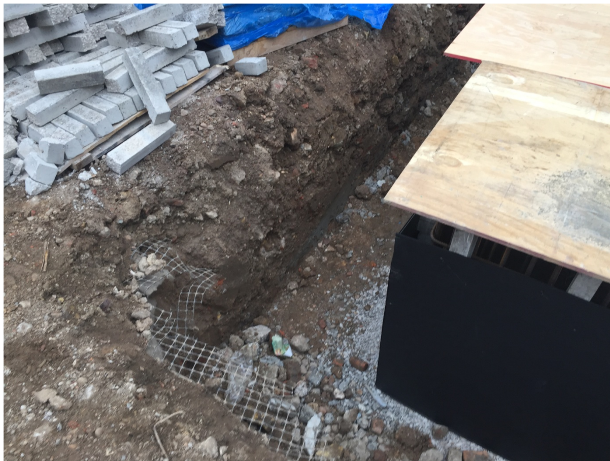
Plate 4: Pile Cap 6, northwest facing
