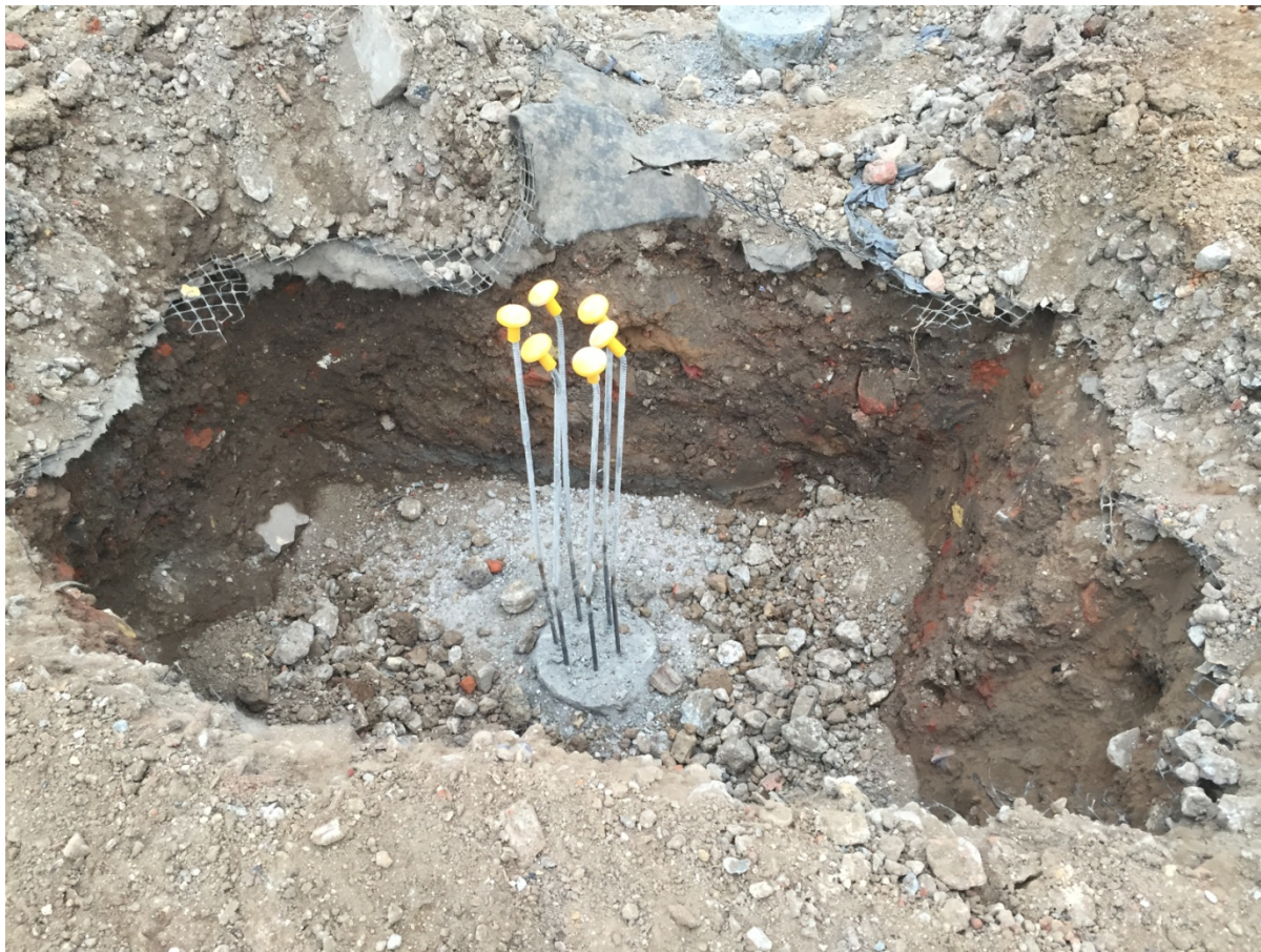
Plate 1: Pile Cap 1, facing west
