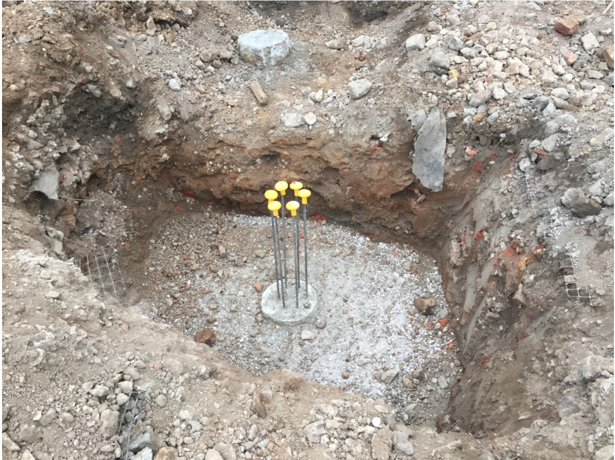
Plate 2: Pile Cap 2, facing west
