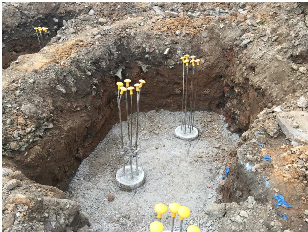
Plate 3: Pile Cap 4, facing south
