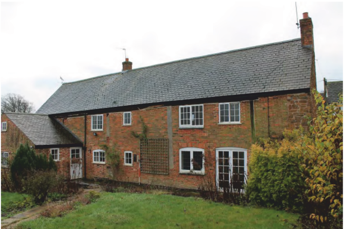
Plate 17 Priory Farmhouse, rear elevations, looking south-east
