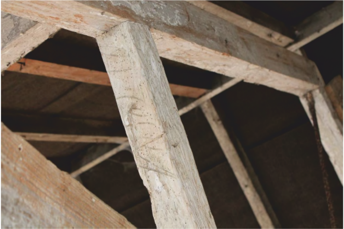
Plate 6 Baltic marks on raking strut in (A1)
