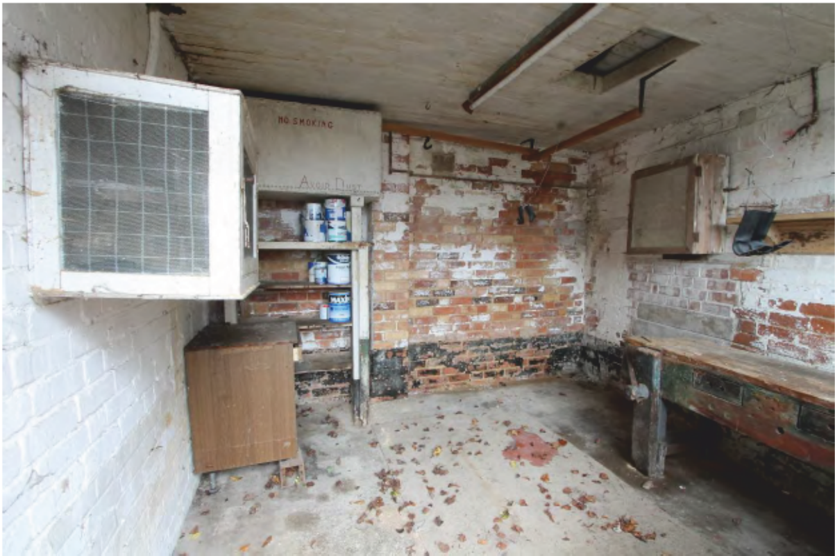
Plate 11 Room (B1) looking west
