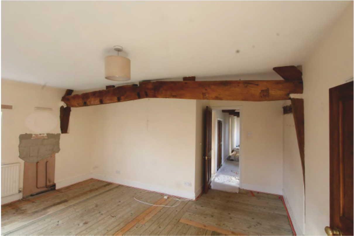
Plate 24 Tie beam in eastern bedroom, showing internal blockwork to south wall
