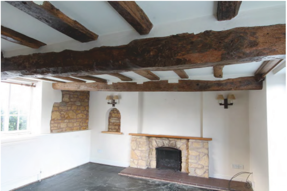
Plate 21 Western end room (Bays 1-2) looking south-west
