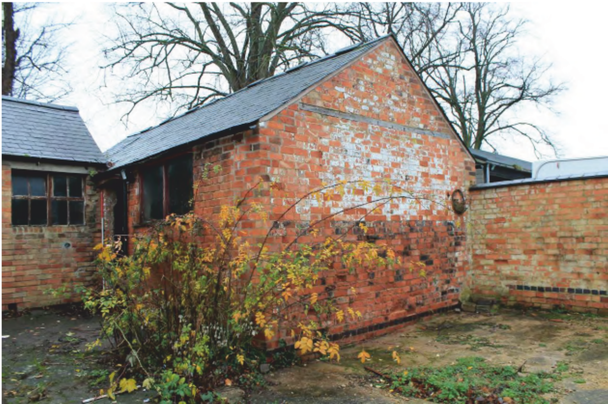
Plate 1 Cow shed (A) looking north-west
