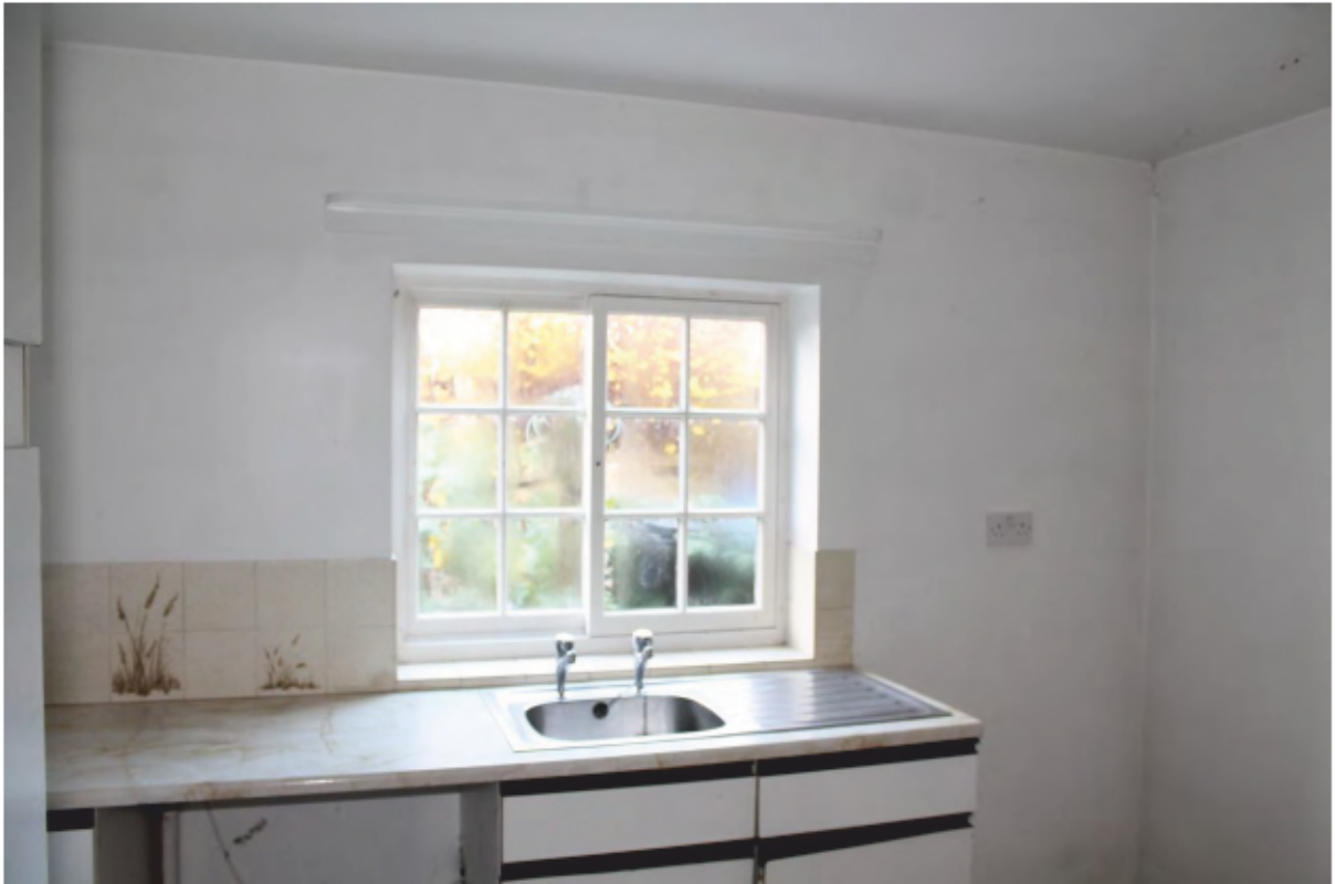
Plate 32 Interior of rear extension/dairy
