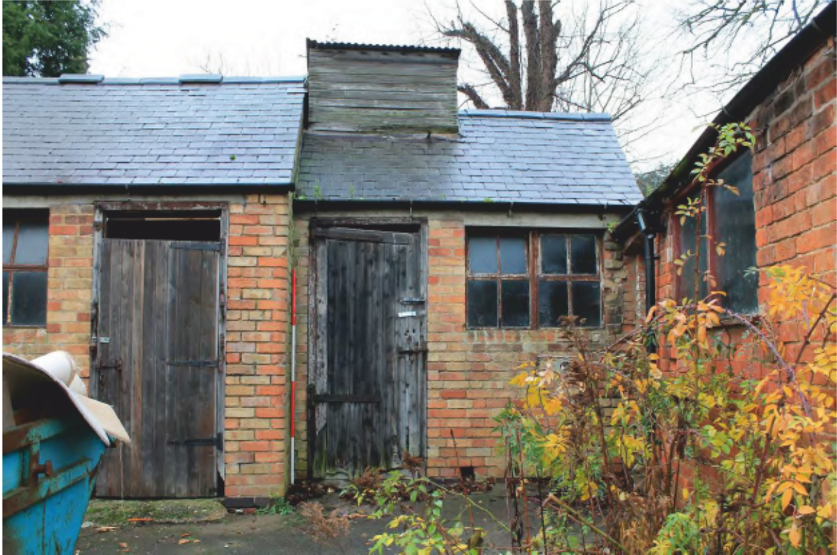
Plate 9 Building (B) northern end, looking west
