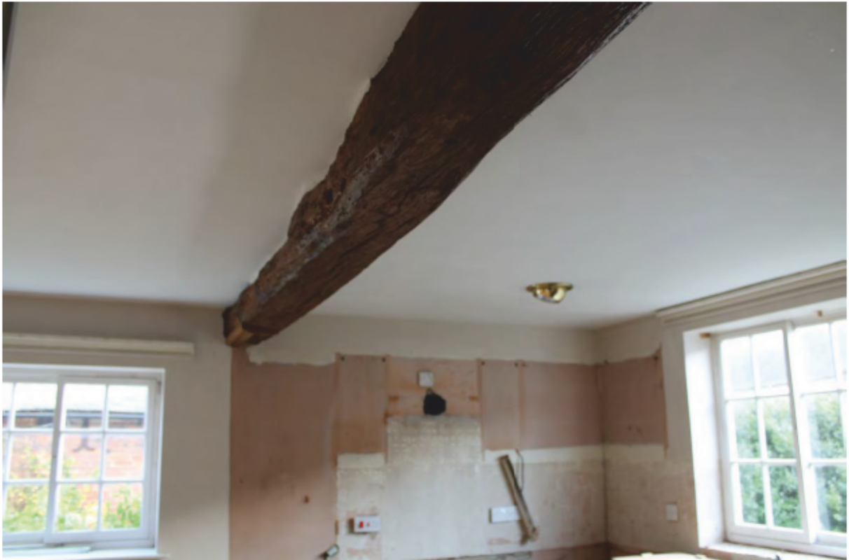
Plate 22 Axial bridging joist in Kitchen (7) looking east
