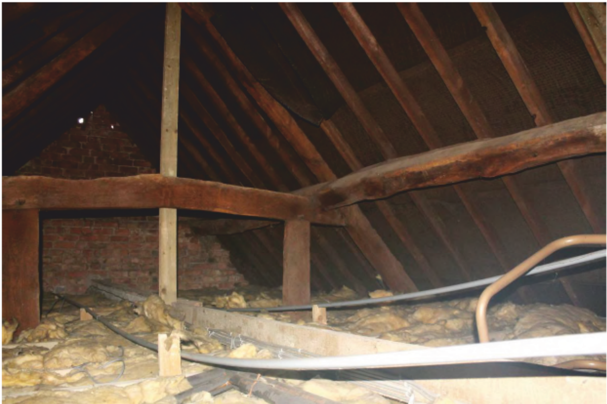
Plate 27 Un-braced roof over eastern part, looking south-east
