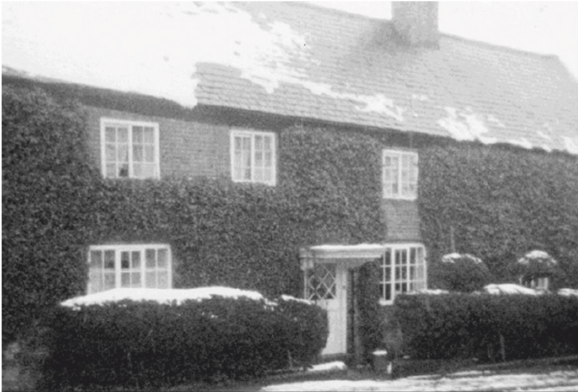
Priory Farm, 41, Main Street, is a 16th century Grade II listed building, formerly known as Ivy Cottage. It is a rectangular house built partly of ironstone with a timber framed upper storey, later faced with brick. The use of differing materials indicates that the house was built in stages over many years.
