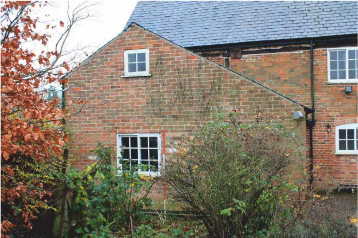
Plate 30 Rear extension looking south
