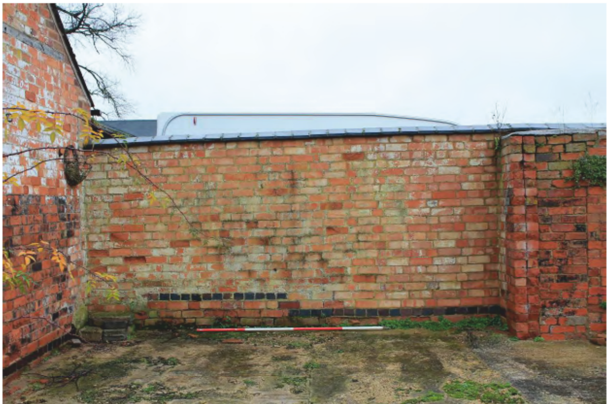
Plate 13 Remains of former shed (western part) looking north
