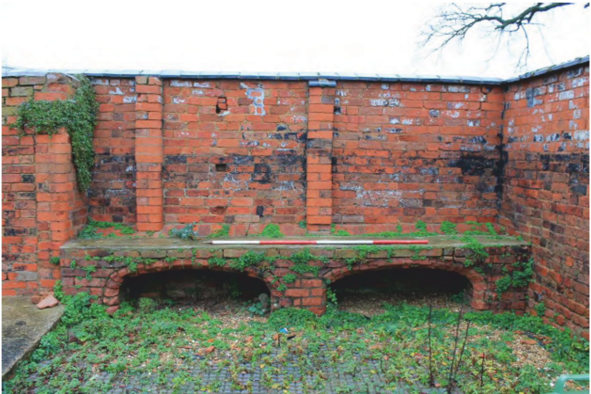
Plate 14 Base of mangers within demolished eastern part, looking north
