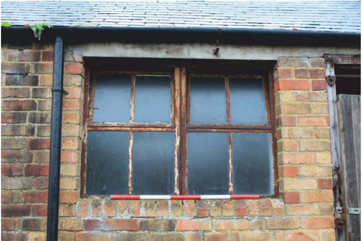
Plate 10 Building (B) typical window
