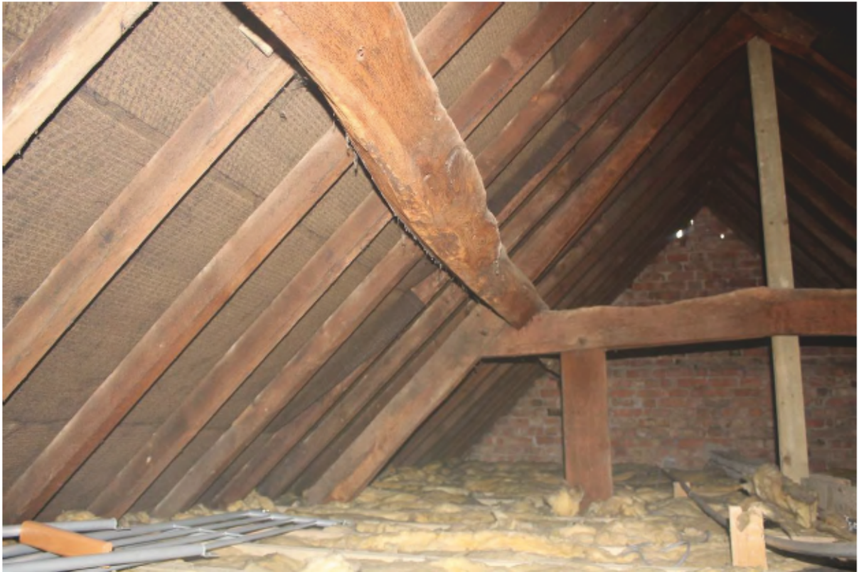
Plate 28 Un-braced roof over eastern part, looking east, showing C19 rafters
