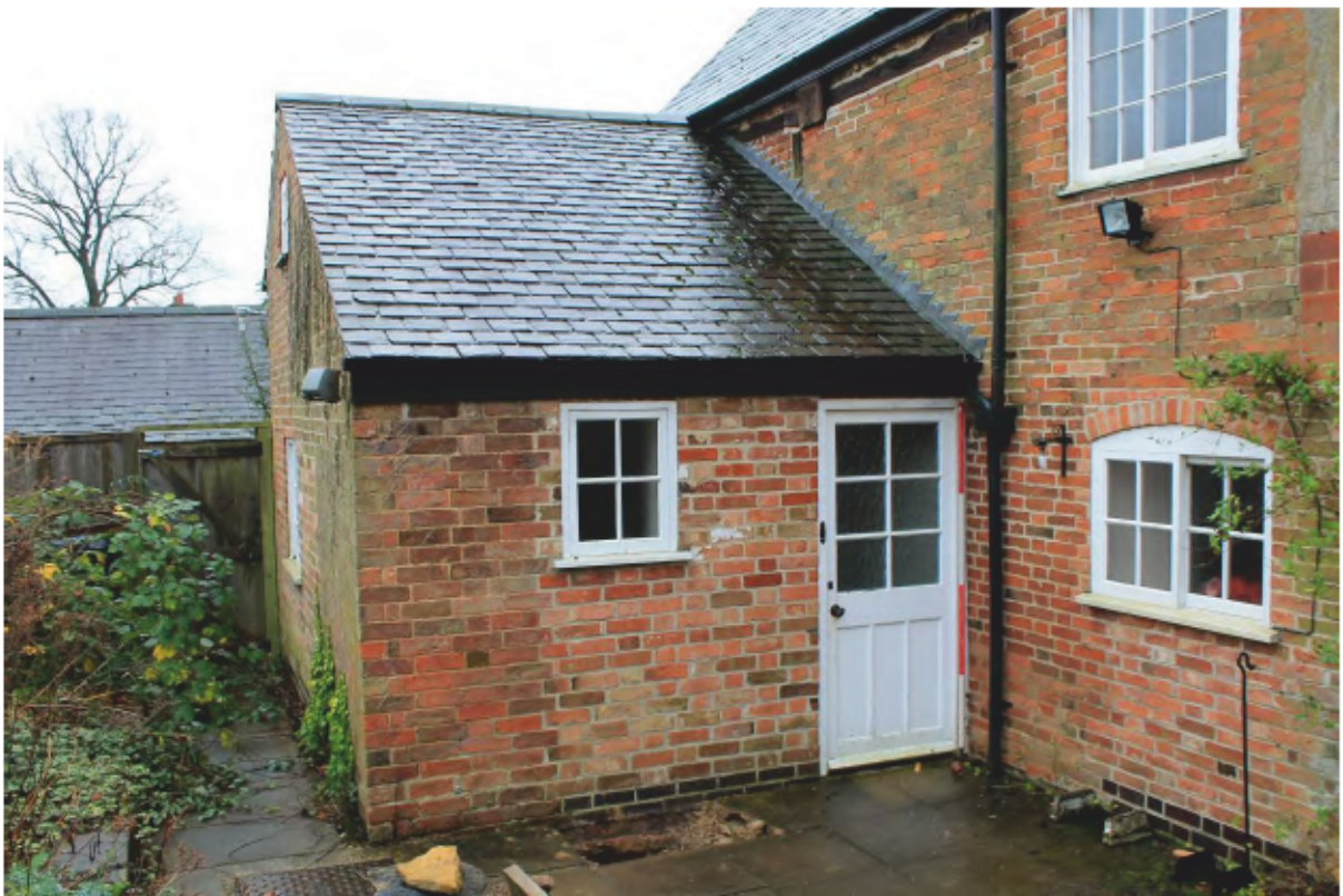
Plate 31 Rear extension looking east, showing modern rebuilding
