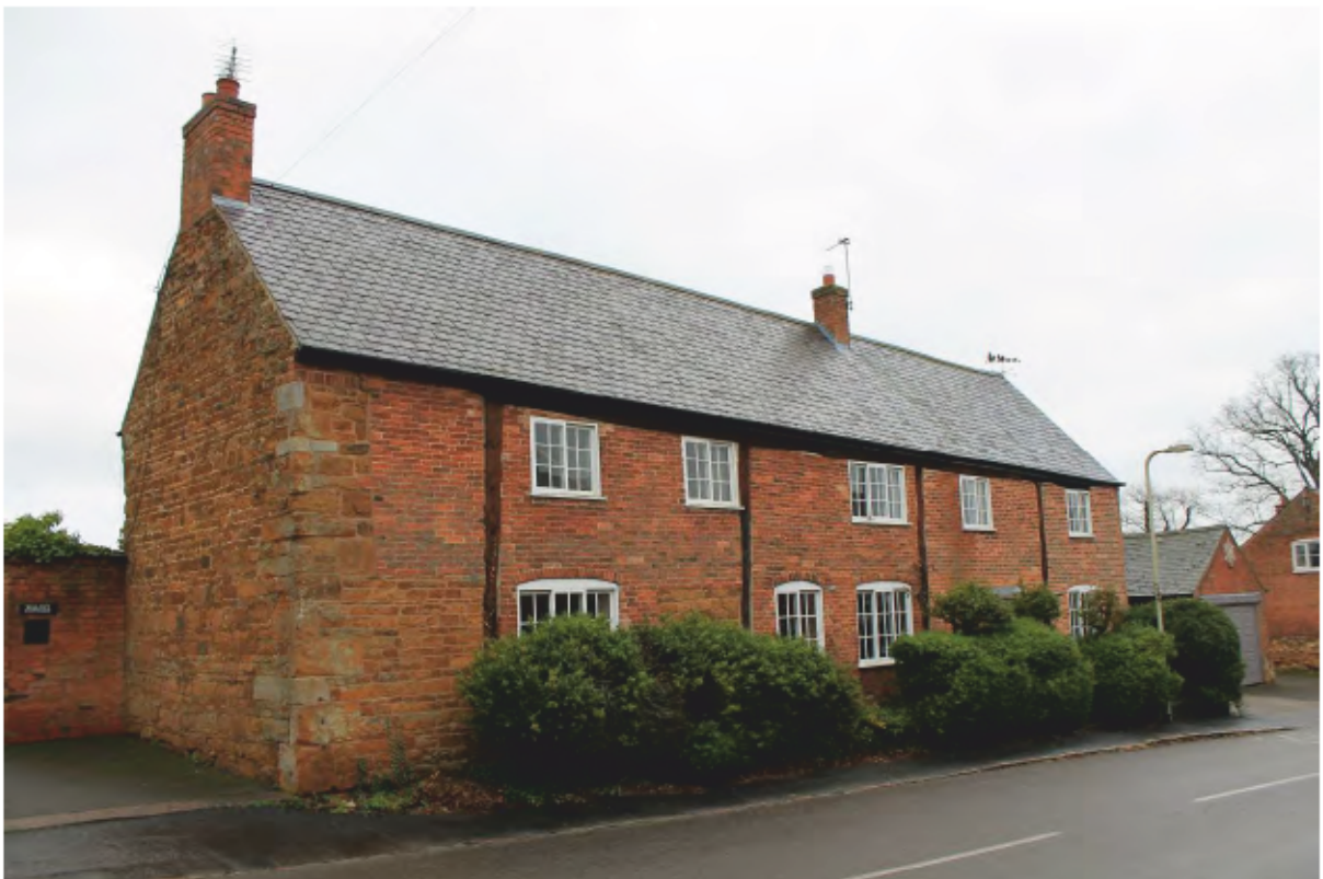
Plate 15 Priory Farmhouse looking north-east
