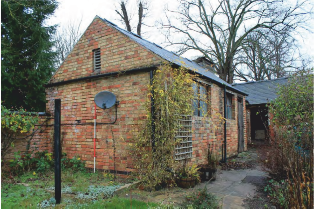
Plate 8 Cow shed (B) looking north-west
