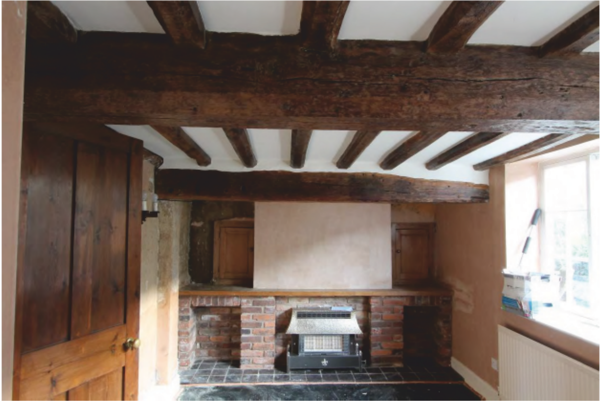
Plate 20 Heavy scantling binding joists, looking towards fireplace (bays 2-4)
