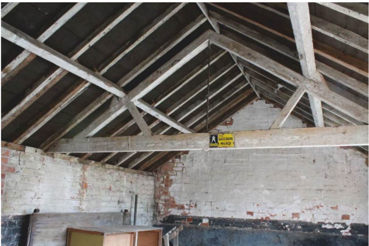
Plate 5 Detail of softwood truss and roof (A1)
