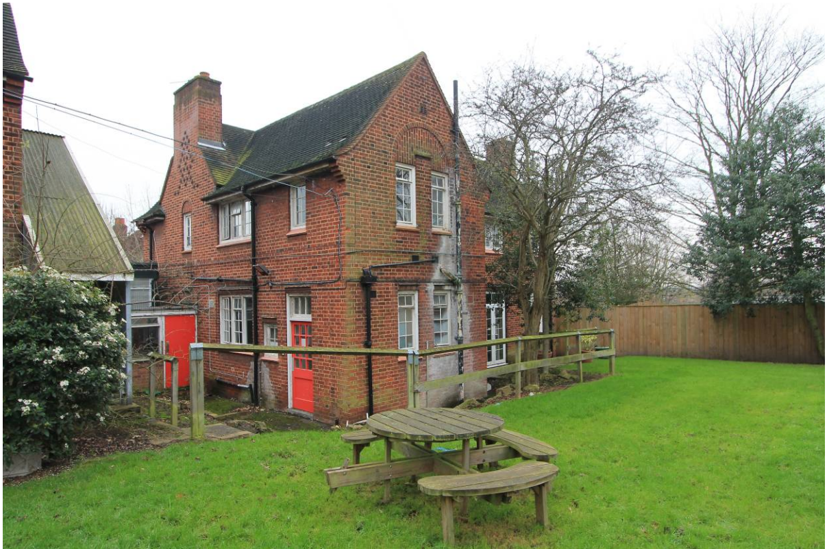
Plate 5 Western Villa rear elevations looking south-west
