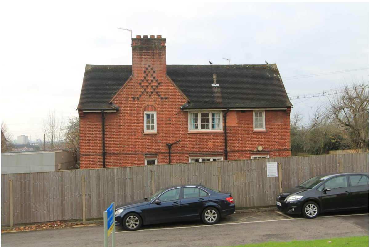
Plate 10 Eastern end elevation to Eastern Villa, looking west
