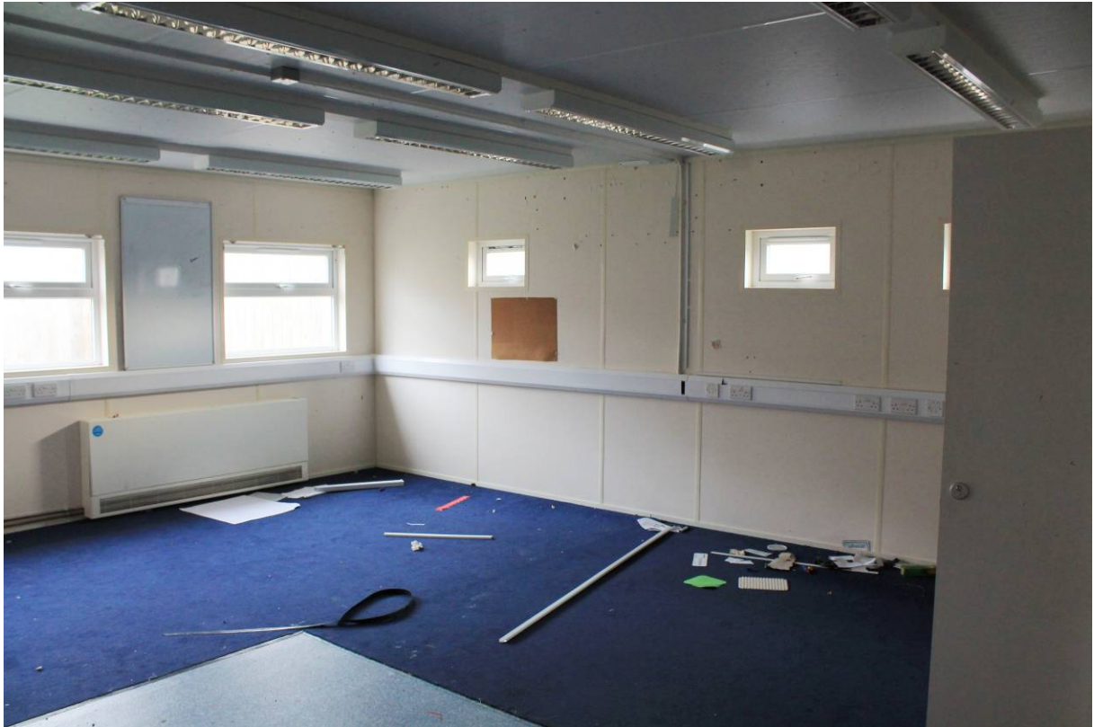
Plate 25 Modern flat roofed extension looking south-east
