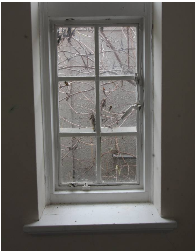
Plate 24 Typical example of metal casement
