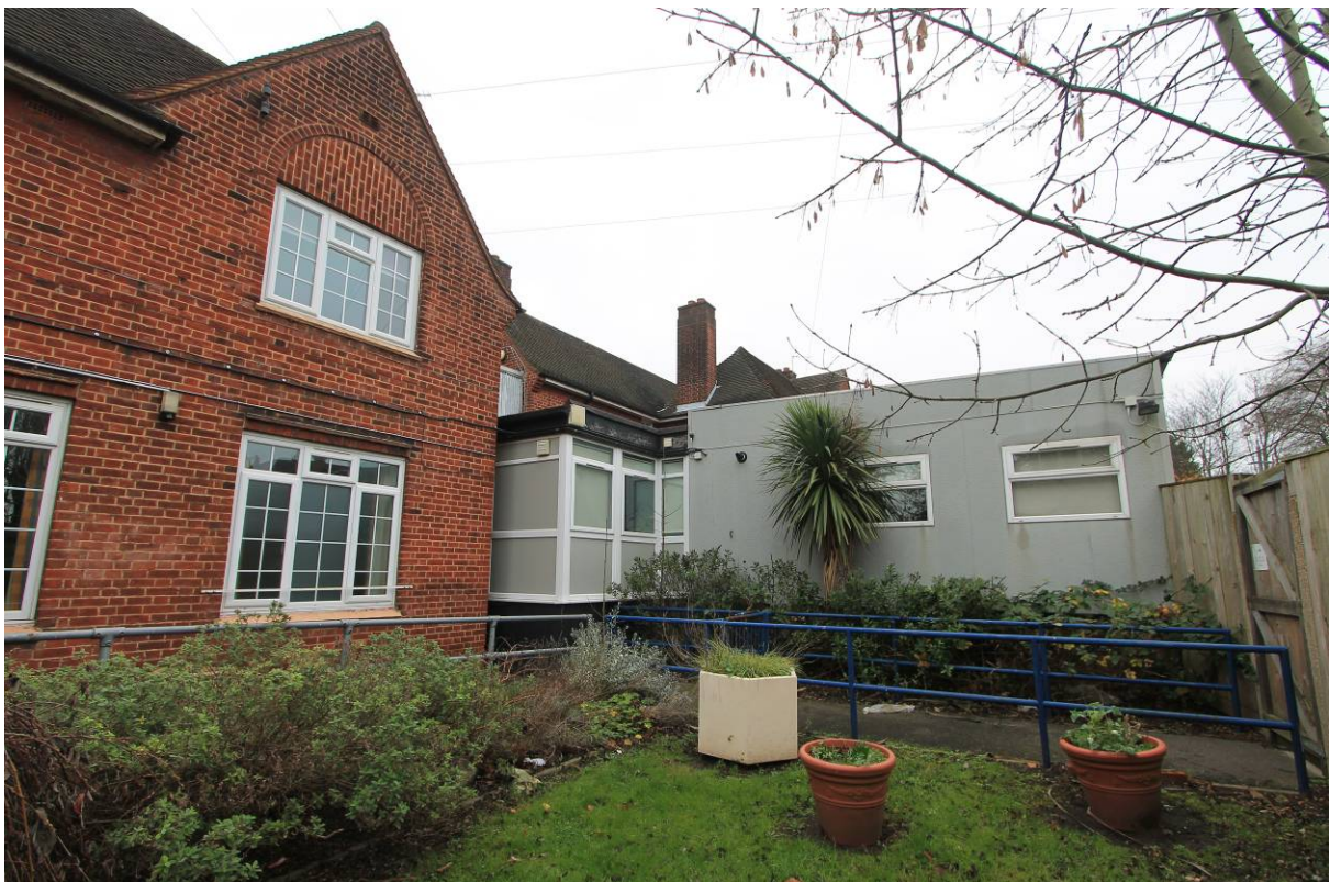
Plate 2 Modern flat-roofed extension to the front (south) of Eastern Villa
