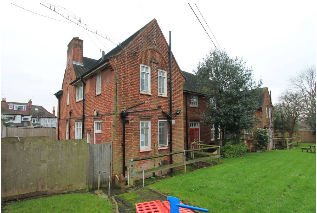
Plate 8 Rear elevations looking south-west
