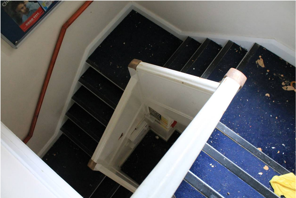
Plate 23 Open well stair in Eastern Villa
