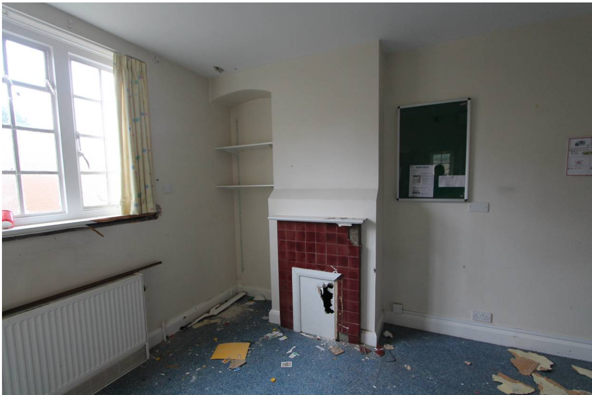
Plate 20 Eastern Villa, ground floor former kitchen (14) looking south-east
