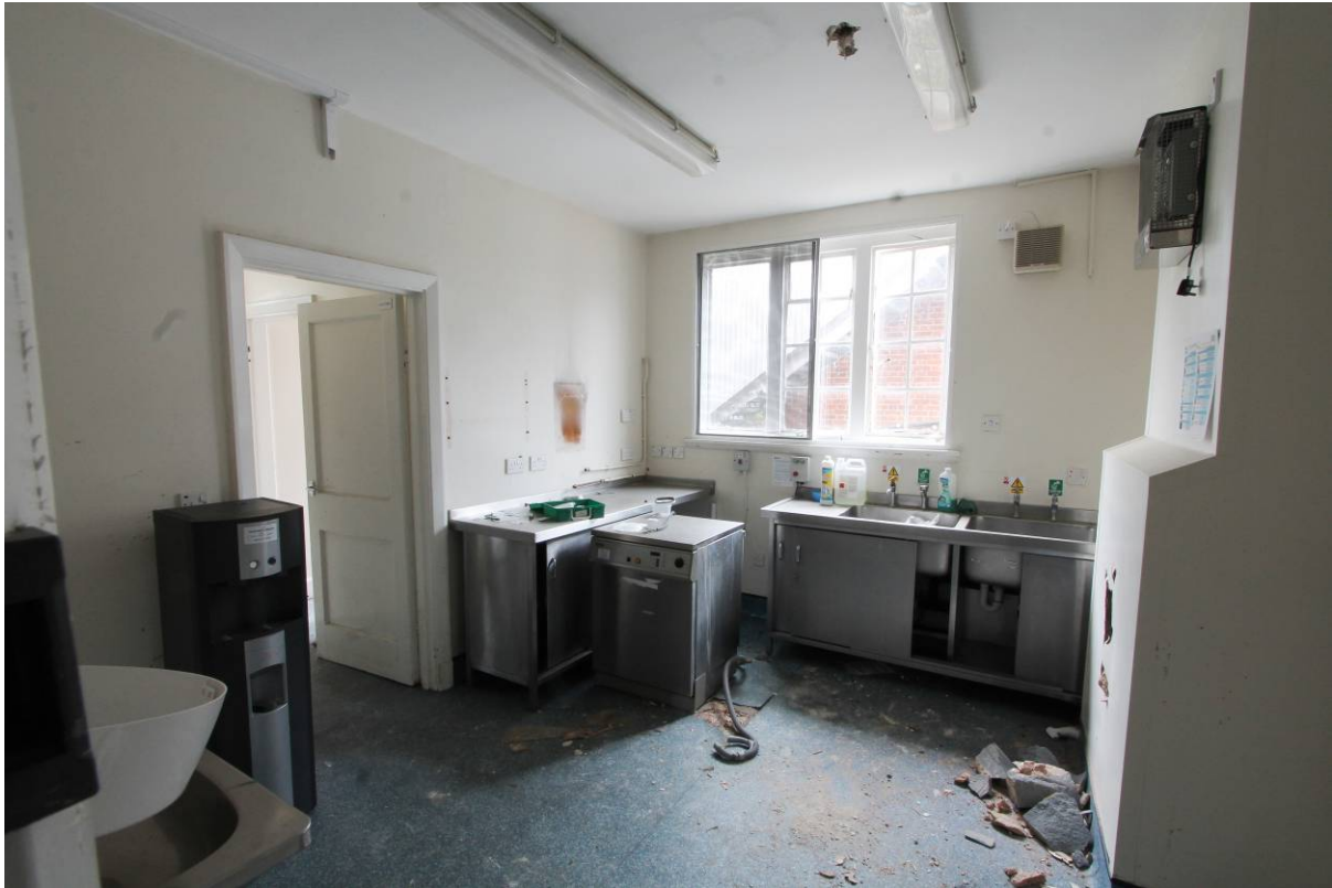
Plate 15 Western Villa, ground floor kitchen looking east
