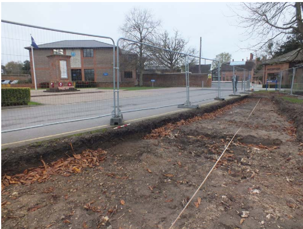
Plate 7: General shot of Access Road Trench at north-western extent, looking north-west (BRBS15 D1 (52))
