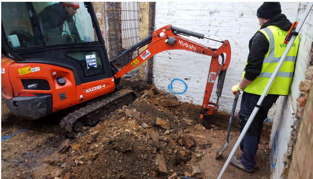
Plate 2: Excavation of foundation trench Area A
