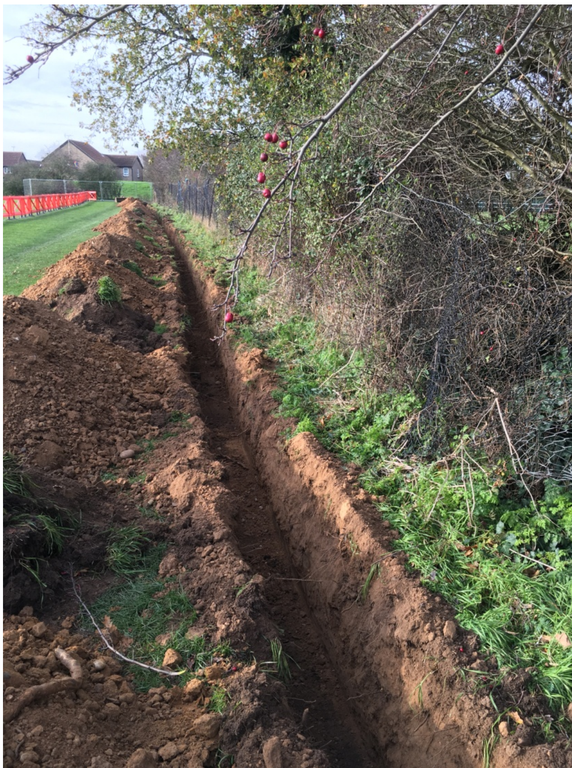
Plate 7: Trench 4 showing extent of trench cut for drainage pipe, view west
