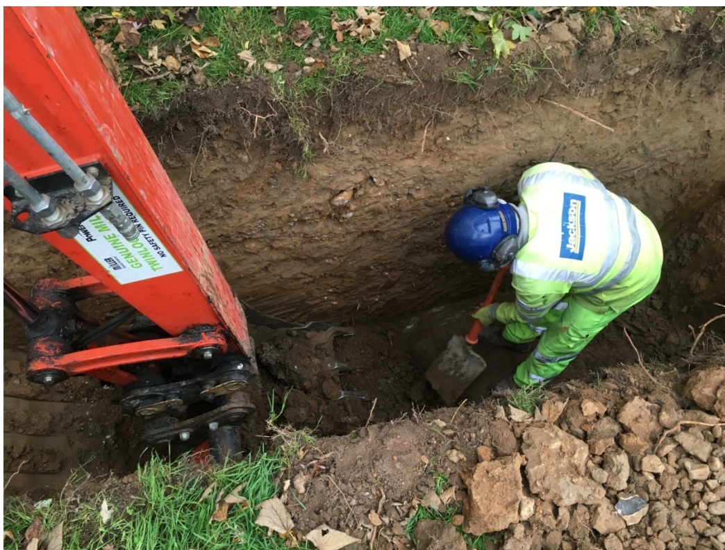
Plate 3: Excavation in Trench 1, locating surface water sewer pipe, view north
