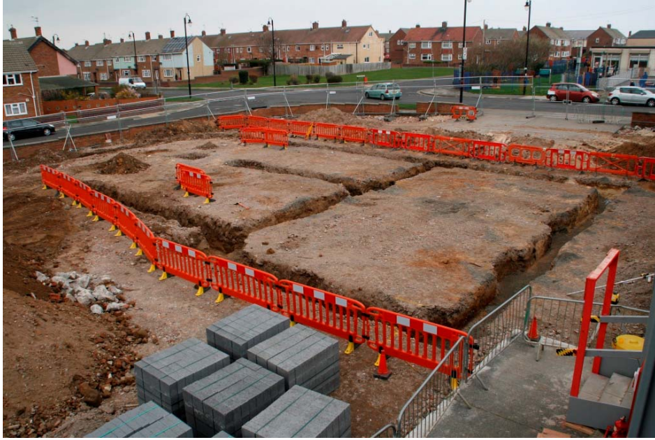
Plate 7. Area 4, general view of foundation trenches, looking north-west
