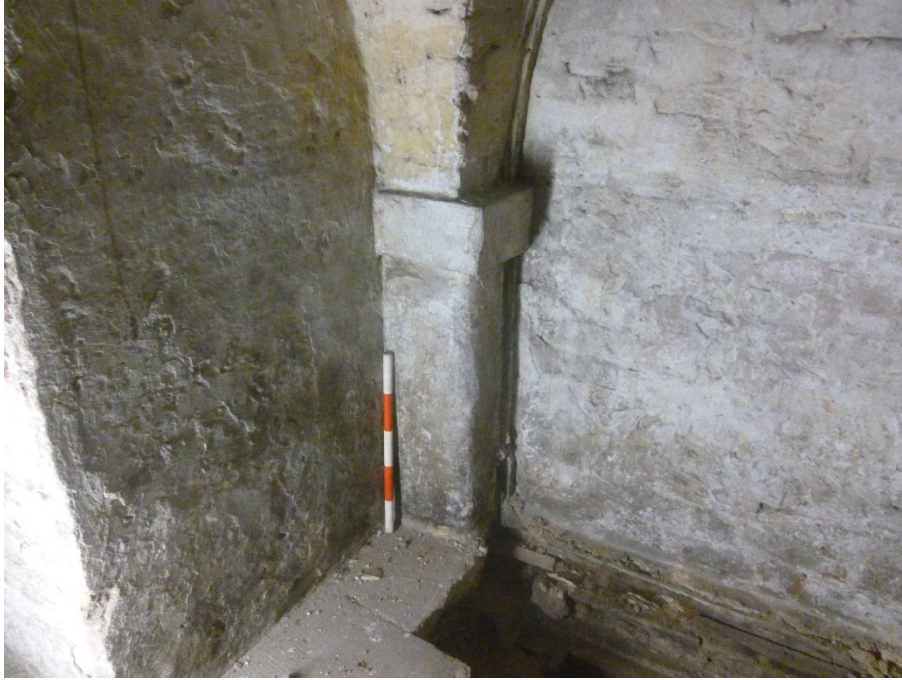
Plate 15: Test Pit H in the basement with corner column
