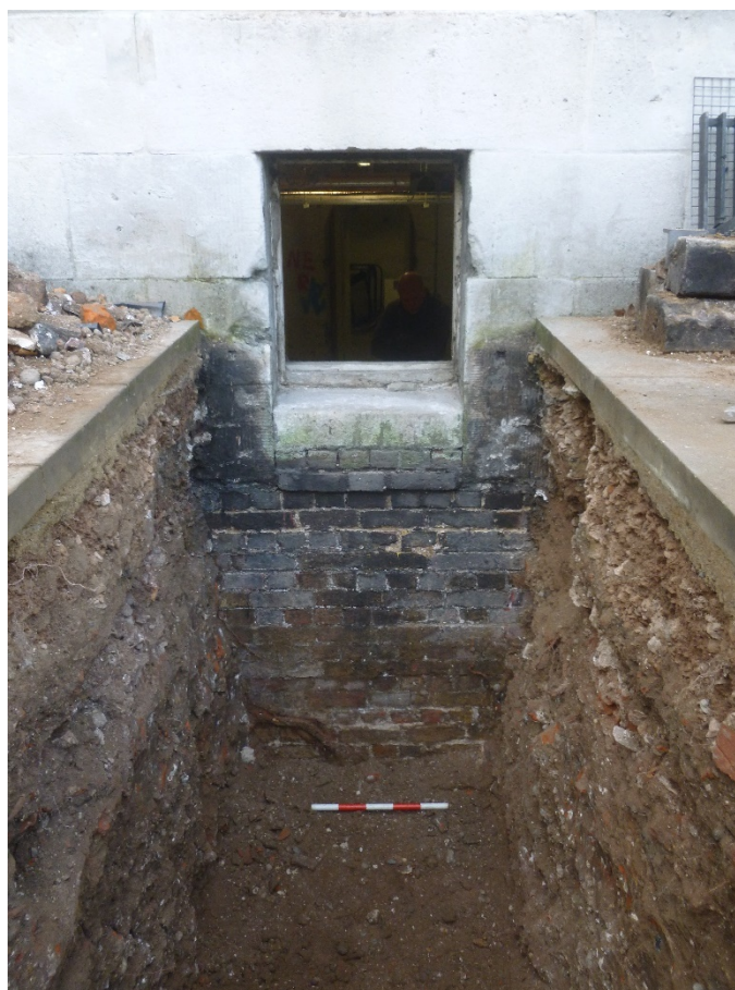
Plate 5: Trench 6, Window of the North Frontage excavated
