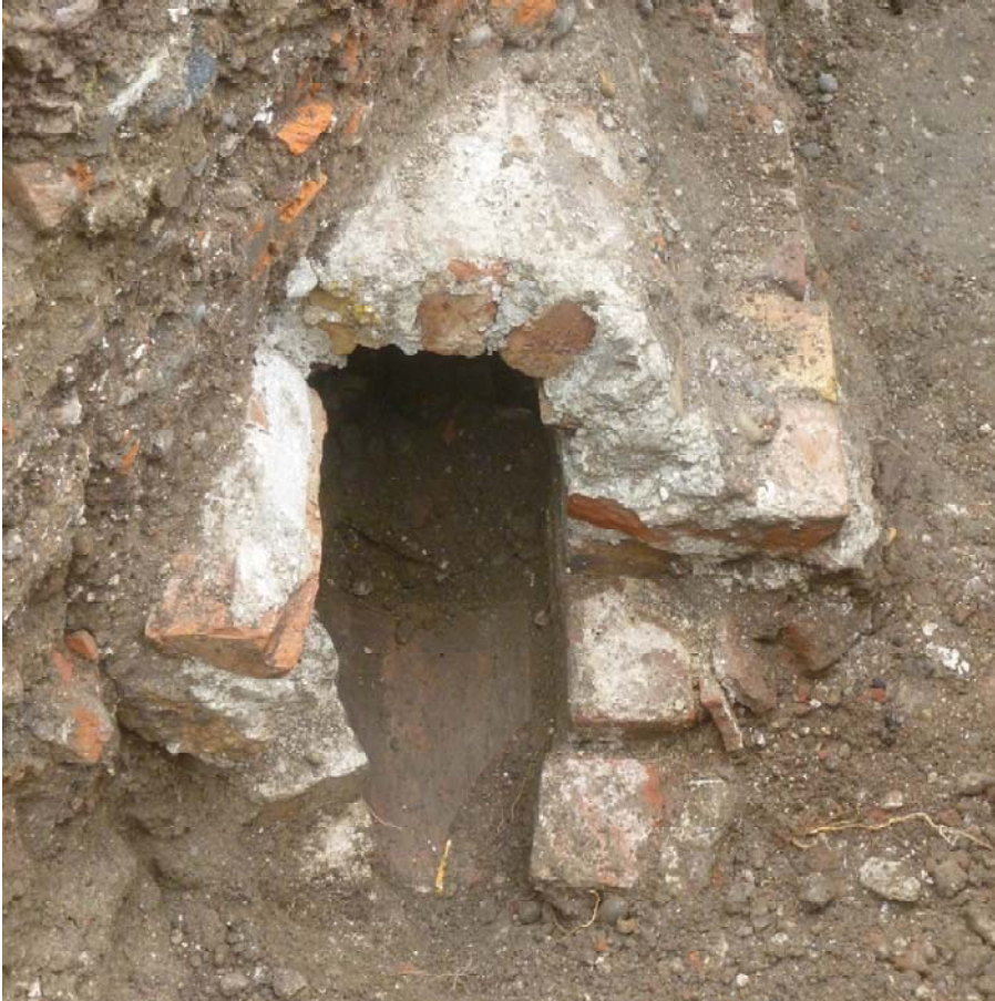
Plate 8: 18 th Century culvert [177] in Trench 9
