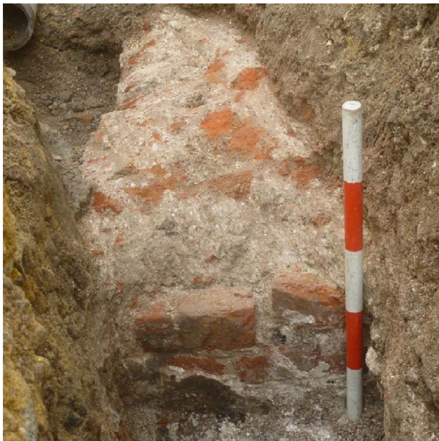
Plate 11: 17 th Century Wall Base [239] with adhering plaster
