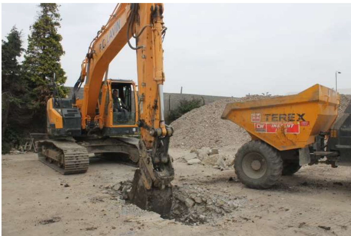
Plate 5 – Mechanical excavation of test pits (Test Pit 3; facing north)
