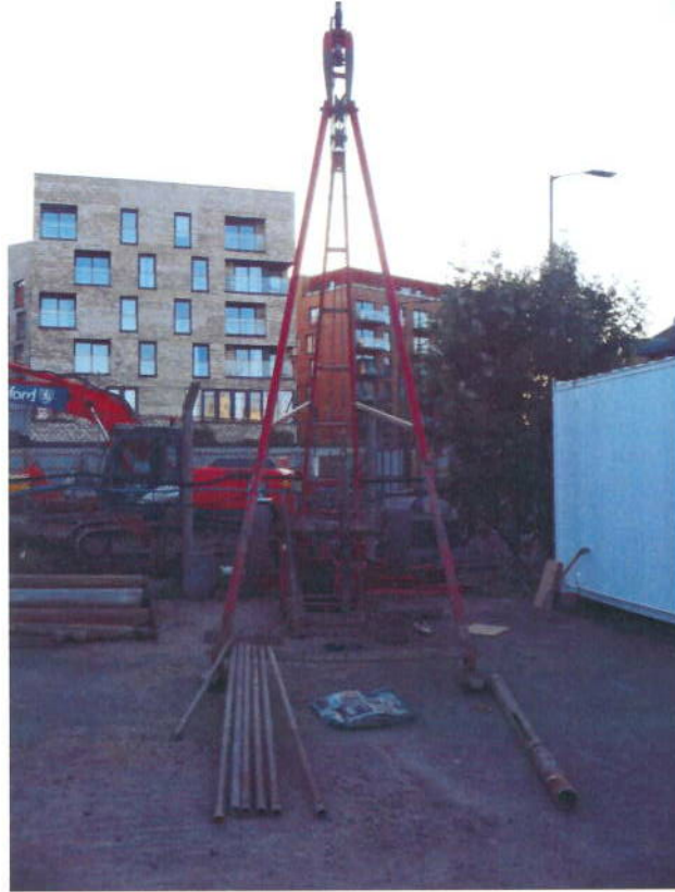
RIG SET UP AT BH1A
