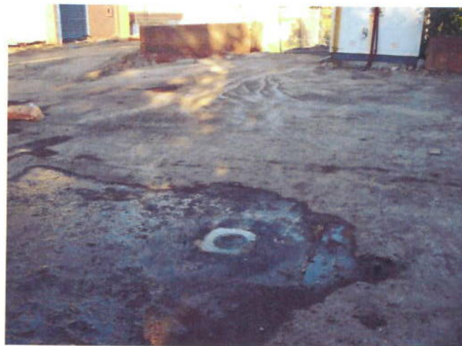
FLUSH HEADWORKS PROTECTING INSTALLATION
