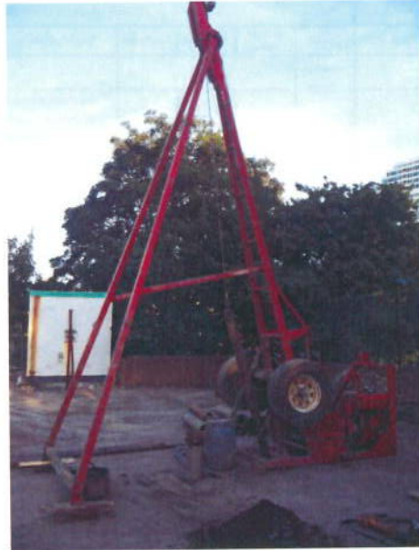
RIG SET UP AT BH3, HAZARDOUS CHEMICAL STORE IN BACKGROUND
