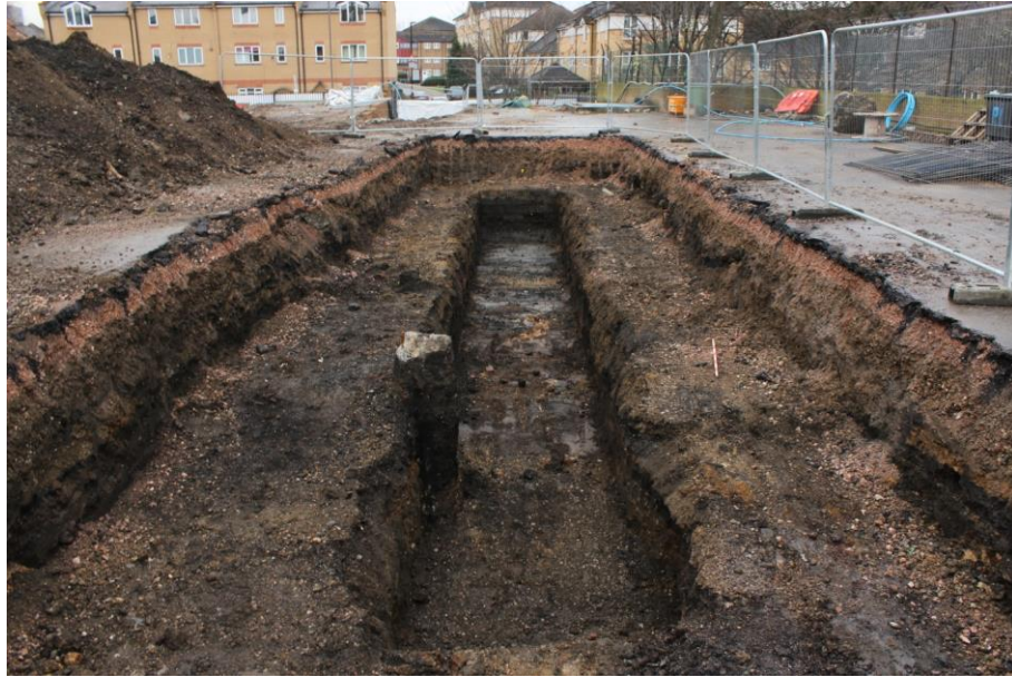
Plate 5: Trench 3 facing east, 1m scale
