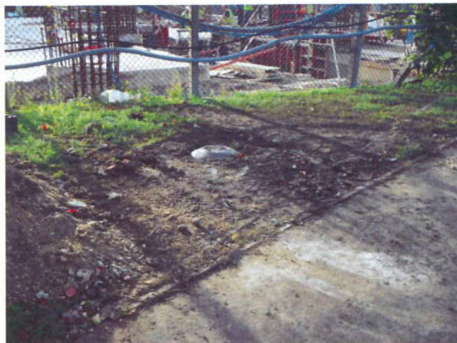
FLUSH HEADWORKS PROTECTING INSTALLATION
