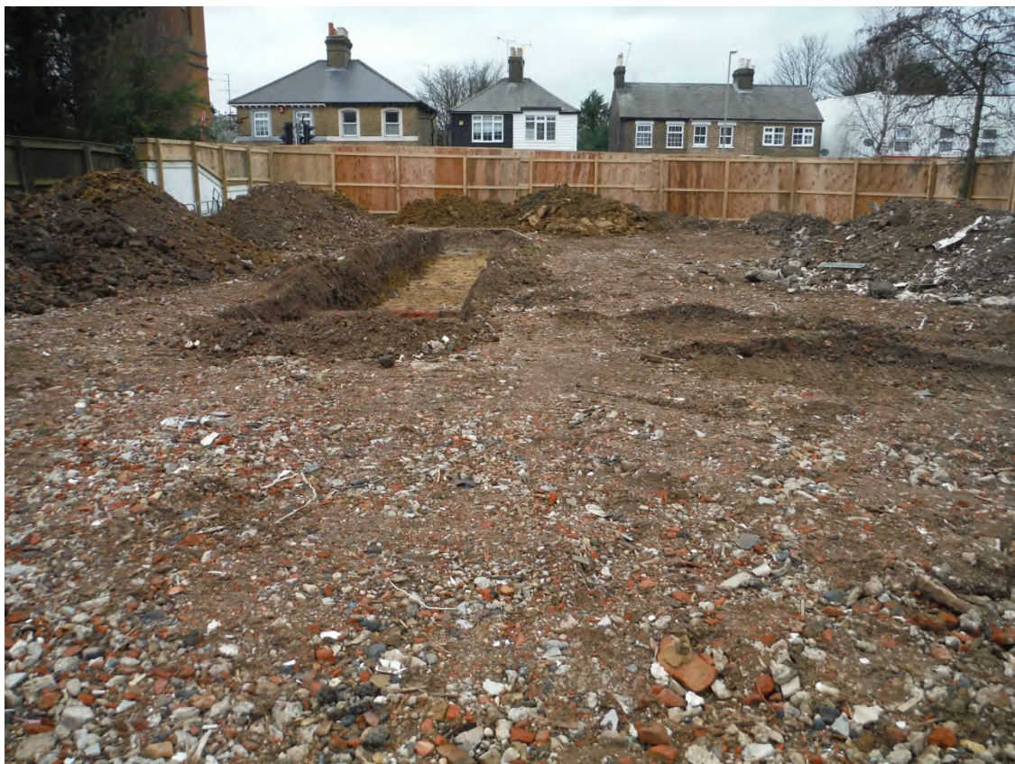
Plate 5: The site, view west
