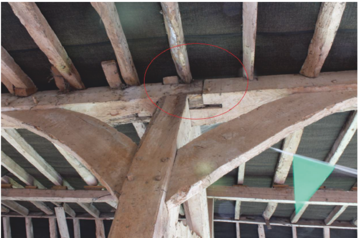
Plate 10 Face halved and counter bladed scarf and carpenters marks (highlighted) to arcade plate in Barn (A), looking west
