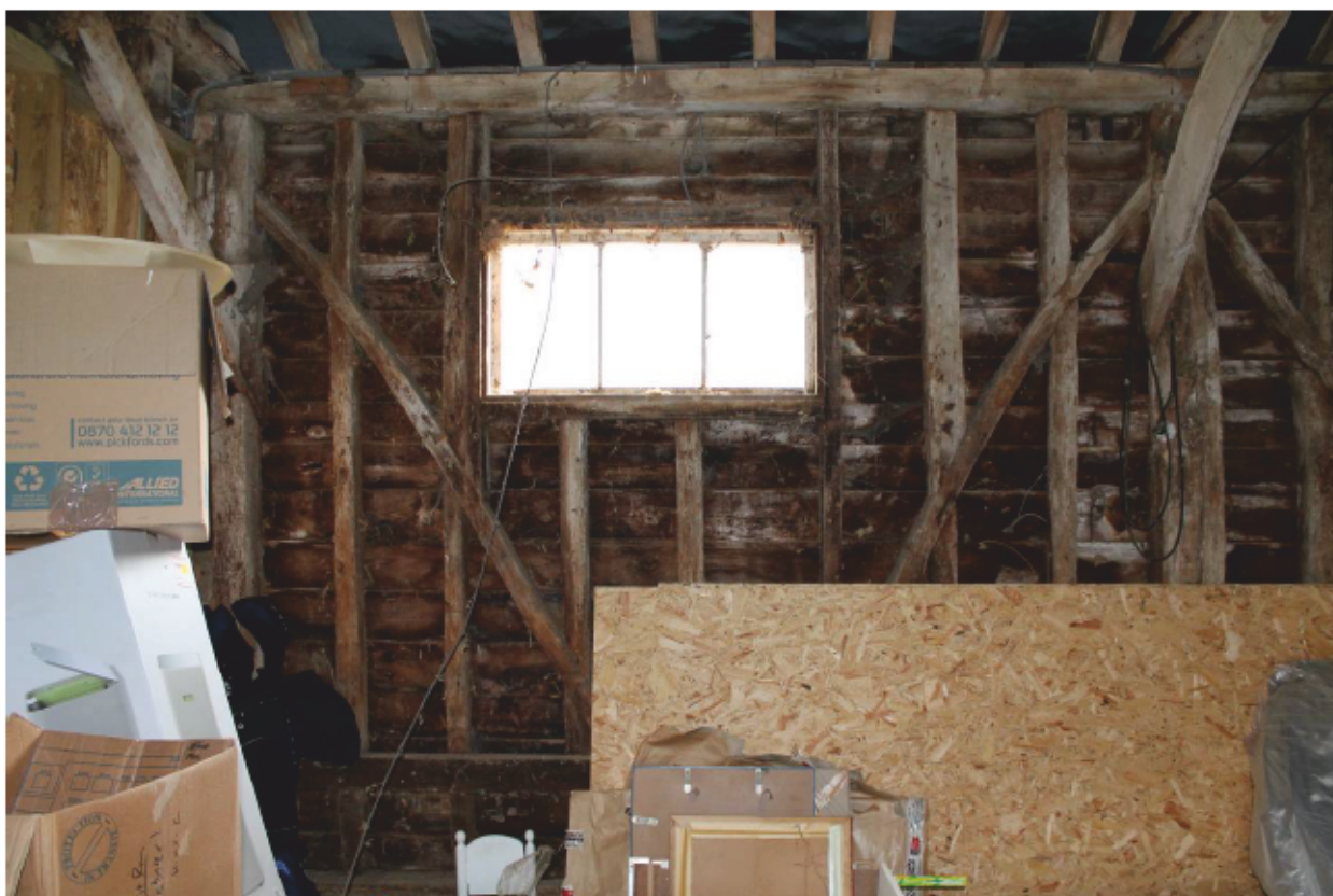
Plate 19 Primary braced wall framing in Cowshed (B), looking east
