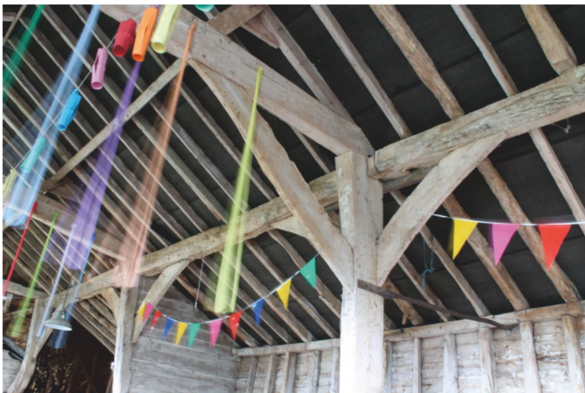
Plate 8 Jowled post and arched bracing to arcade in Barn (A), looking north-east
