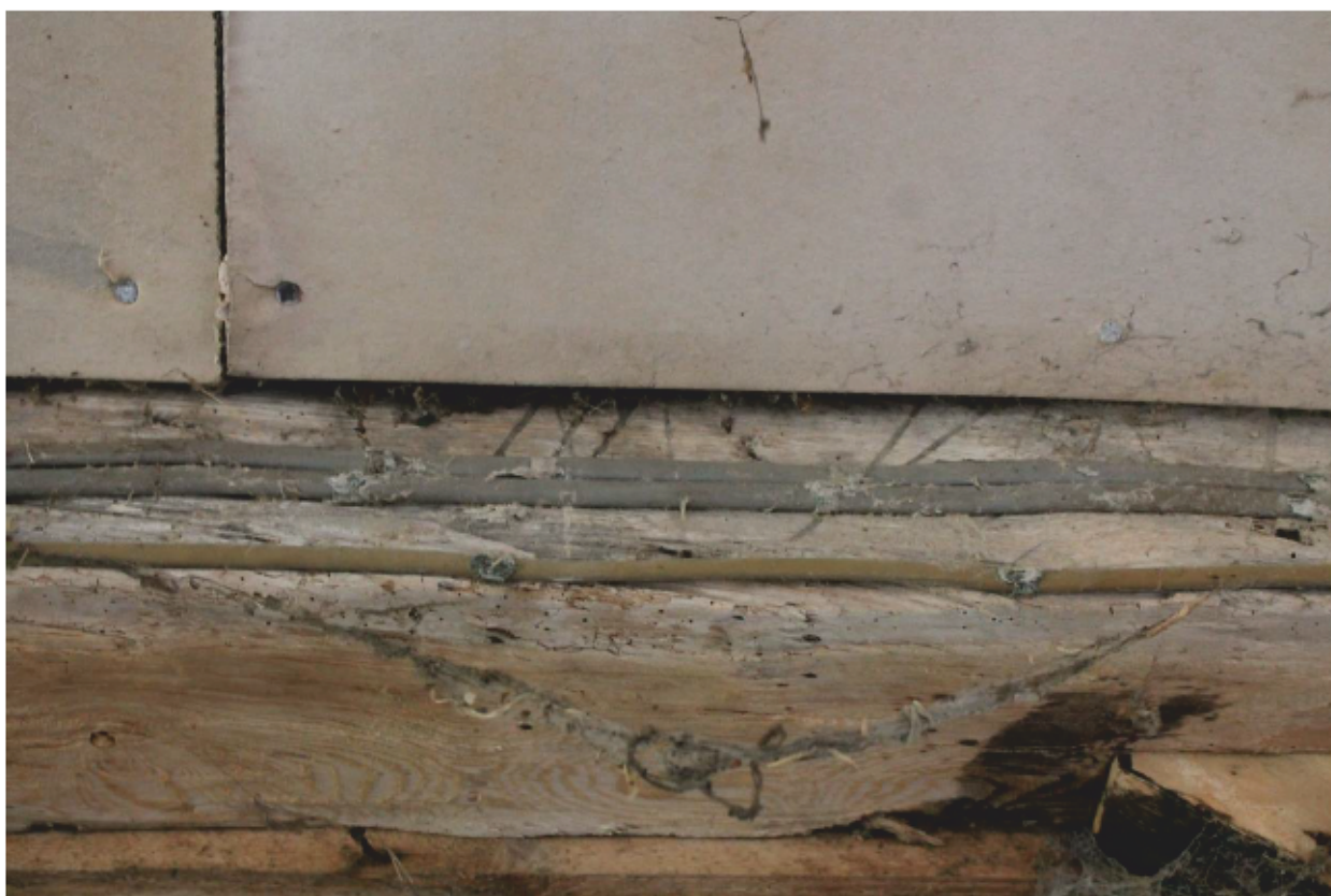
Plate 28 Baltic marks on arcade plate in Shelter shed (C), looking north
