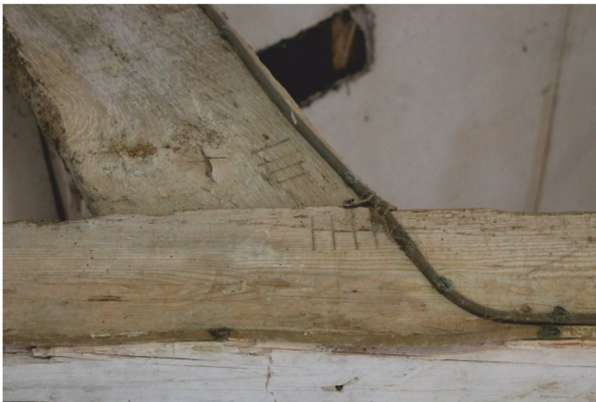
Plate 25 Carpenters marks (III) on tie-beam and raking strut in Shelter shed (C), looking east
