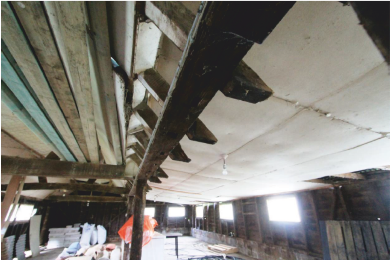
Plate 35 Empty mortices to plate soffit in Shed (D), looking south-west
