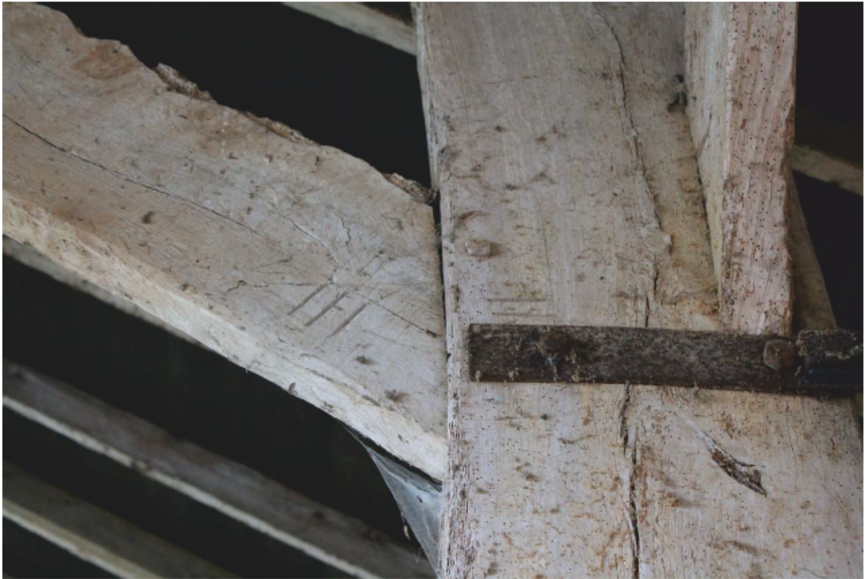
Plate 9 Carpenters assembly marks (III) on post and brace (Bay 2-3) in Barn (A), looking north
