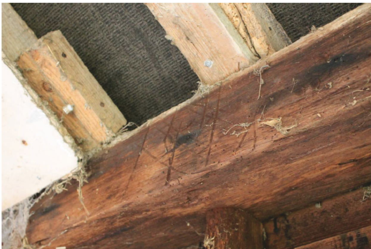
Plate 27 Baltic marks on wall plate in Shelter shed (C), looking south-east
