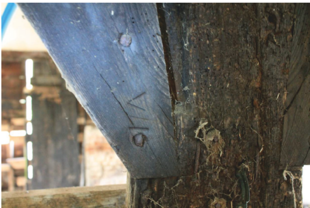
Plate 24 Roman marking (VII) to arch brace in Shelter shed (C), looking south
