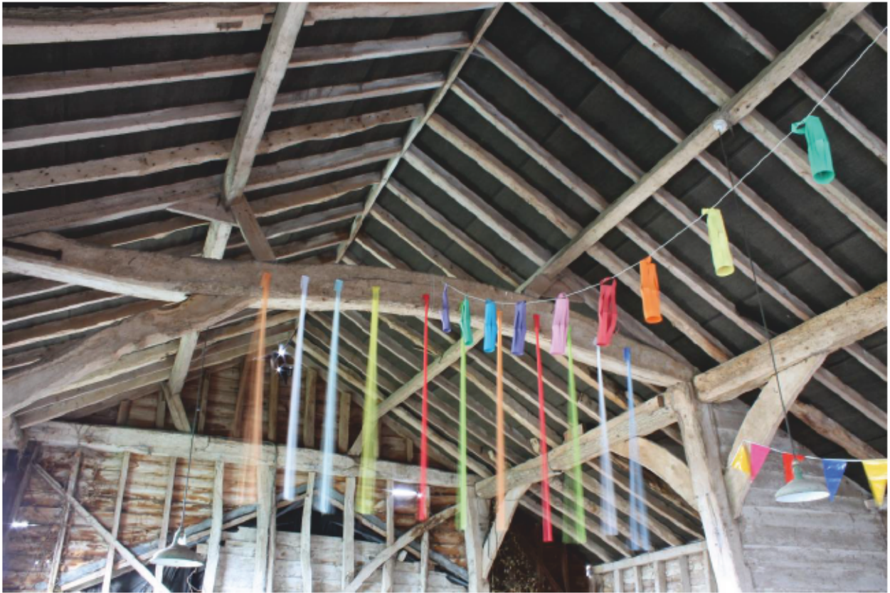
Plate 15 Simple replacement roof structure and common rafters in Barn (A), looking north
