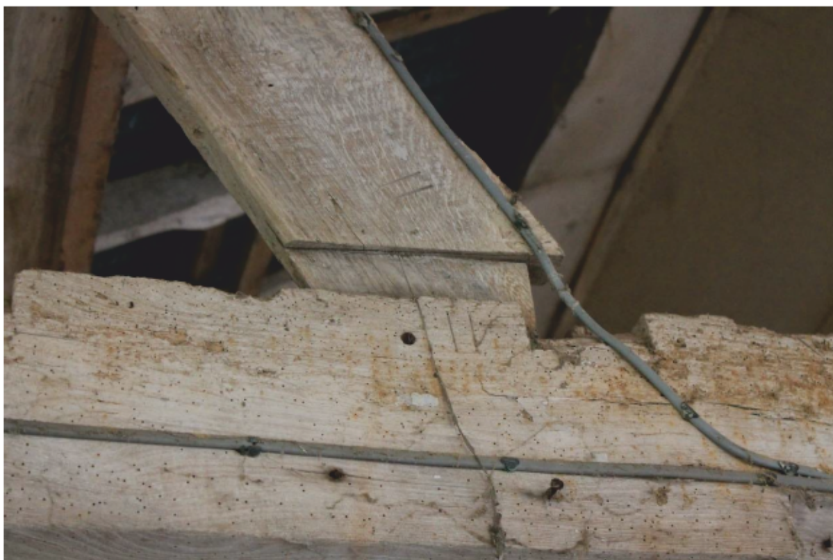
Plate 26 Carpenters marks (II) on tie-beam and raking strut in Shelter shed (C), looking east
