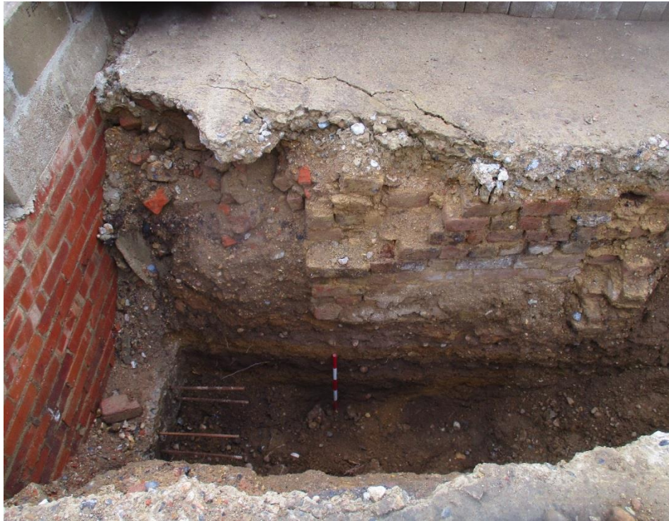
Plate 3: Section 3, section of 19 th century brick wall to right (view to south east) Scale 0.5m
