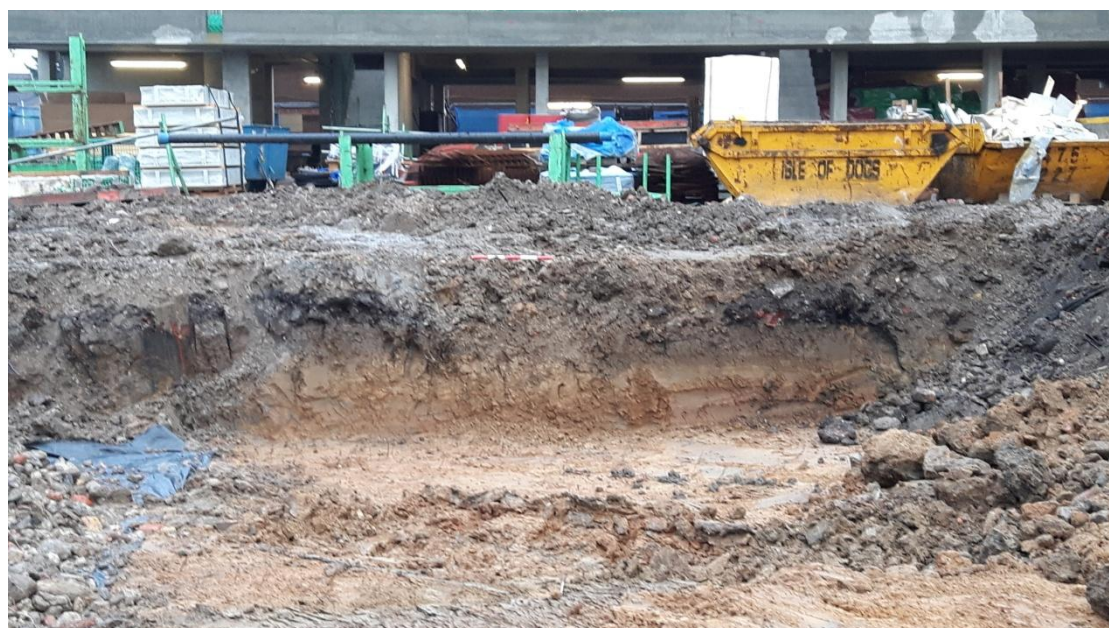
Plate 4 - South facing section of Trench 4. This also shows the large amount of modern made ground on top of the natural alluvium.
