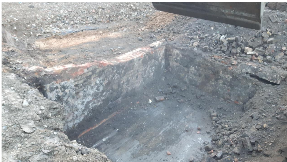
Plate 7 – Southeast facing shot of modern basement [133]
