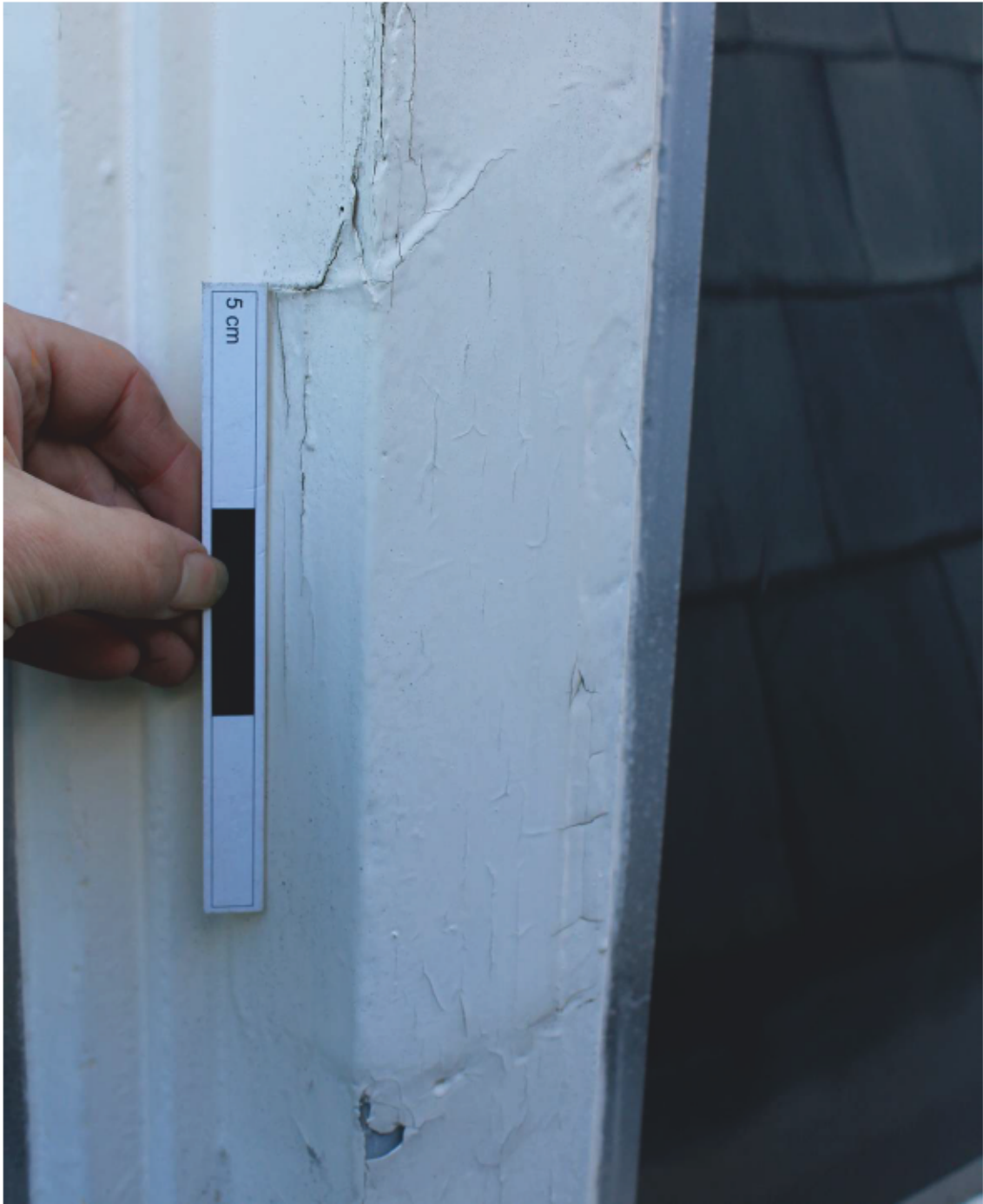
Plate 35 Lantern B: External Repair 18
