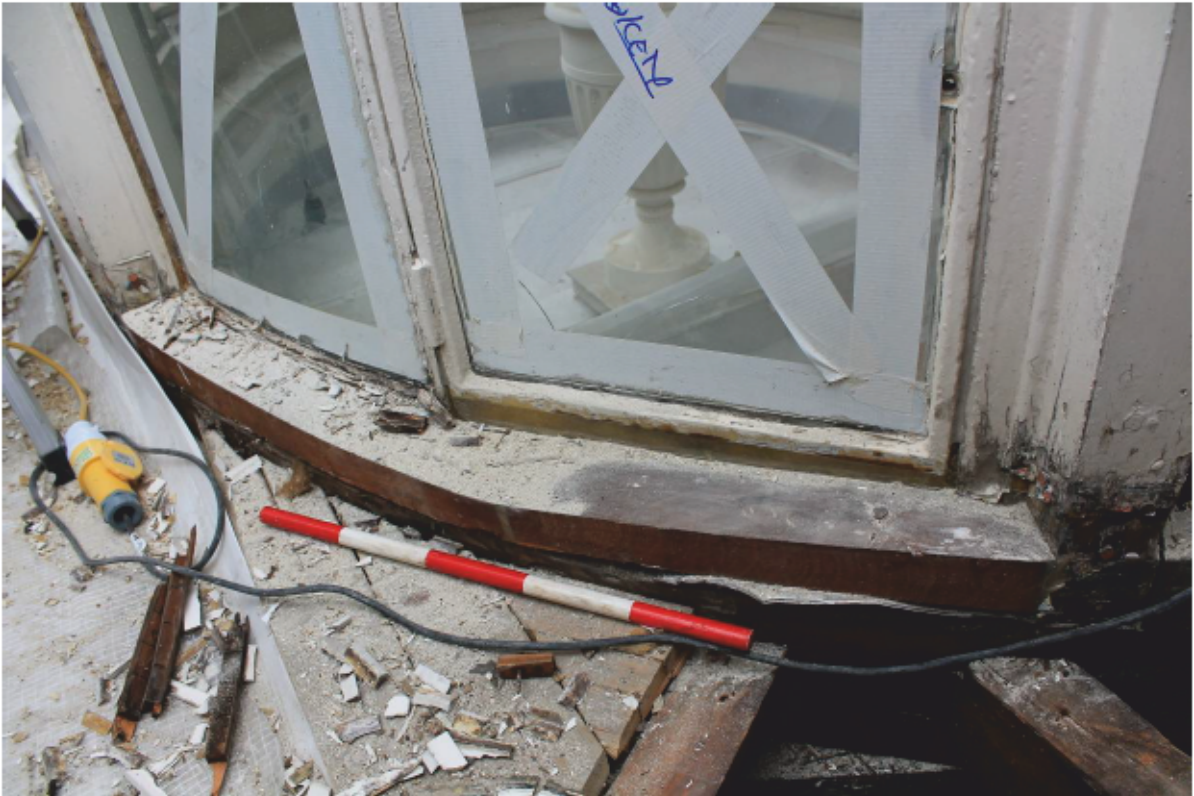
Plate 76 Lantern A: Modern heightening to sill
