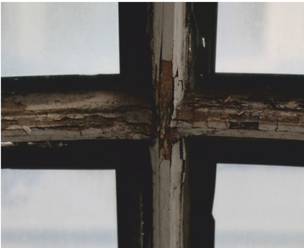
Plate 47 Lantern B: Internal Repair 7
