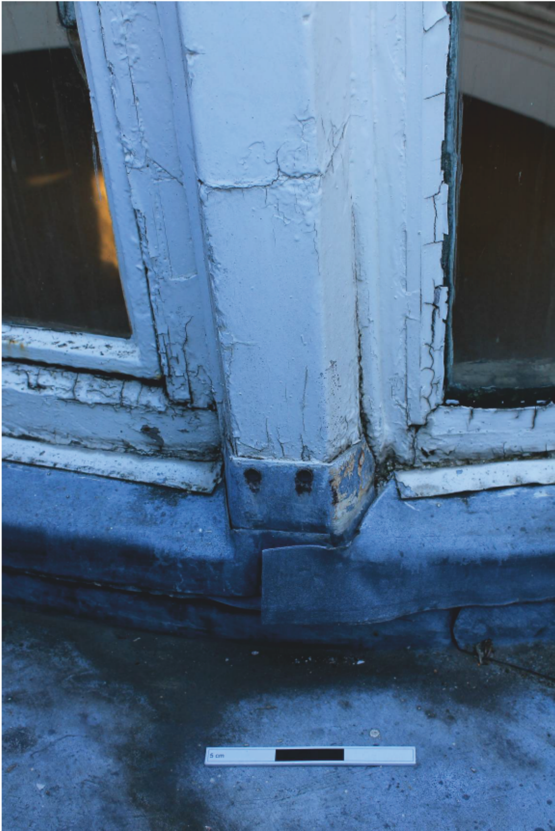
Plate 54 Lantern C: External Repair 28
