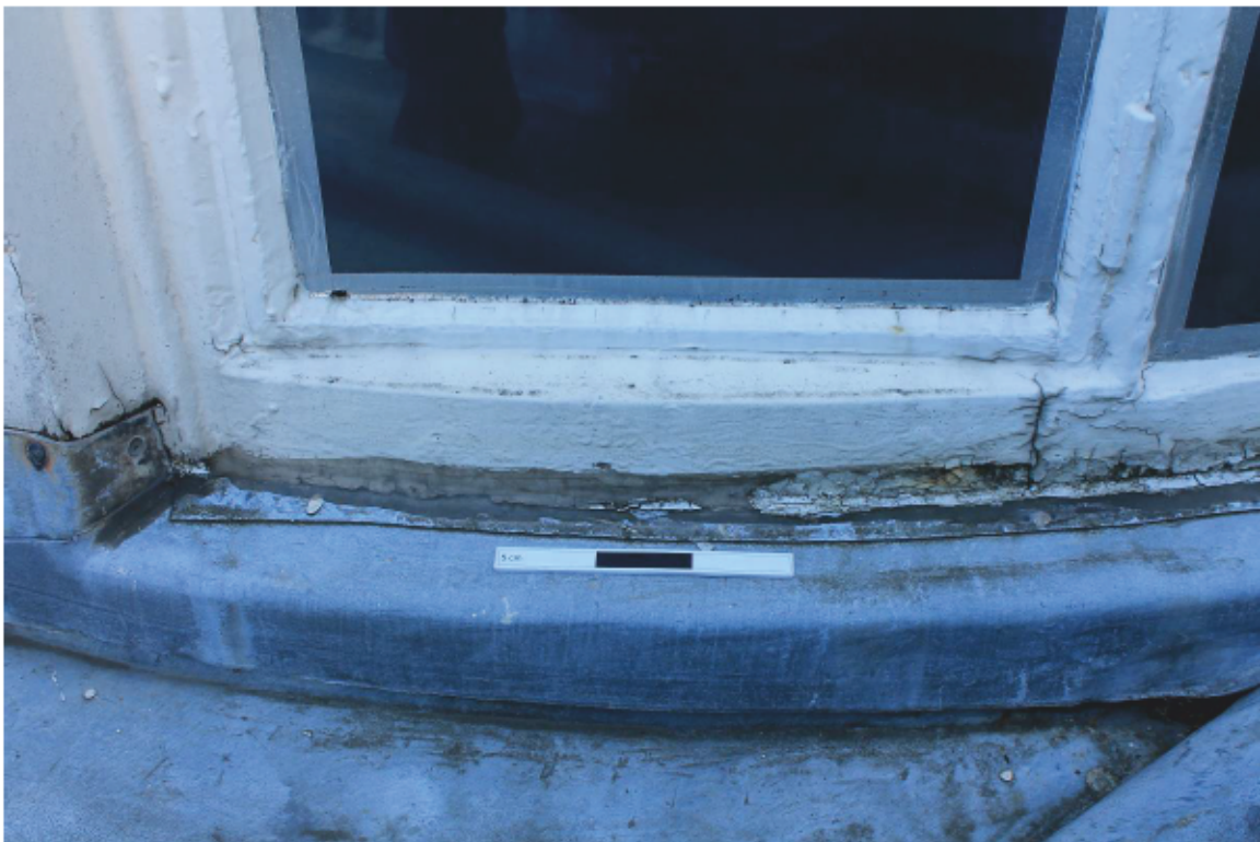
Plate 37 Lantern B: External Repair 20
