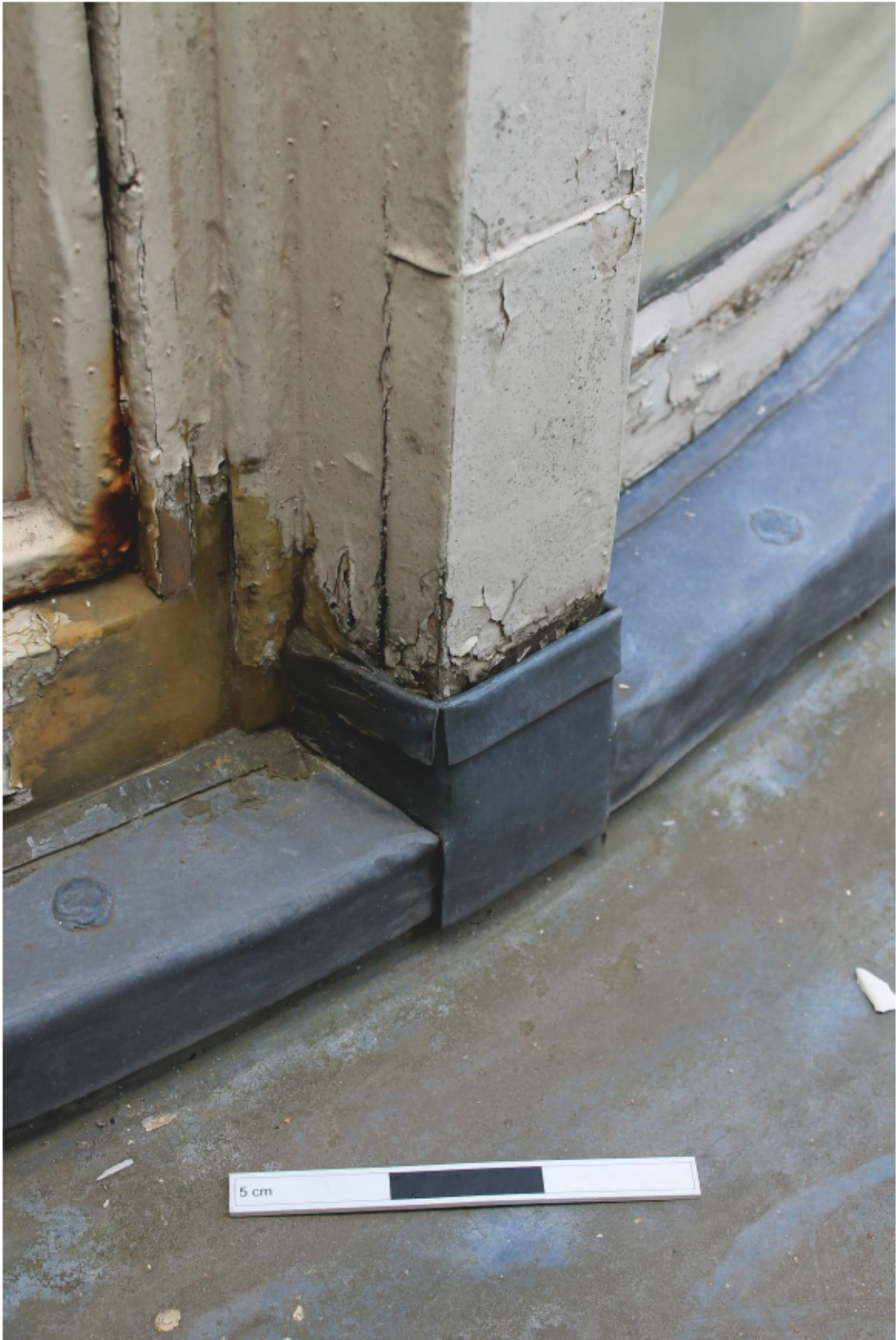
Plate 17 Lantern A: External Repair 14
