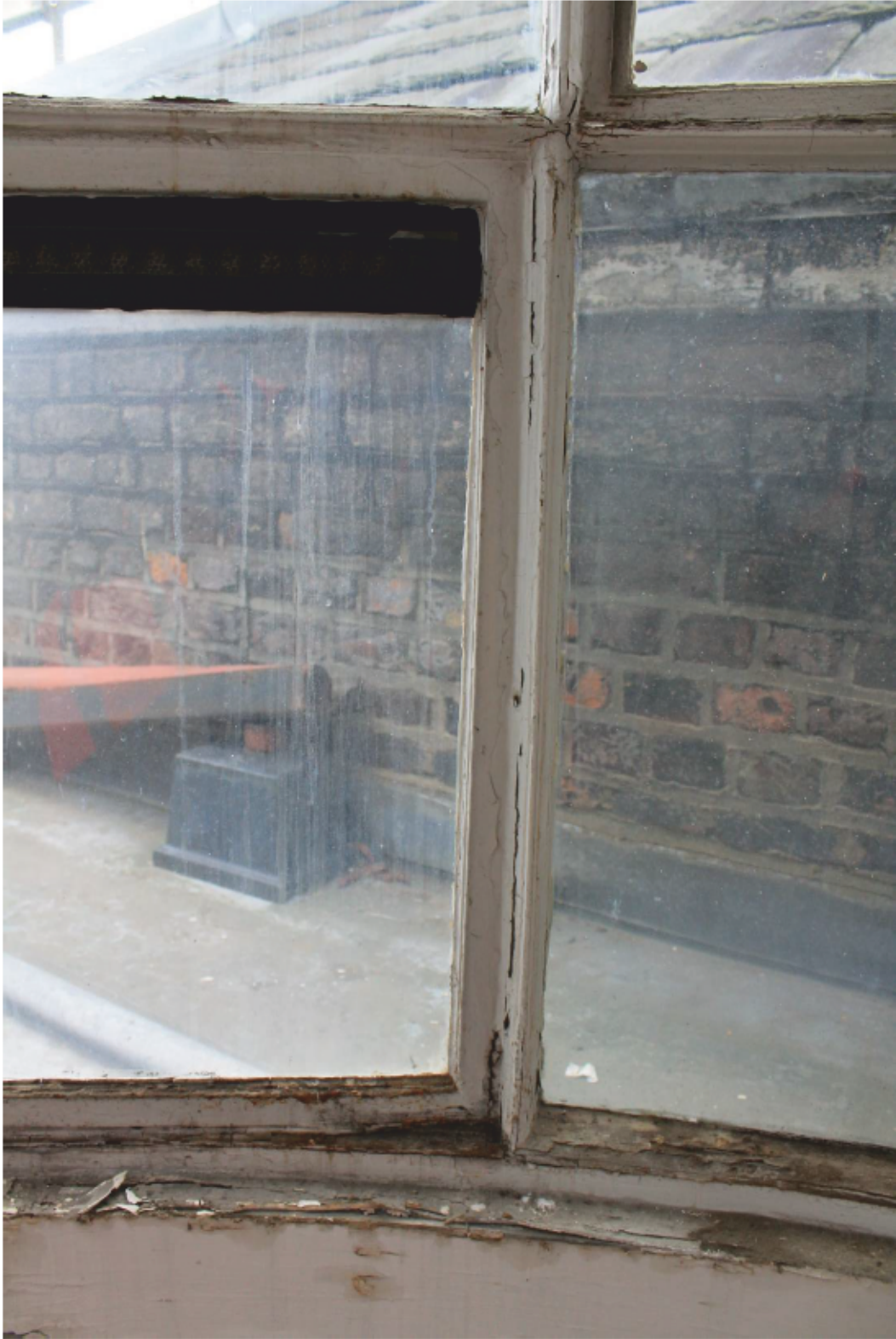
Plate 65 Lantern C: Internal Repair 13
