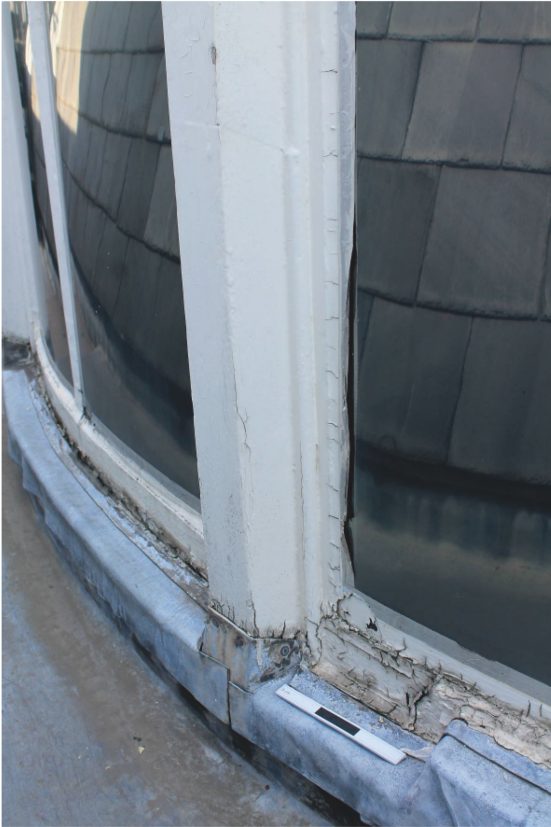
Plate 34 Lantern B: External Repair 17
