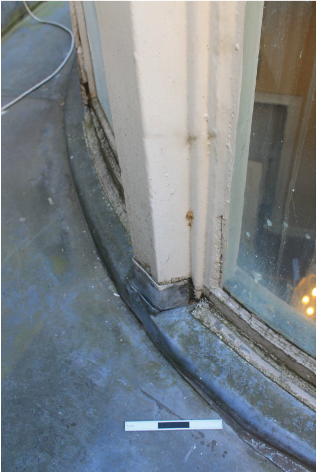
Plate 55 Lantern C: External Repair 29
