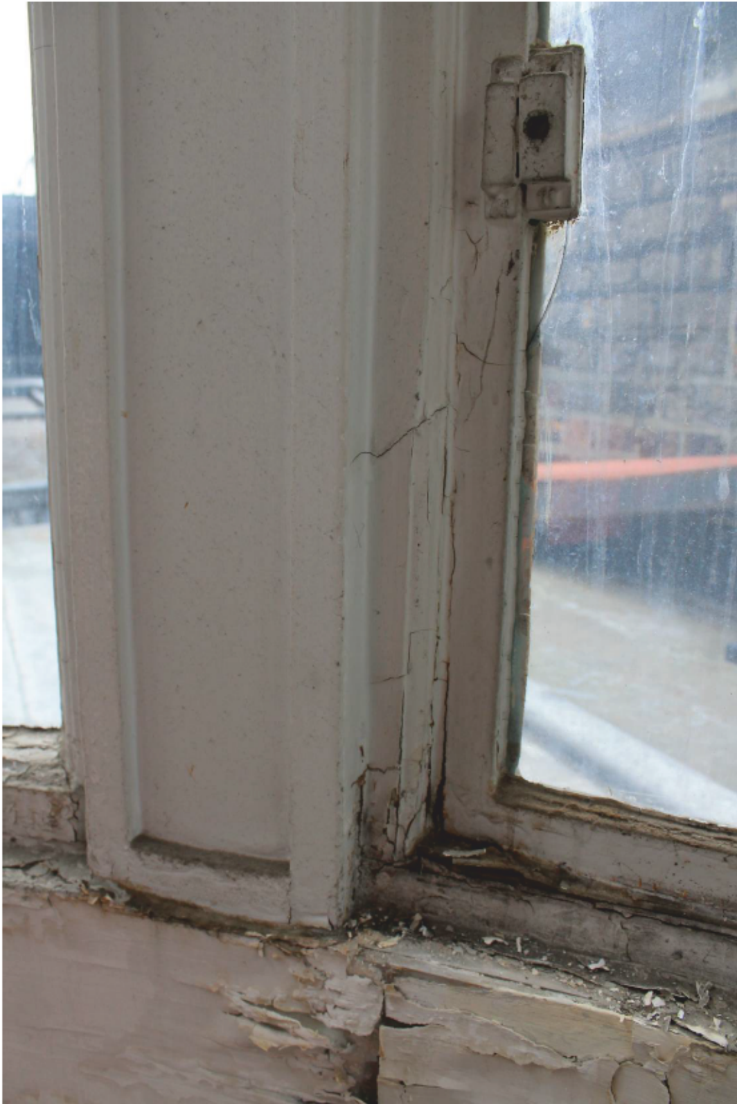
Plate 69 Lantern C: Internal Repair 17
