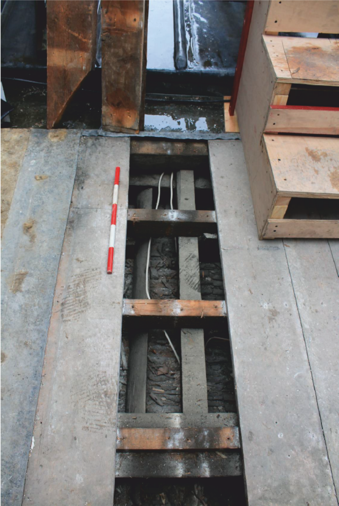
Plate 80 Lantern C: Opening C2 looking west
