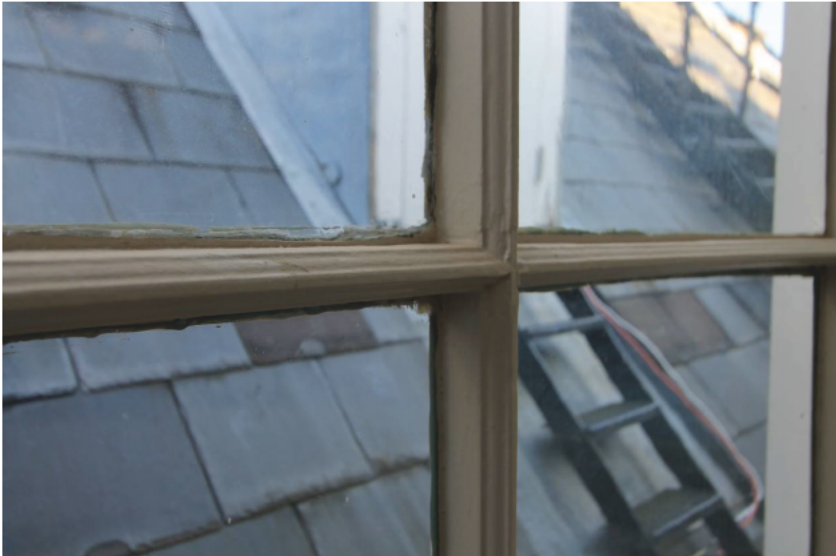
Plate 22 Detail of typical glazing bar
