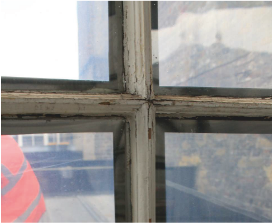
Plate 48 Lantern B: Internal Repair 8
