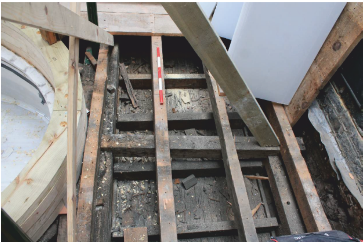
Plate 100 Lantern C: Sub-structure looking north
