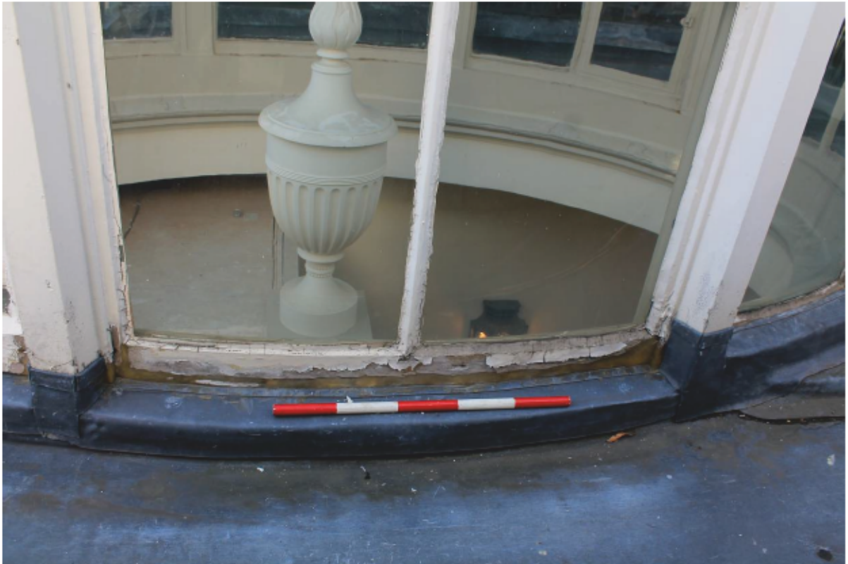
Plate 9 Lantern A: External Repair 6
