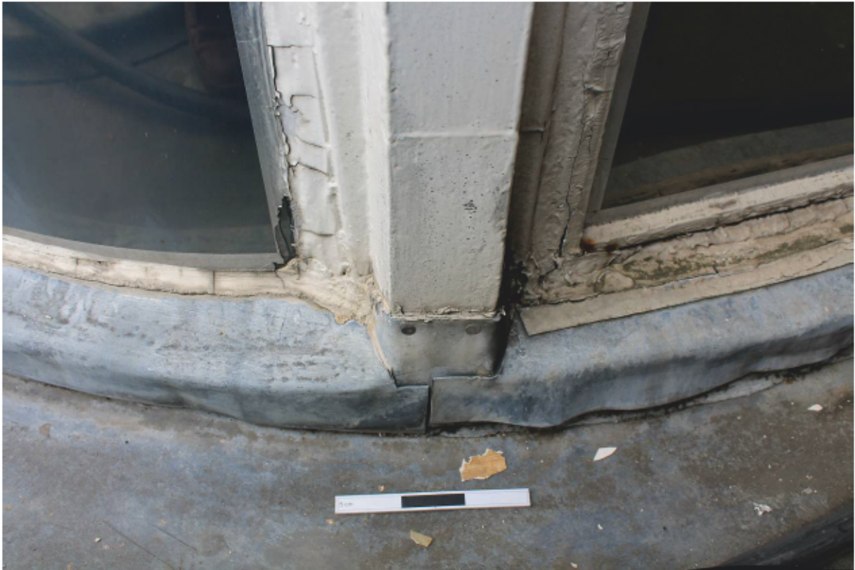
Plate 32 Lantern B: External Repair 15
