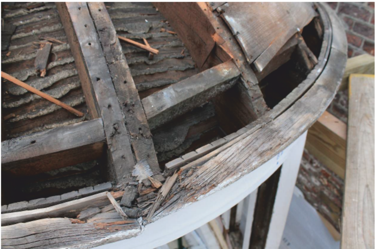
Plate 86 Lantern B: Detail of rafters and eaves
