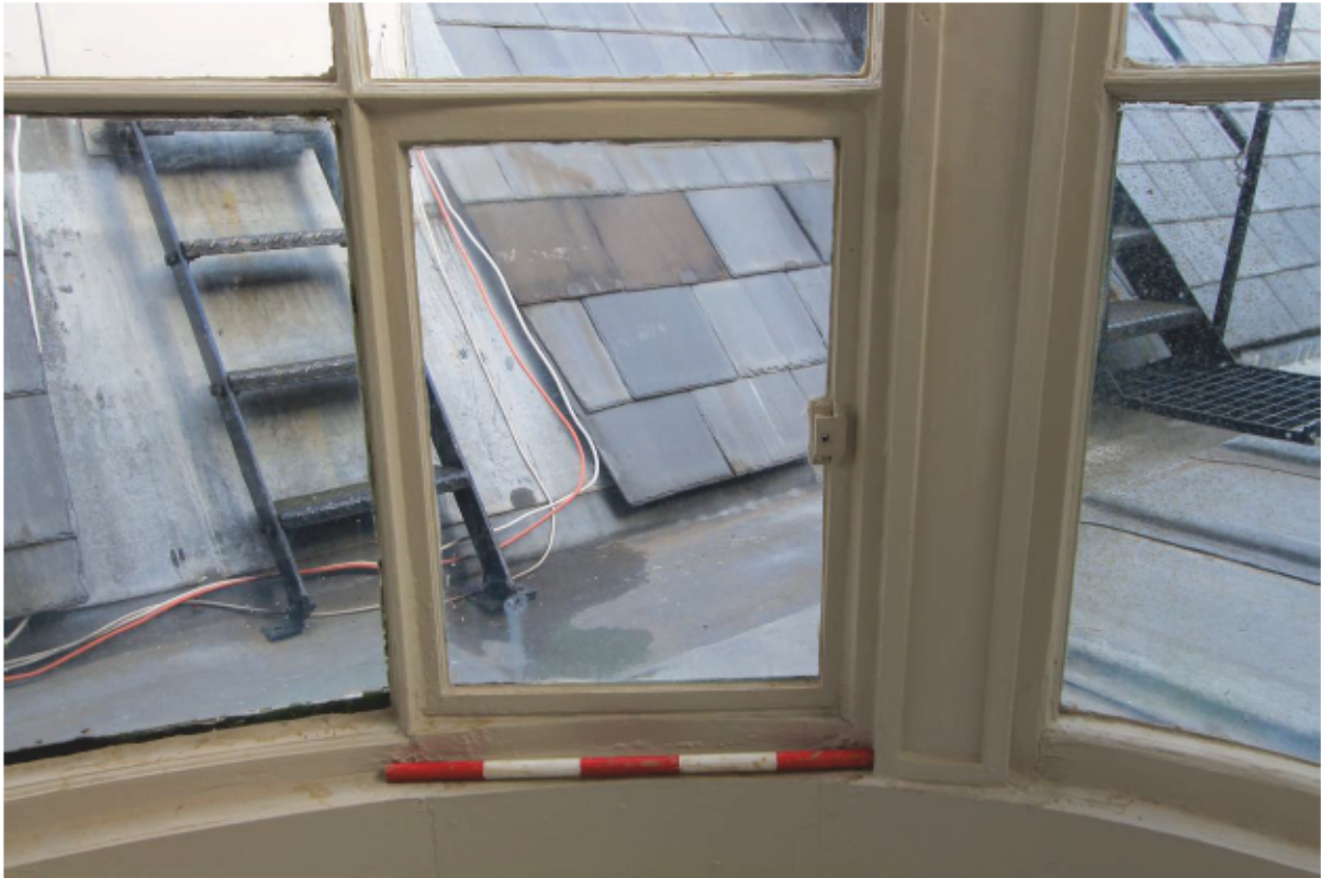
Plate 26 Lantern A: Internal Repair 4
