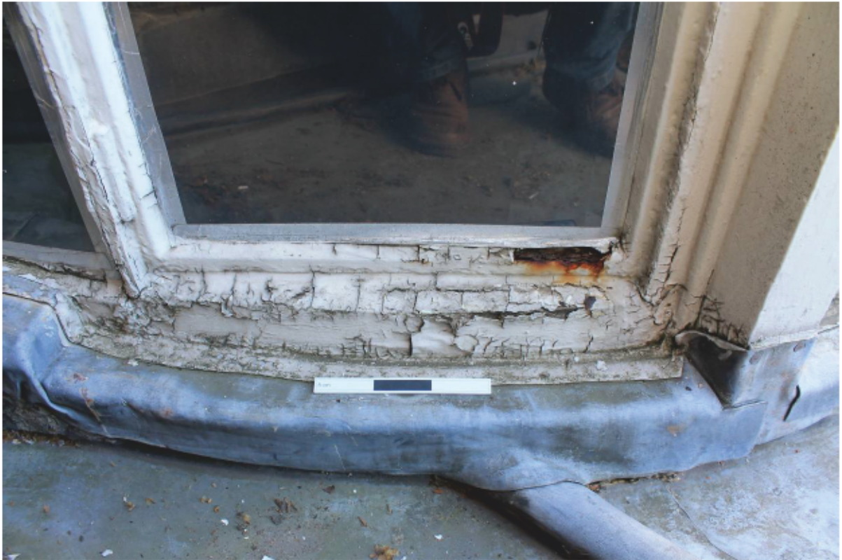
Plate 40 Lantern B: External Repair 23
