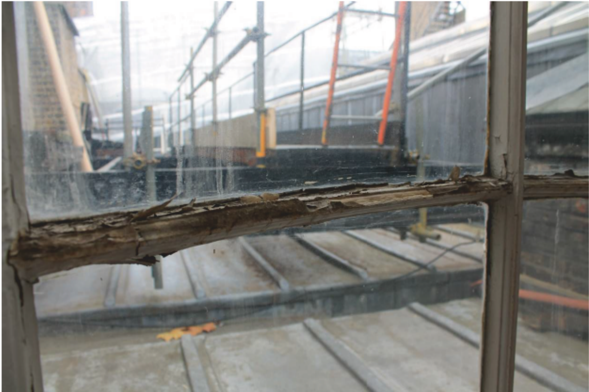
Plate 71 Lantern C: Internal Repair 19
