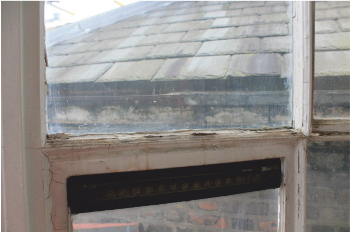
Plate 66 Lantern C: Internal Repair 14
