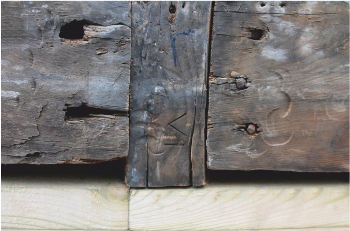
Plate 103 Lantern A: Roman marking to mullion foot
