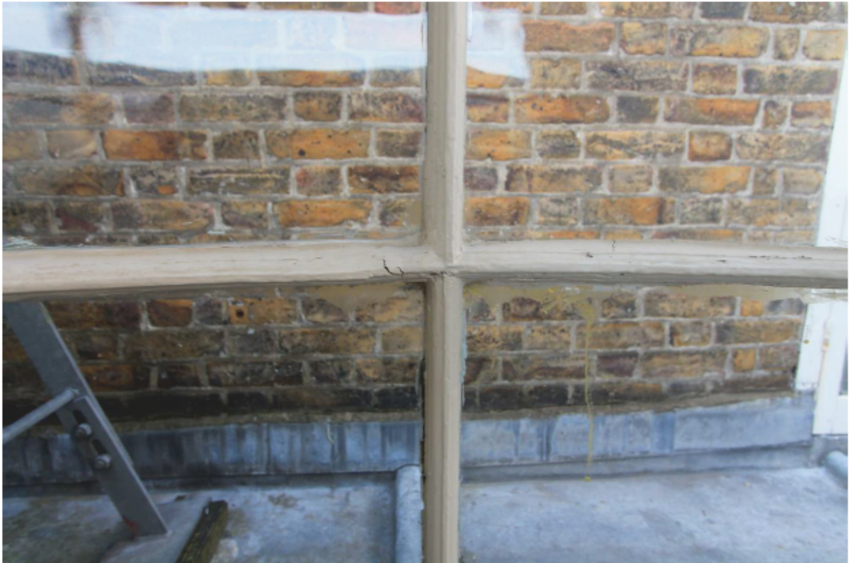
Plate 24 Lantern A: Internal Repair 2
