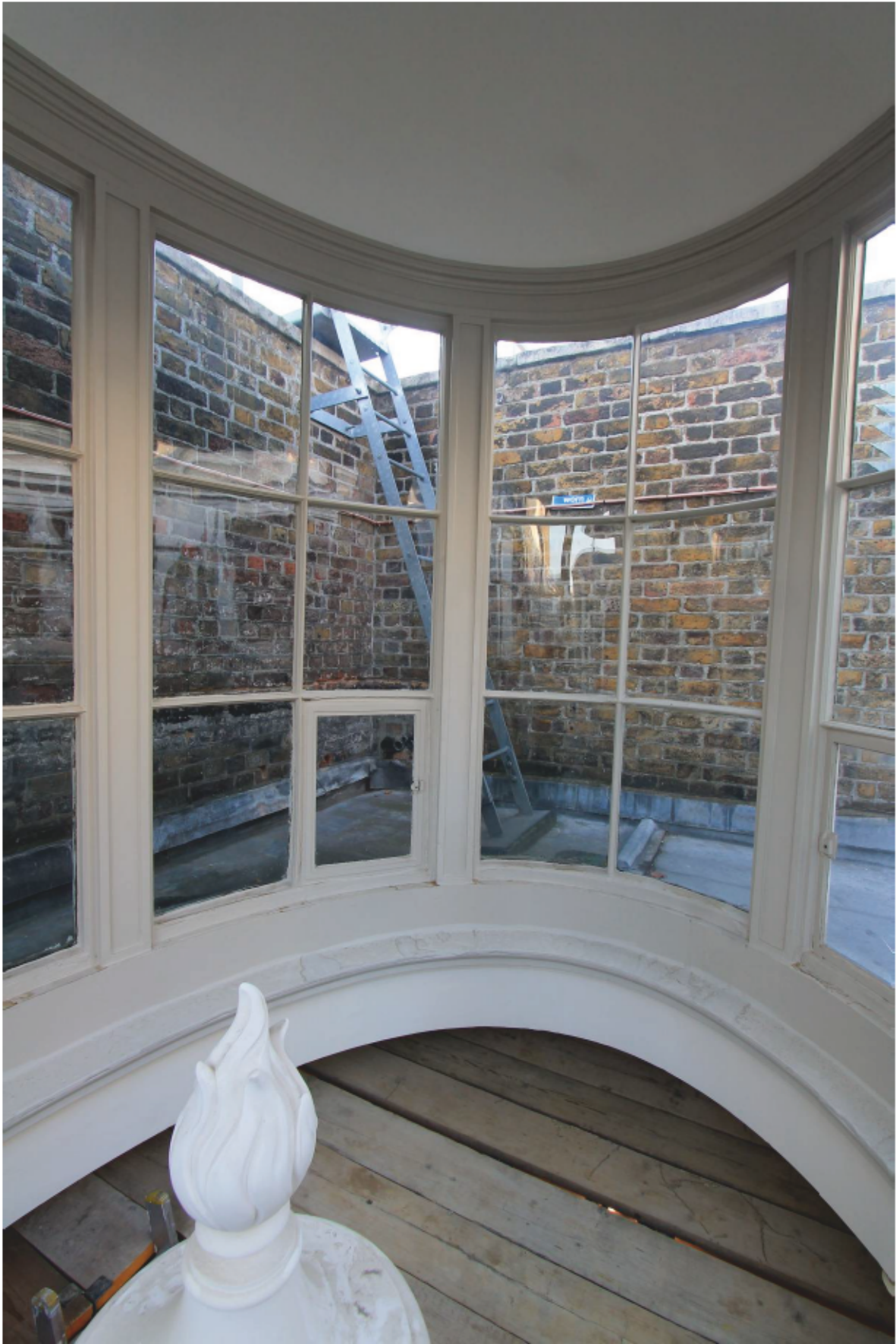
Plate 18 Lantern A: Internal looking south-west
