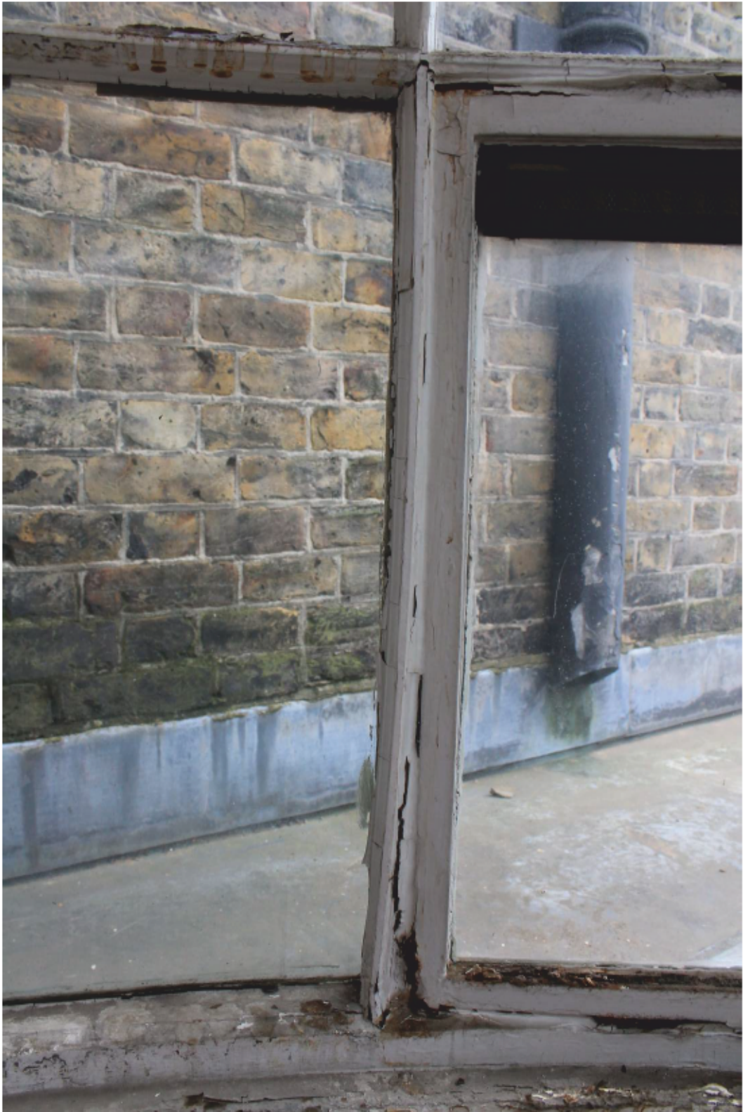
Plate 64 Lantern C: Internal Repair 12
