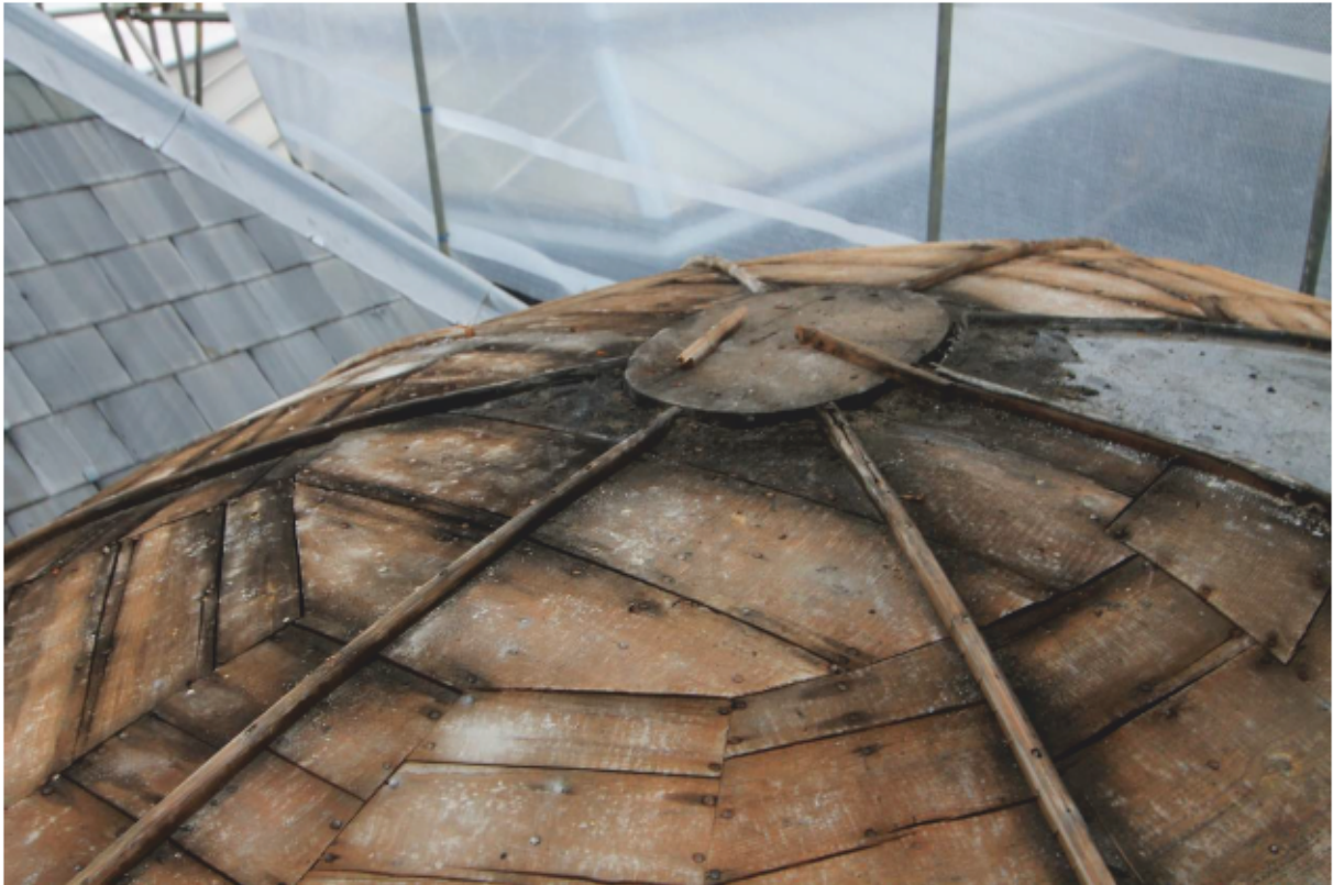
Plate 85 Lantern B: Detail of sarking boards and central boss for leadwork
