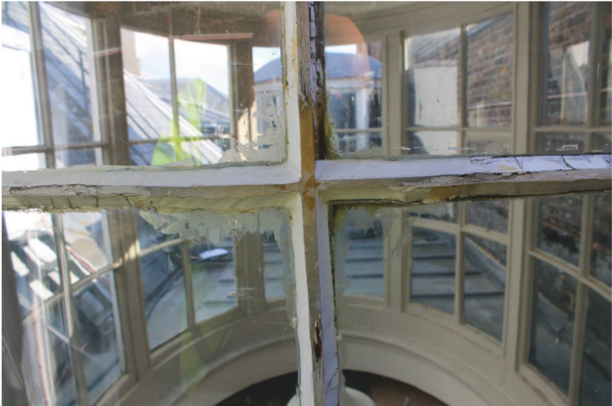
Plate 12 Lantern A: External Repair 9
