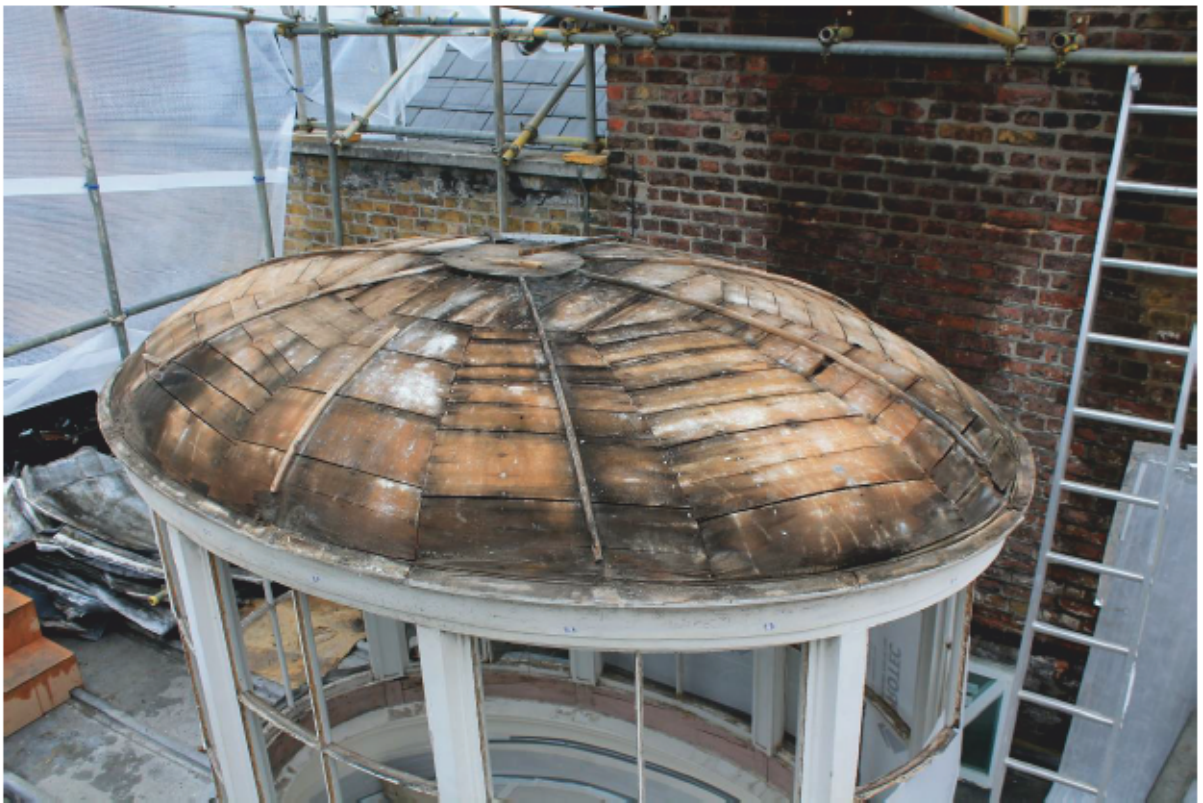
Plate 84 Lantern B: Following removal of lead flashings, looking south-east
