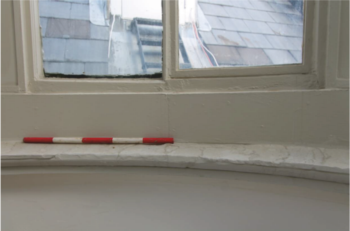
Plate 28 Lantern A: Internal Repair 6 and 6A
