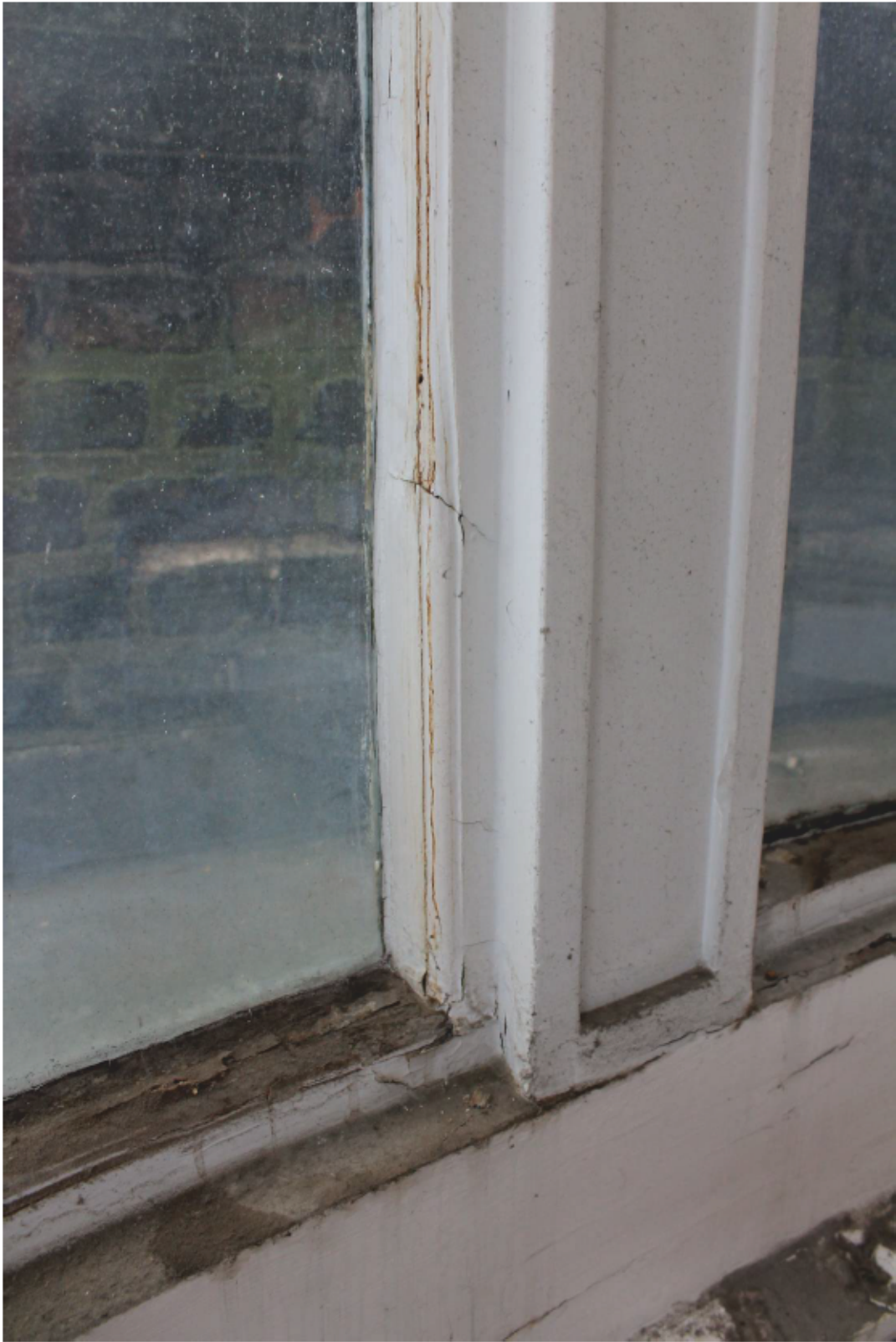
Plate 70 Lantern C: Internal Repair 18
