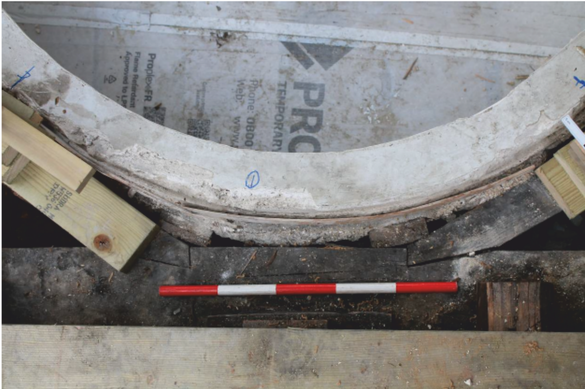
Plate 97 Lantern B: Sub-structure looking east
