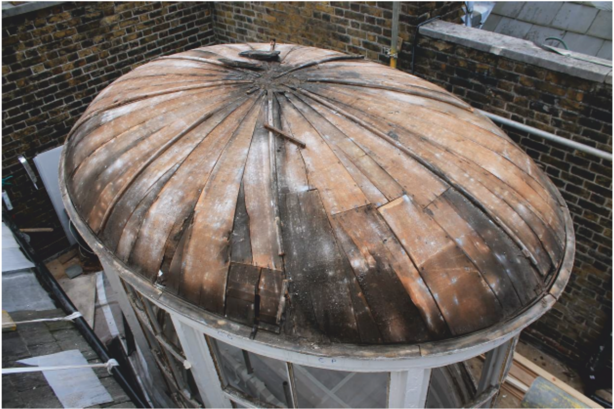
Plate 87 Lantern C: Following removal of leadwork, looking south-east
