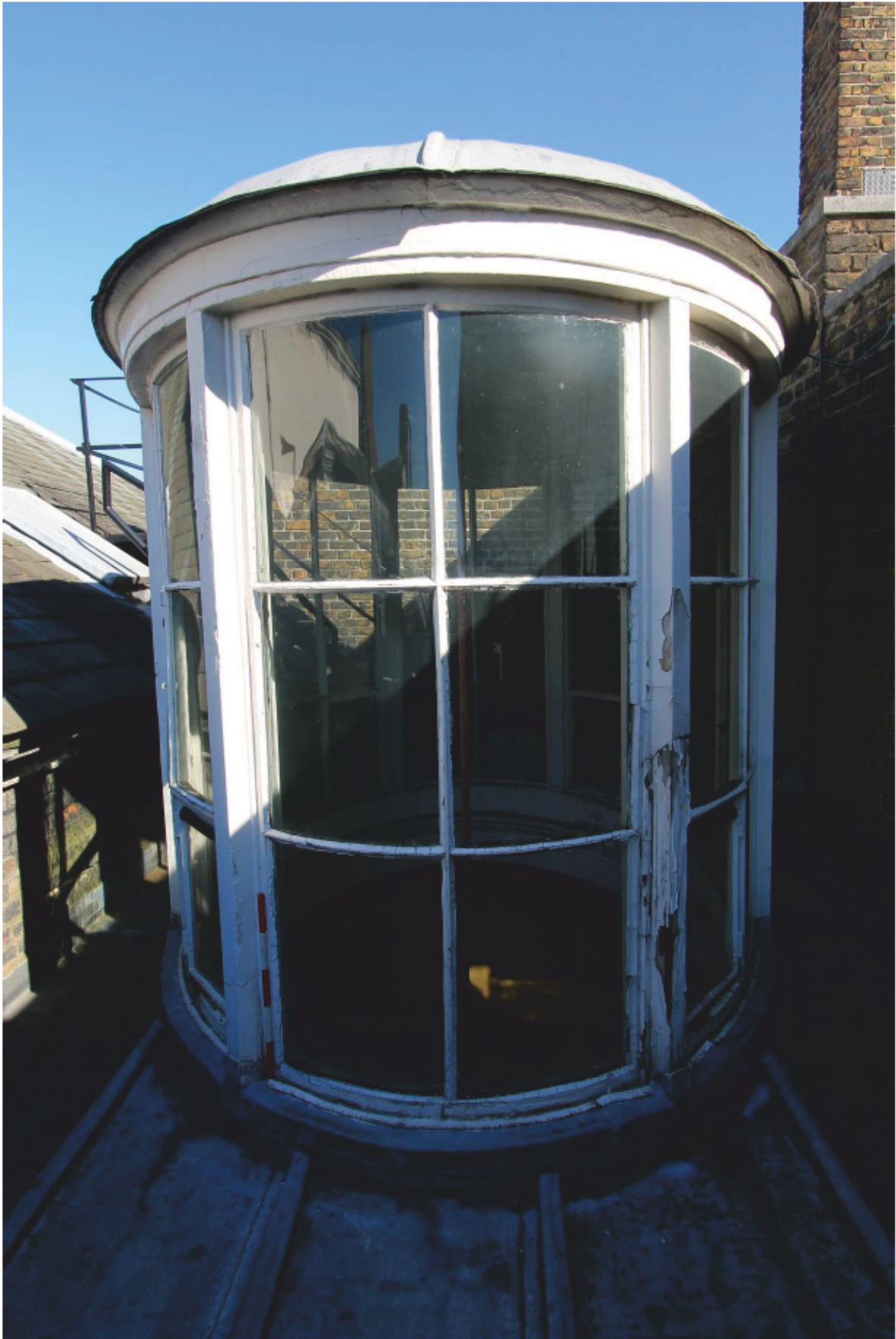
Plate 52 Lantern C: looking east
