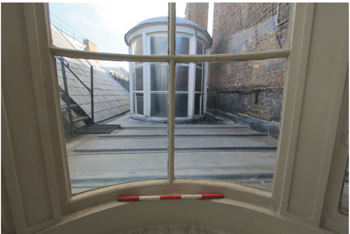
Plate 27 Lantern A: Internal Repair 5
