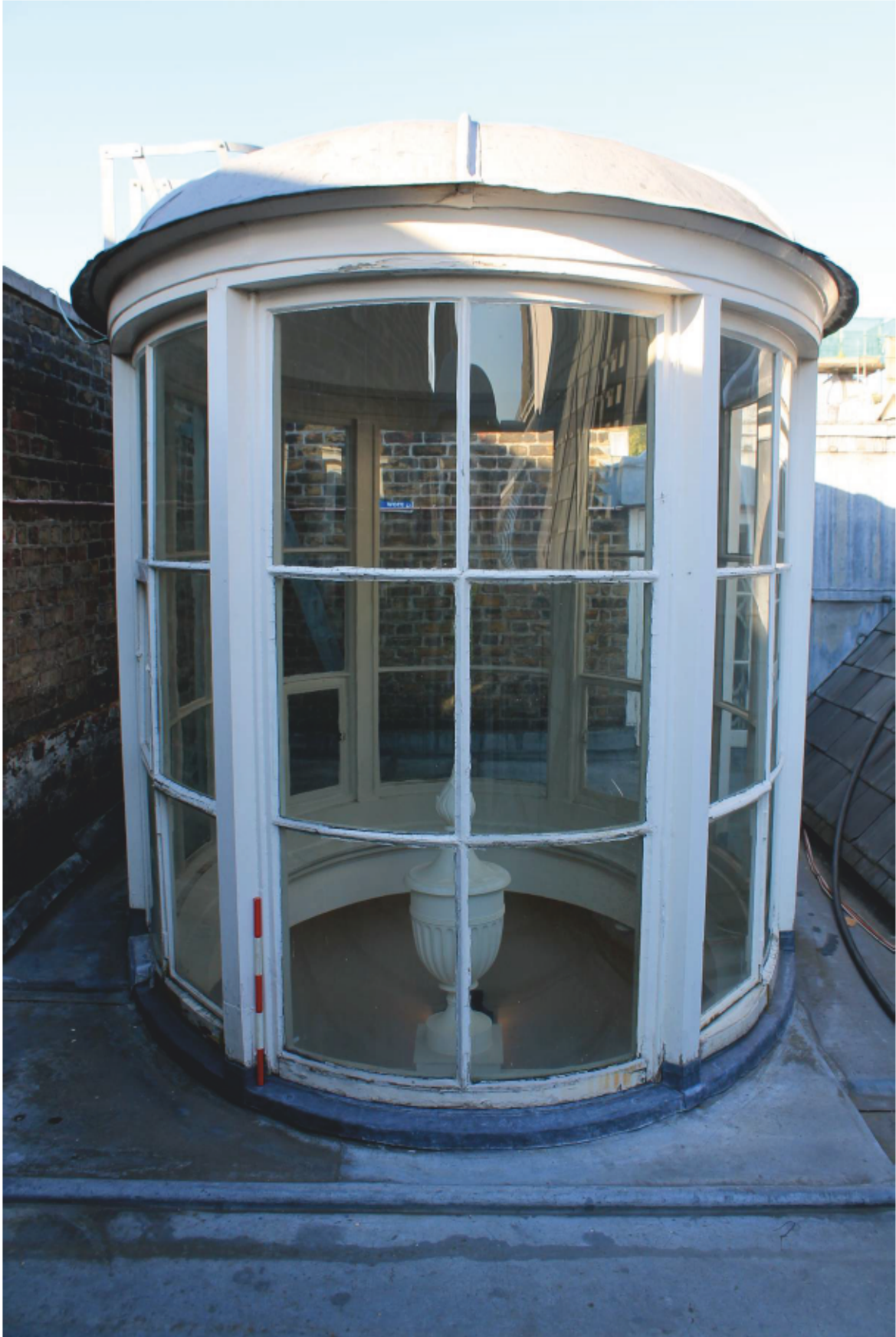
Plate 4 Lantern A looking west
