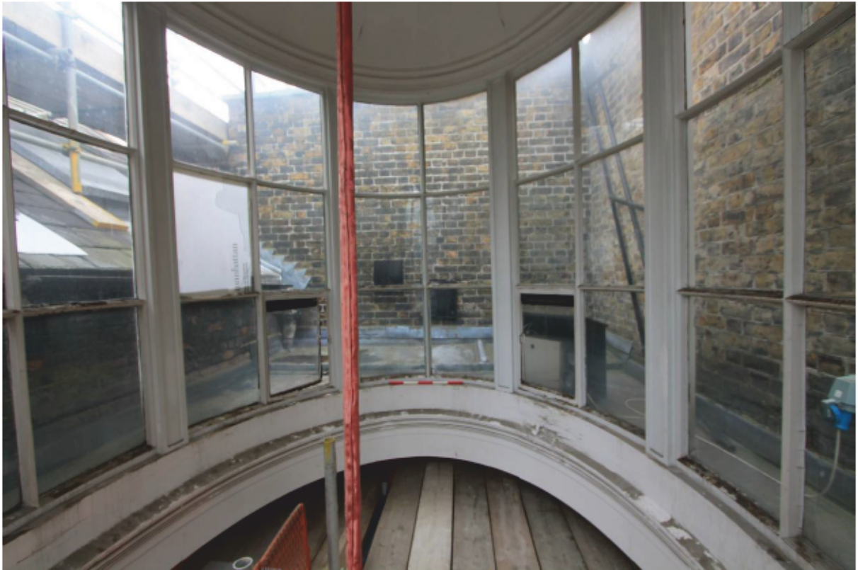
Plate 62 Lantern C: looking east
