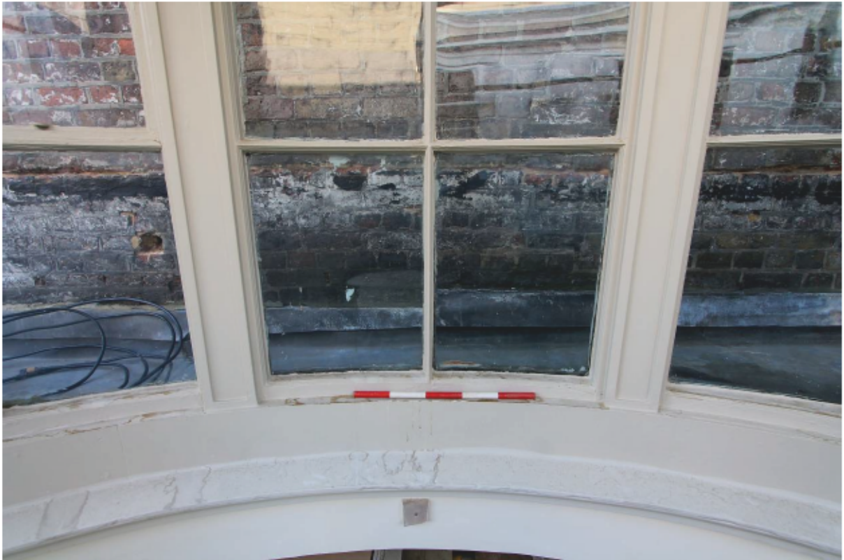
Plate 20 Lantern A: Window Detail looking south
