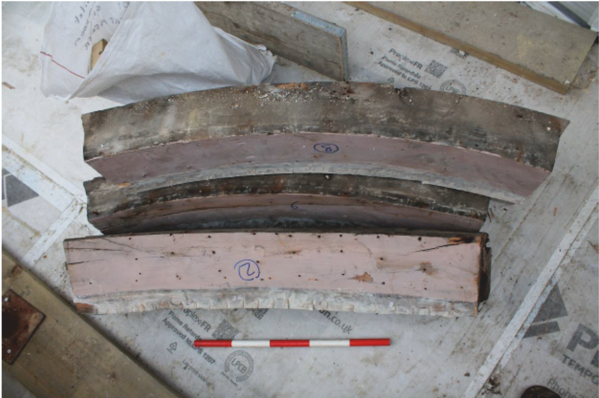
Plate 99 Lantern B: Original sill sections
