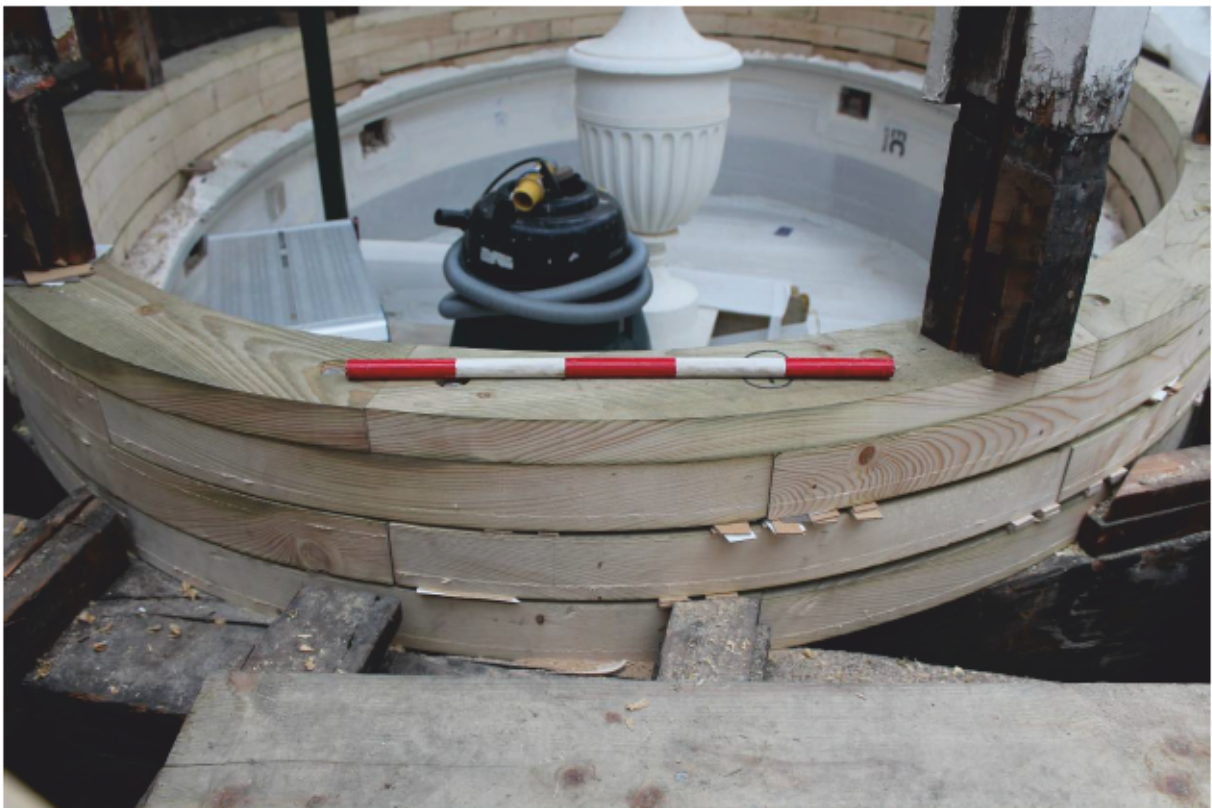
Plate 90 Lantern A: Insertion of new softwood composite sill
