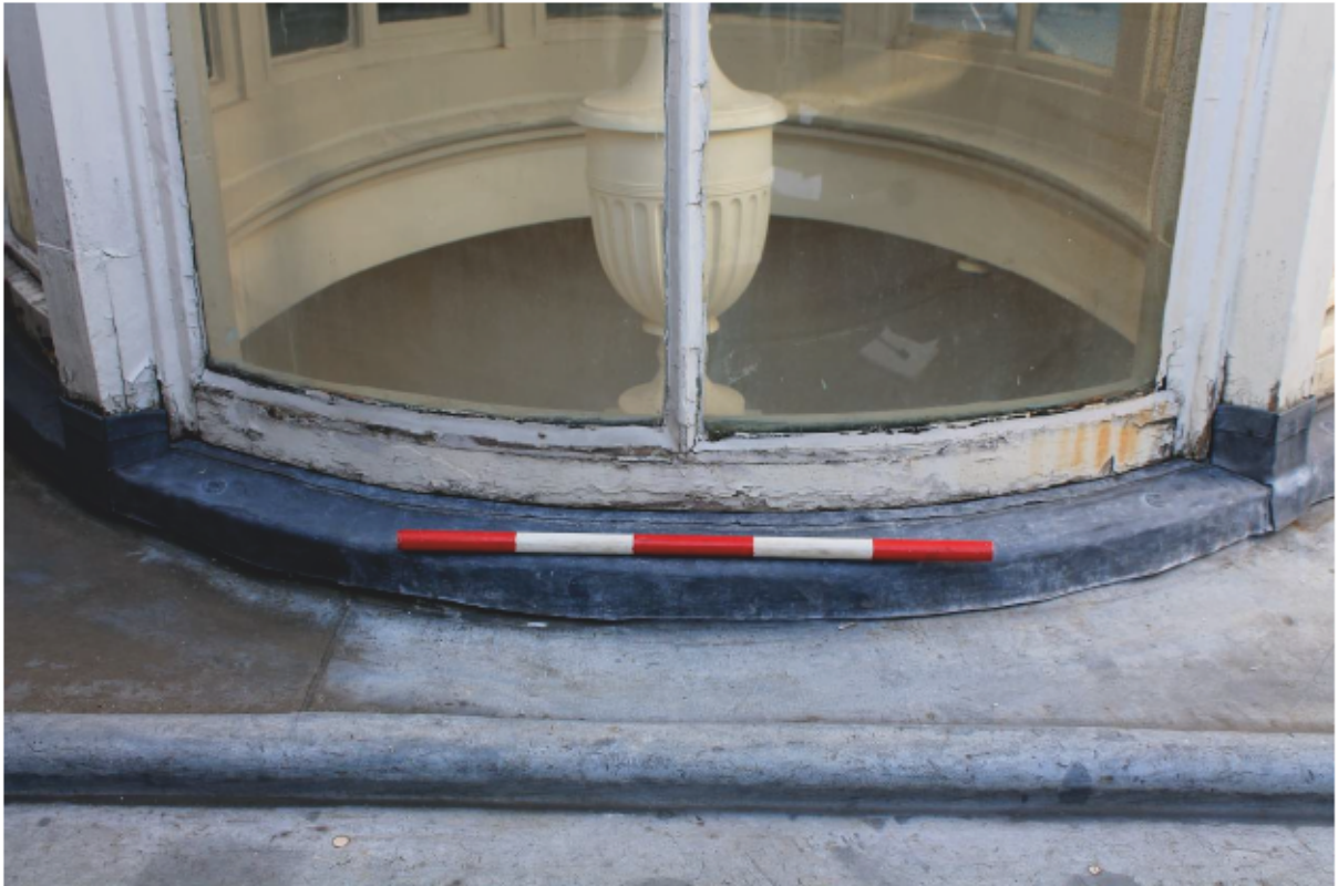
Plate 5 Lantern A: External Repair 1
