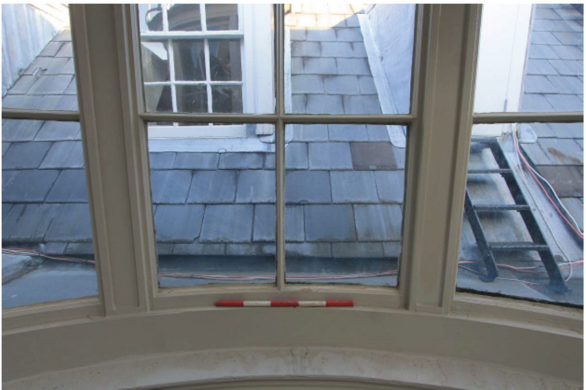
Plate 21 Lantern A: Window Detail looking north
