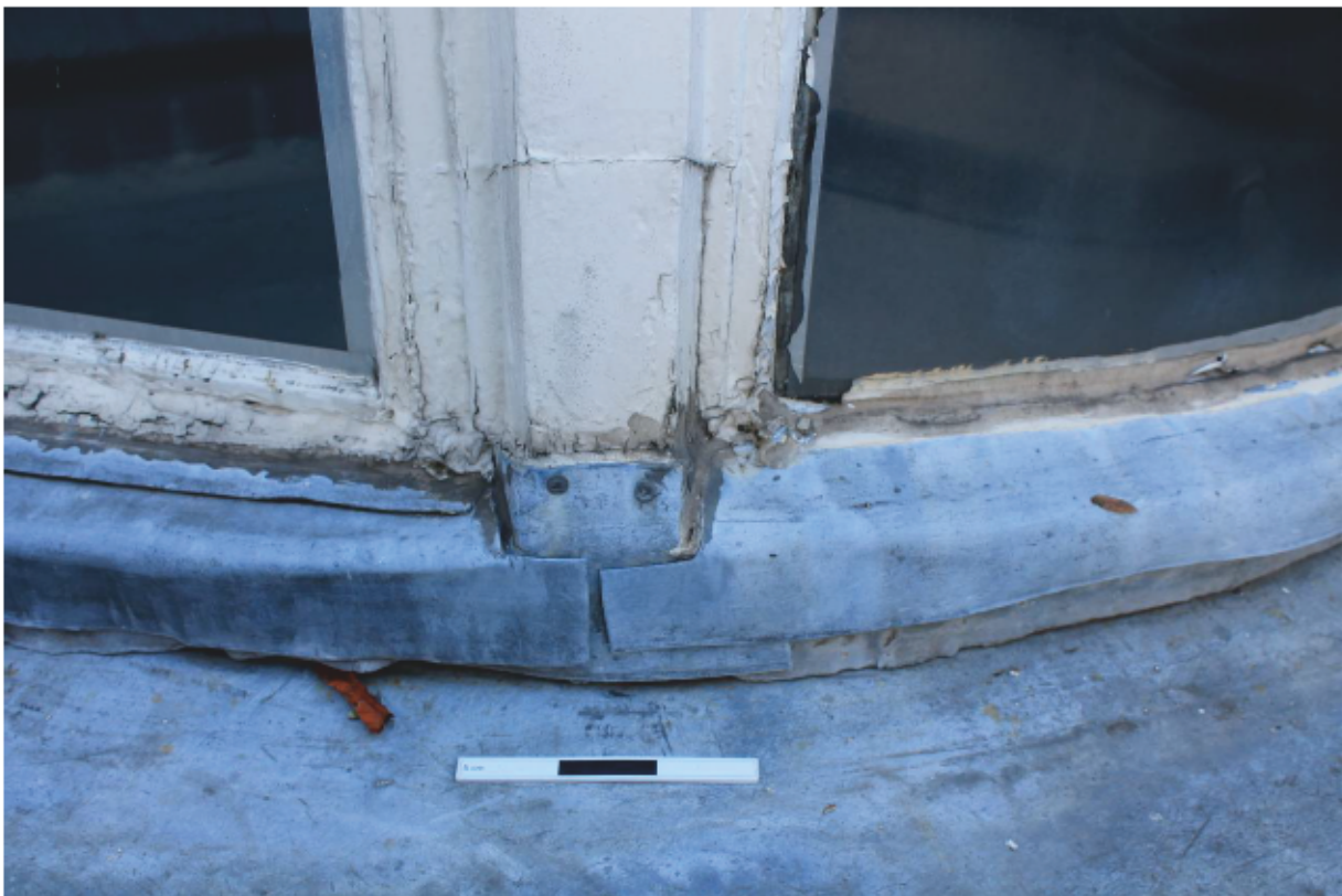
Plate 33 Lantern B: External Repair 16
