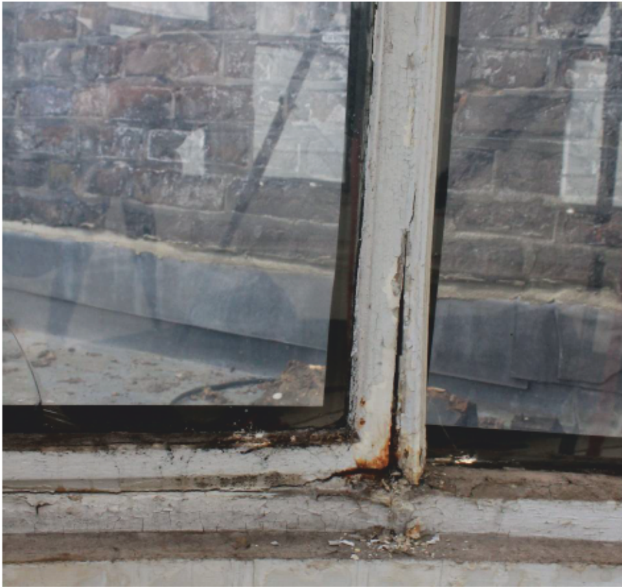
Plate 50 Lantern B: Internal Repair 10
