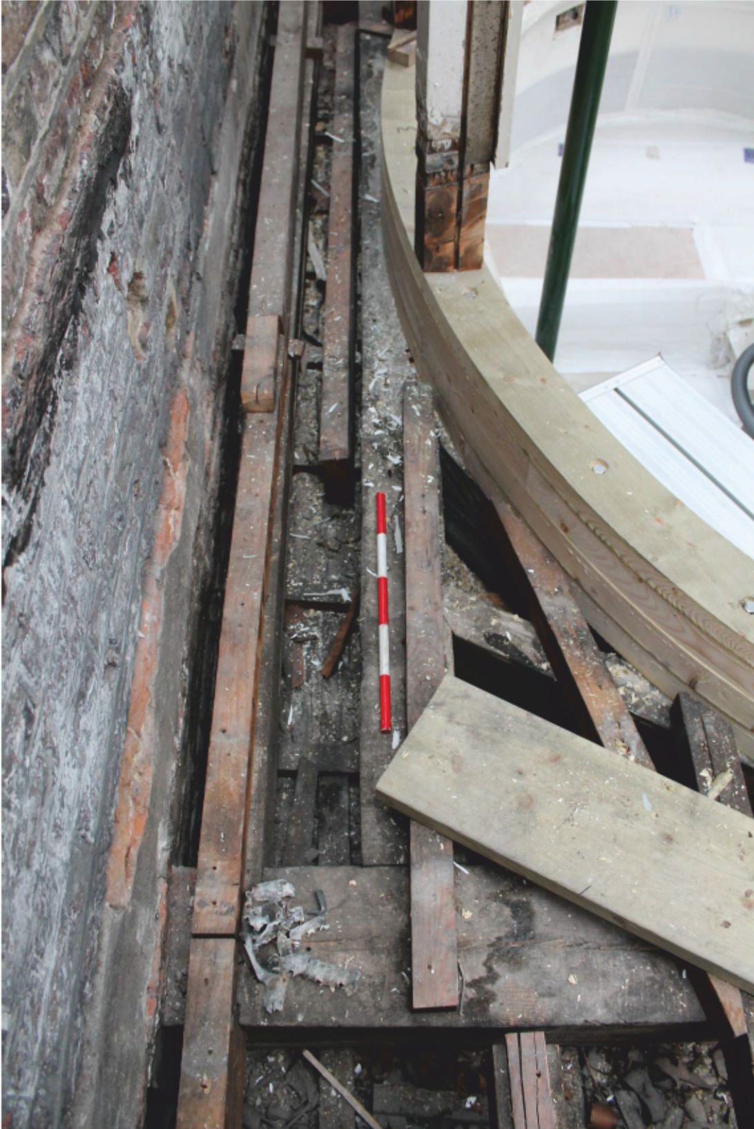
Plate 91 Lantern A: Sub-structure looking west
