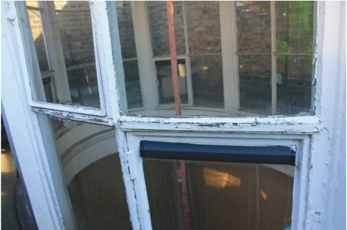
Plate 60 Lantern C: External Repair 34
