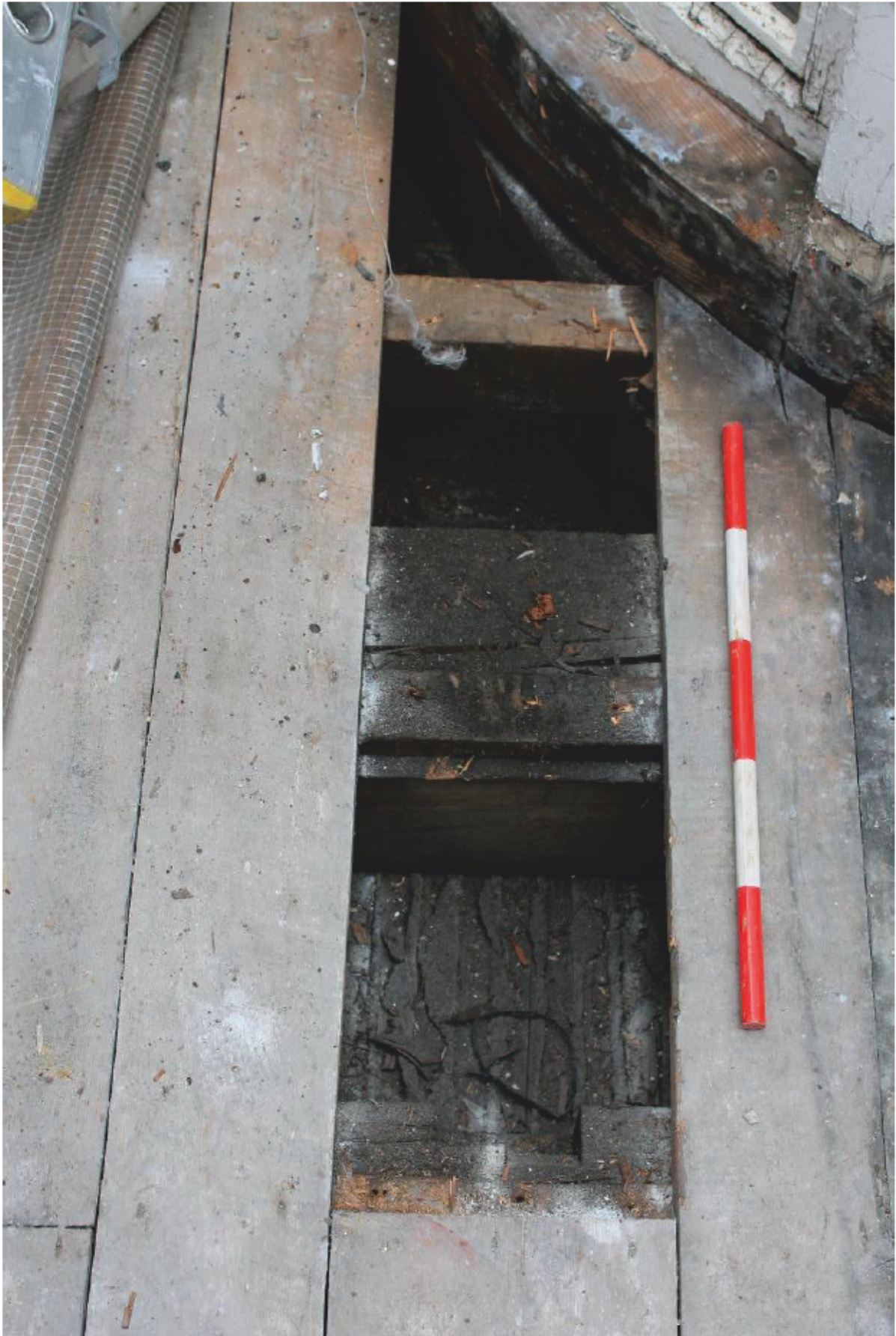
Plate 79 Lantern C: Opening C1 looking east
