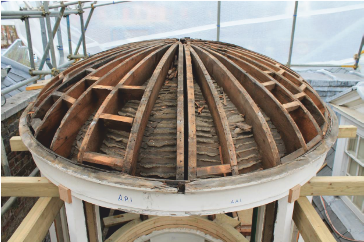
Plate 83 Lantern A: Following removal of sarking boards, looking west
