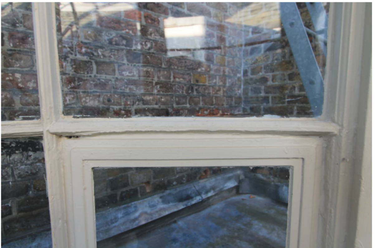
Plate 25 Lantern A: Internal Repair 3
