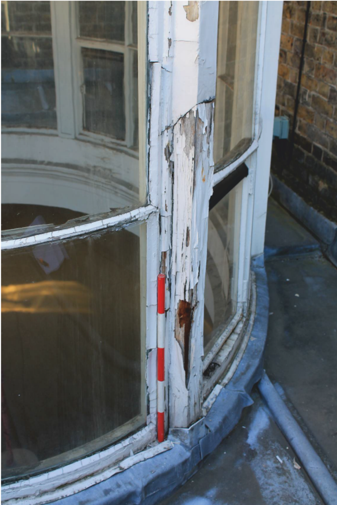
Plate 53 Lantern C: External Repair 27
