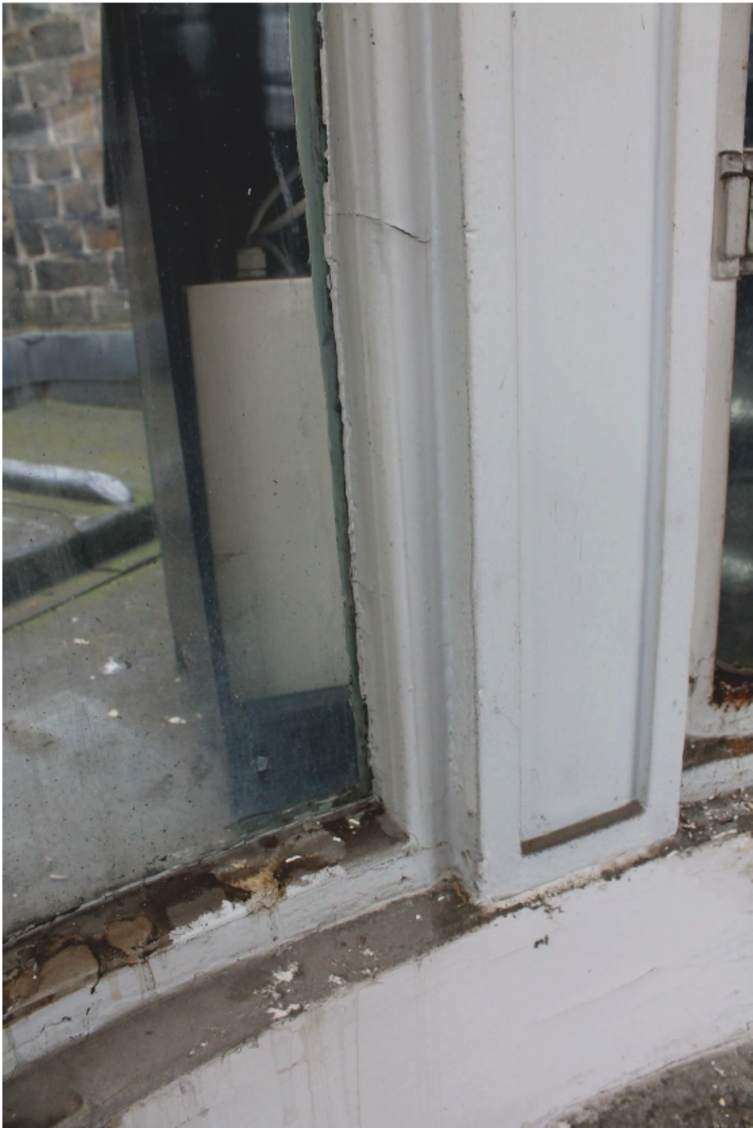
Plate 68 Lantern C: Internal Repair 16
