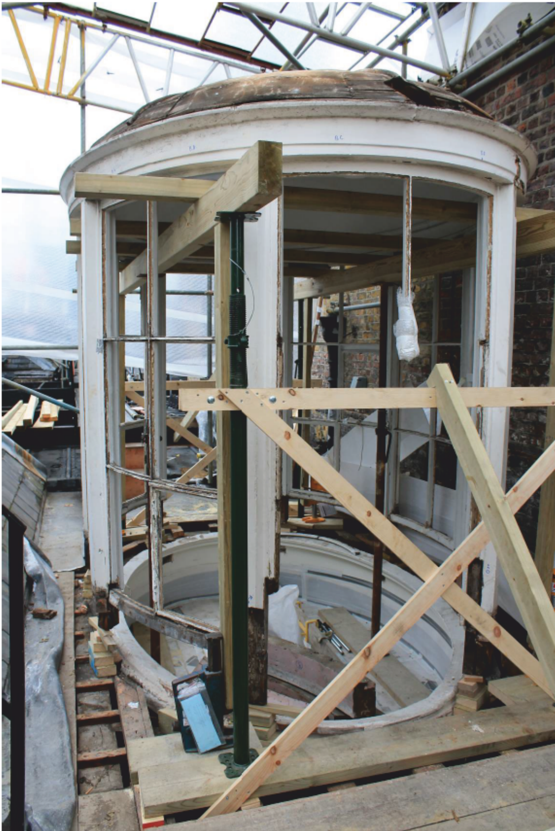
Plate 95 Lantern B, support structure, looking east
