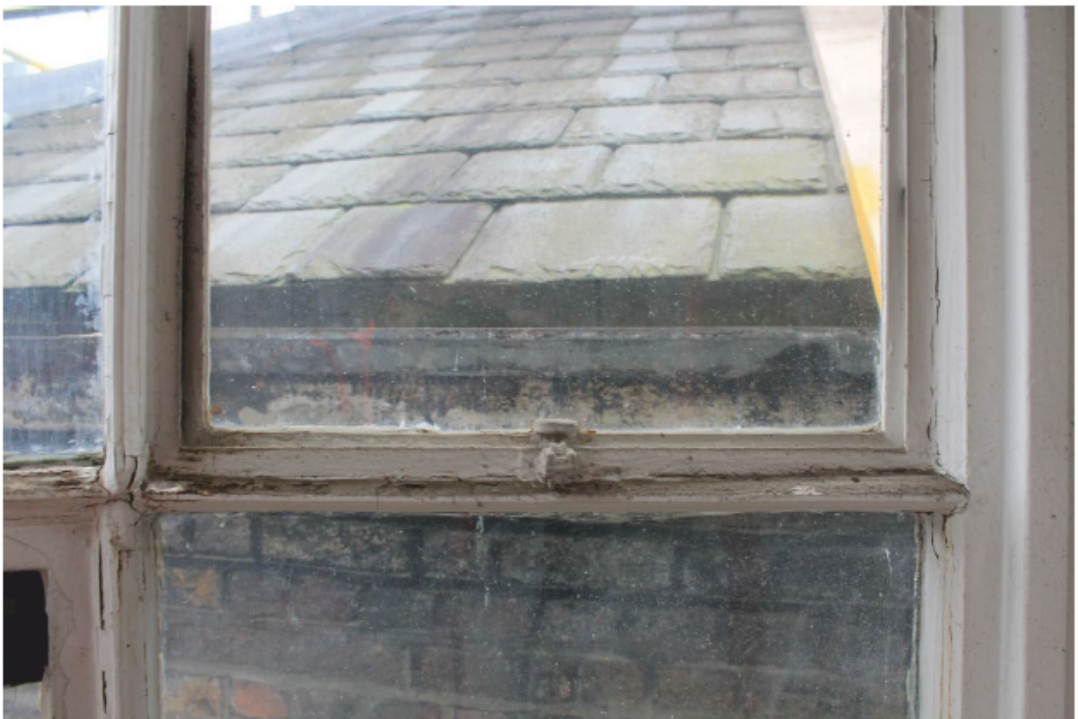
Plate 67 Lantern C: Internal Repair 15
