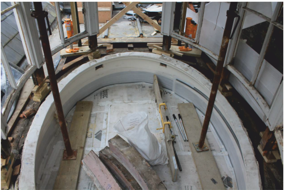
Plate 94 Raising of Lantern B, internal, looking east
