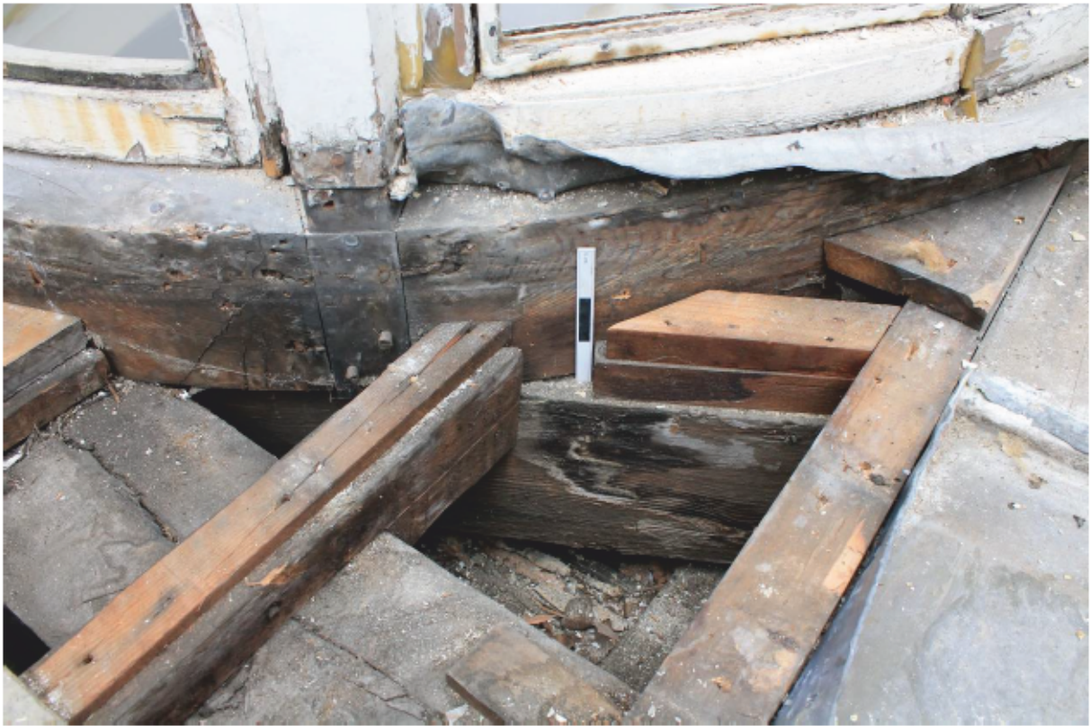
Plate 74 Opening A1: Detail of sectional sill and supporting sub-structure looking south-west
