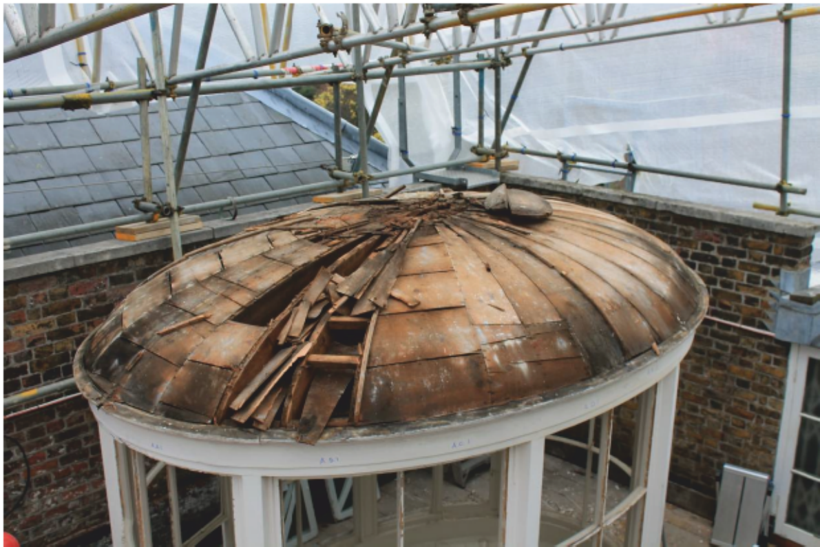
Plate 82 Lantern A: Following removal of lead flashings and ribs
