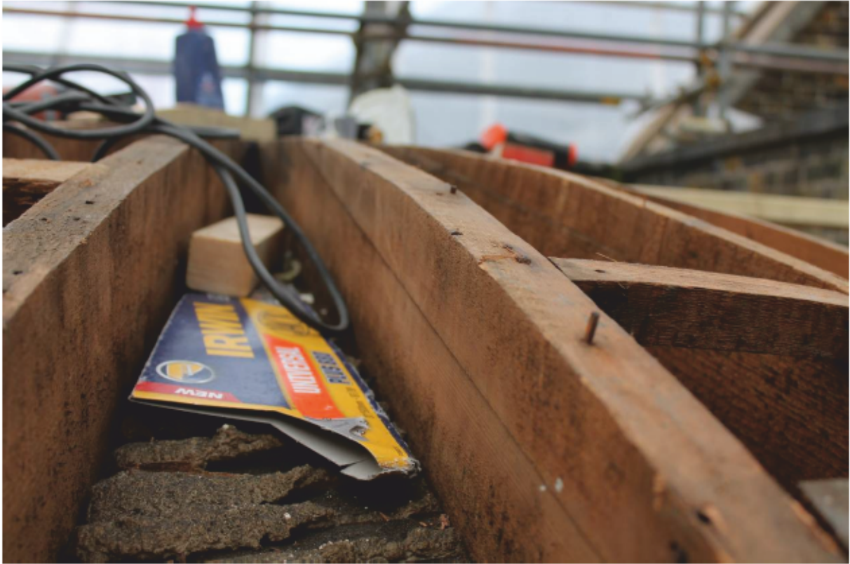
Plate 89 Lantern C: Composite rafter
