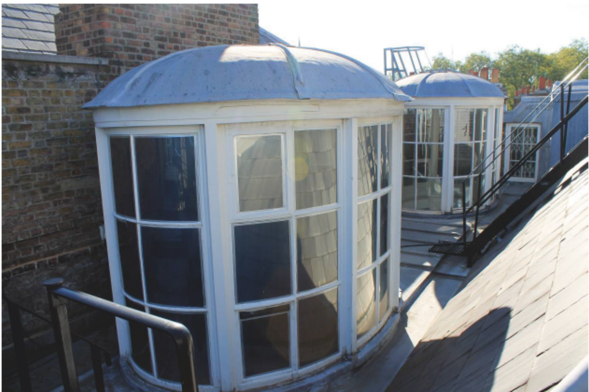
Plate 2 Lanterns B & A looking west
