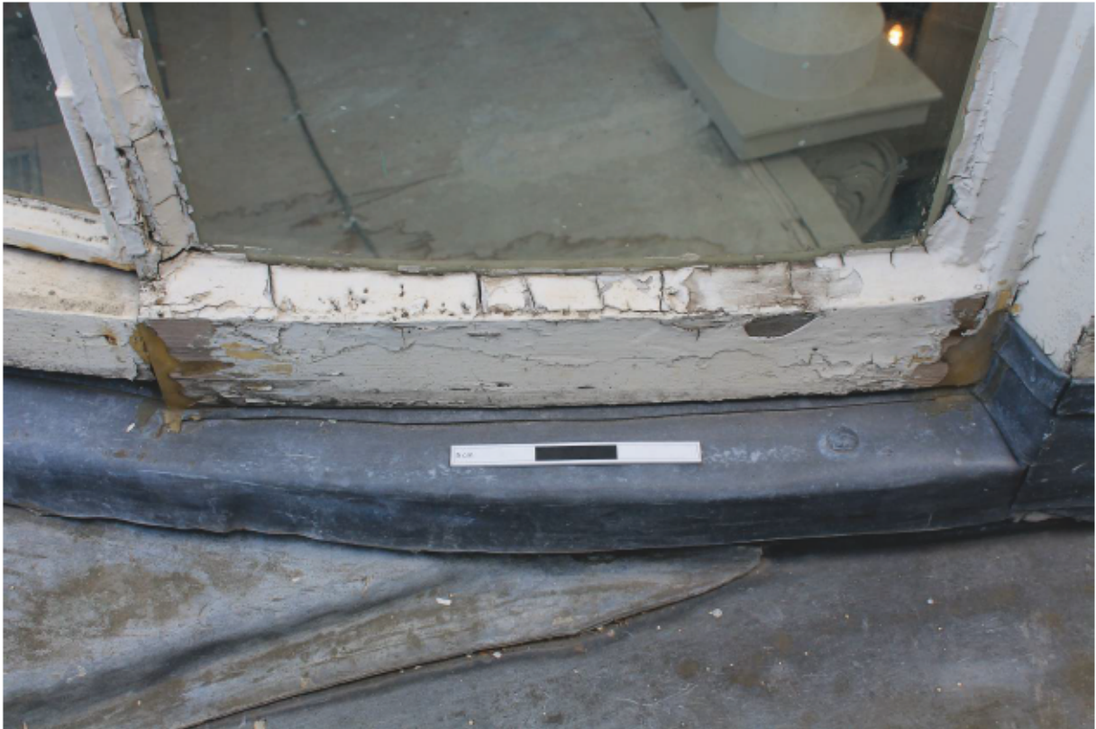
Plate 7 Lantern A: External Repair 4
