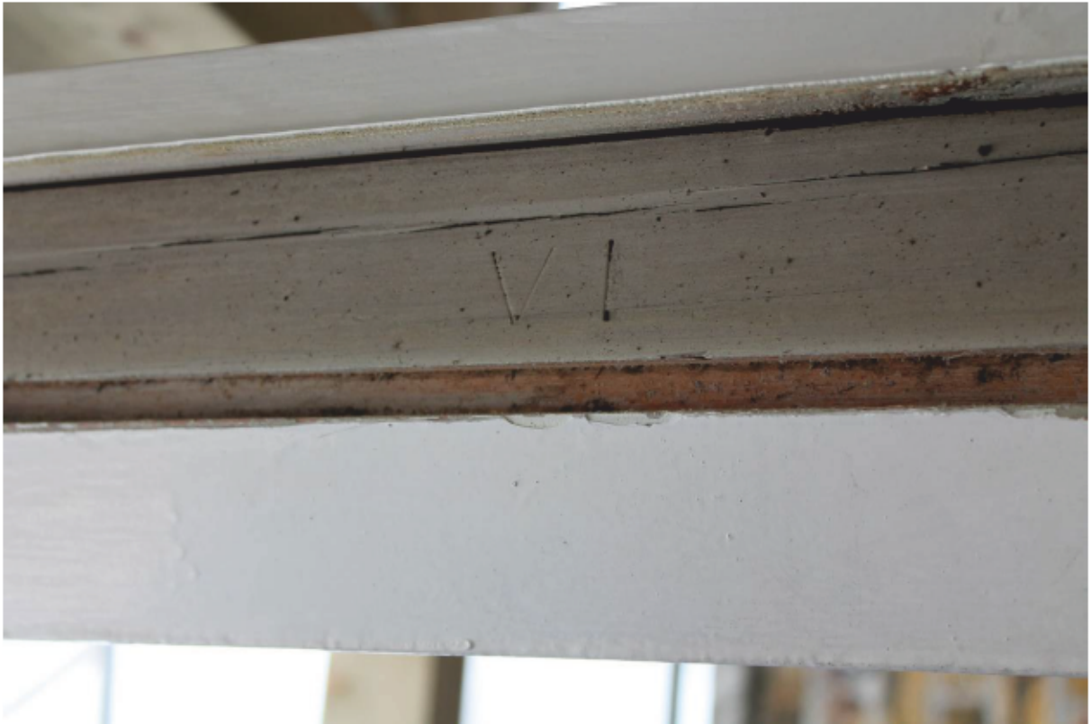
Plate 101 Lantern A: Roman marking to mullion (mid-post)
