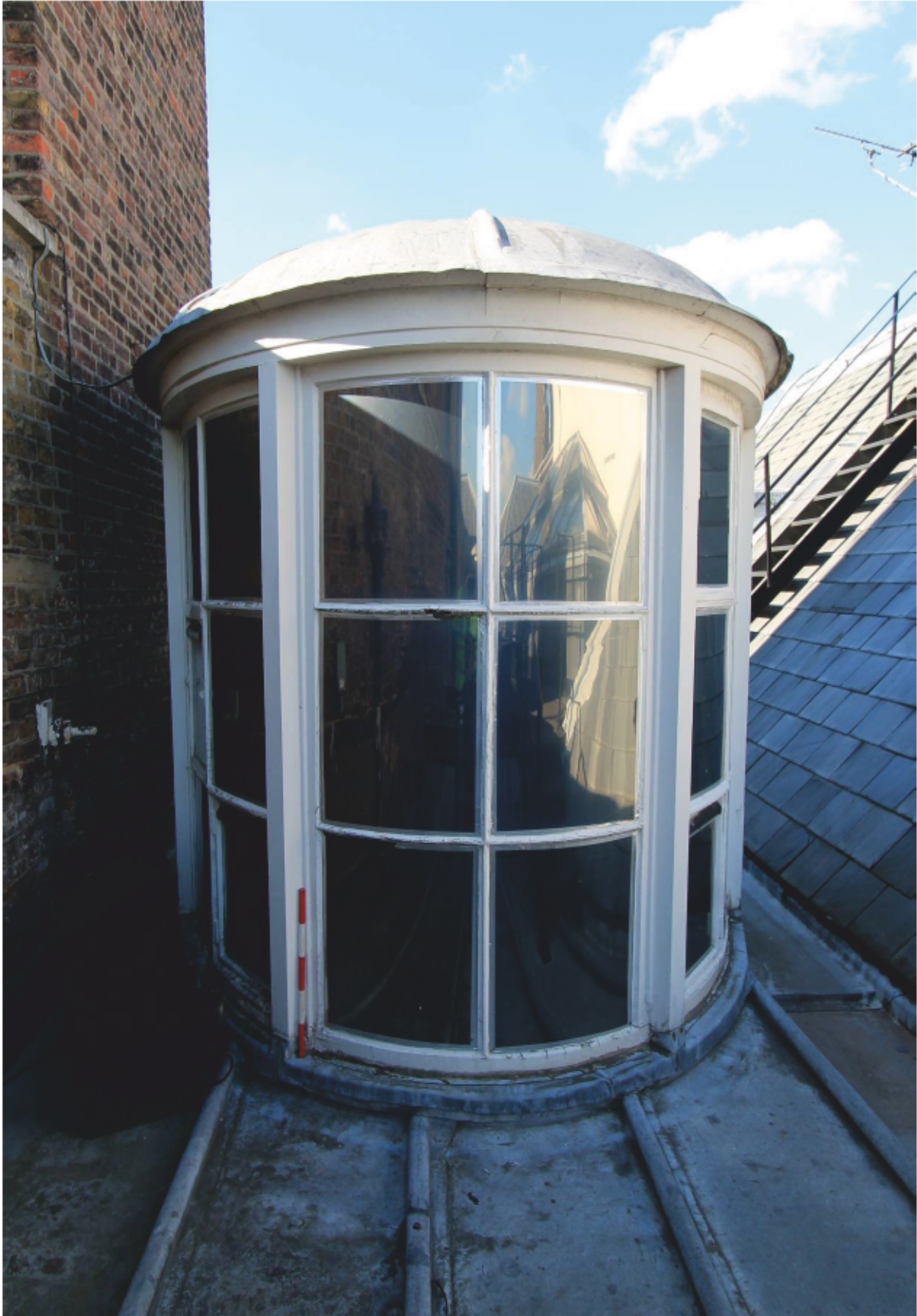
Plate 31 Lantern B: looking west
