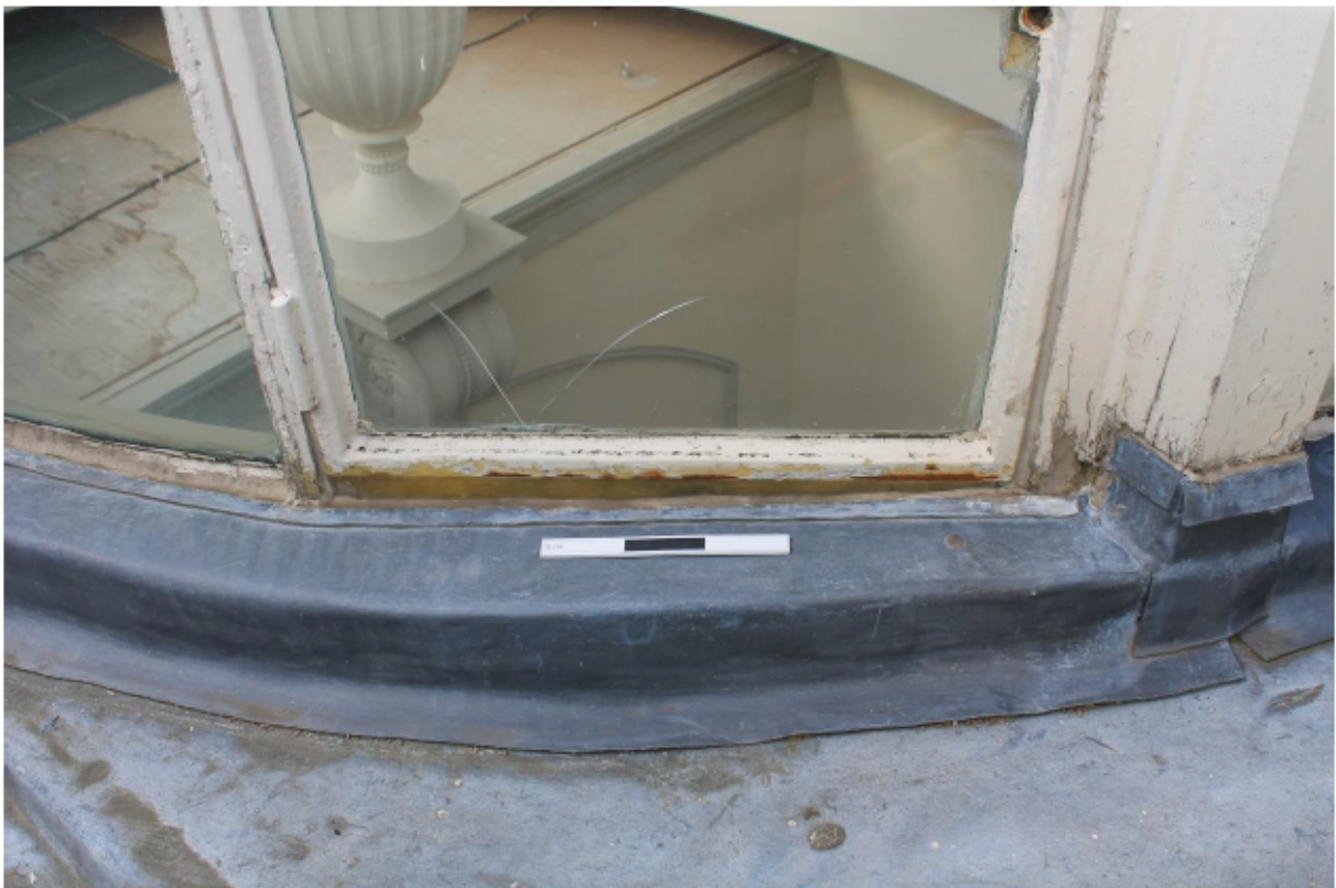
Plate 10 Lantern A: External Repair 7
