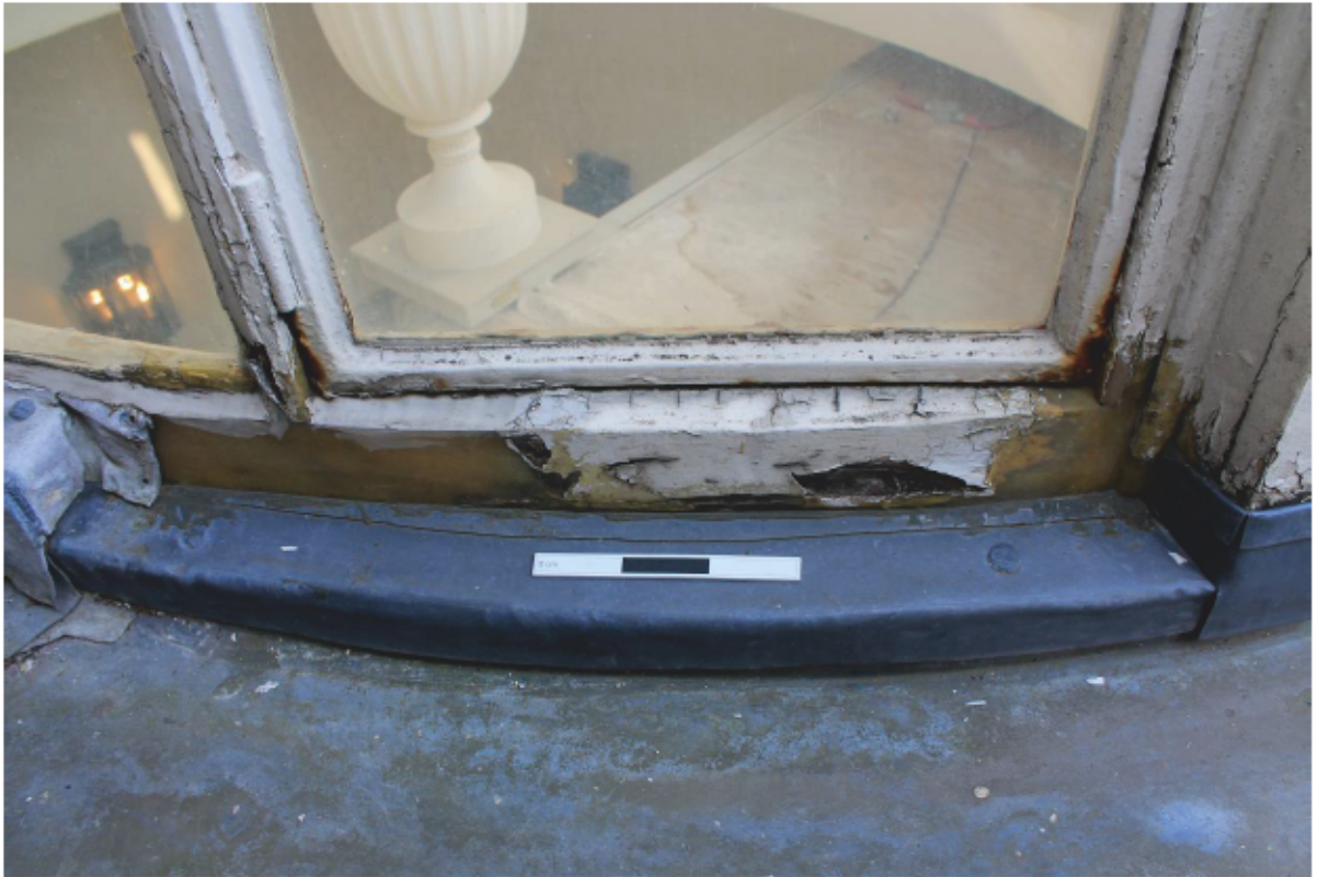
Plate 14 Lantern A: External Repair 11
