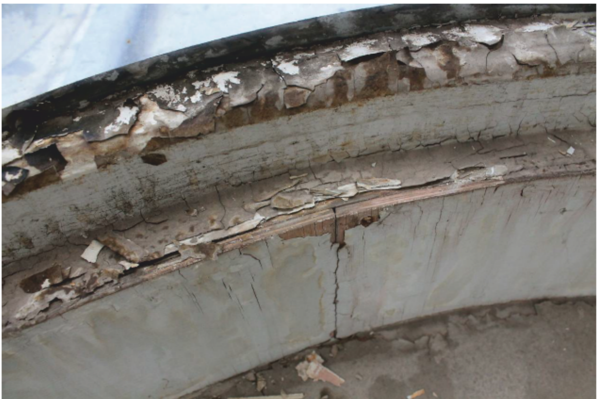
Plate 51 Lantern B: Internal Repair 11
