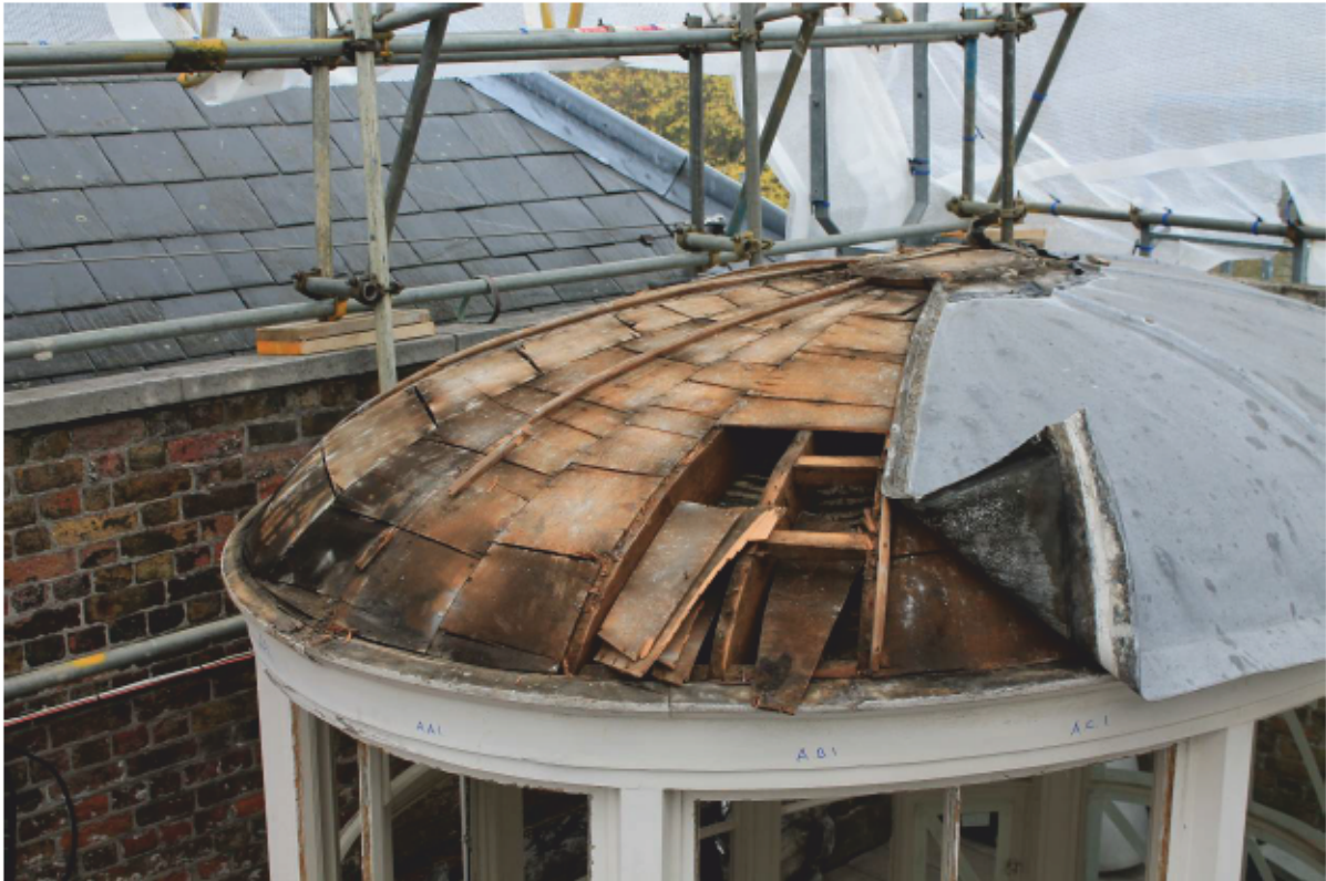
Plate 81 Lantern A: Stripping of domed roof exposing sarking boards, looking south-west
