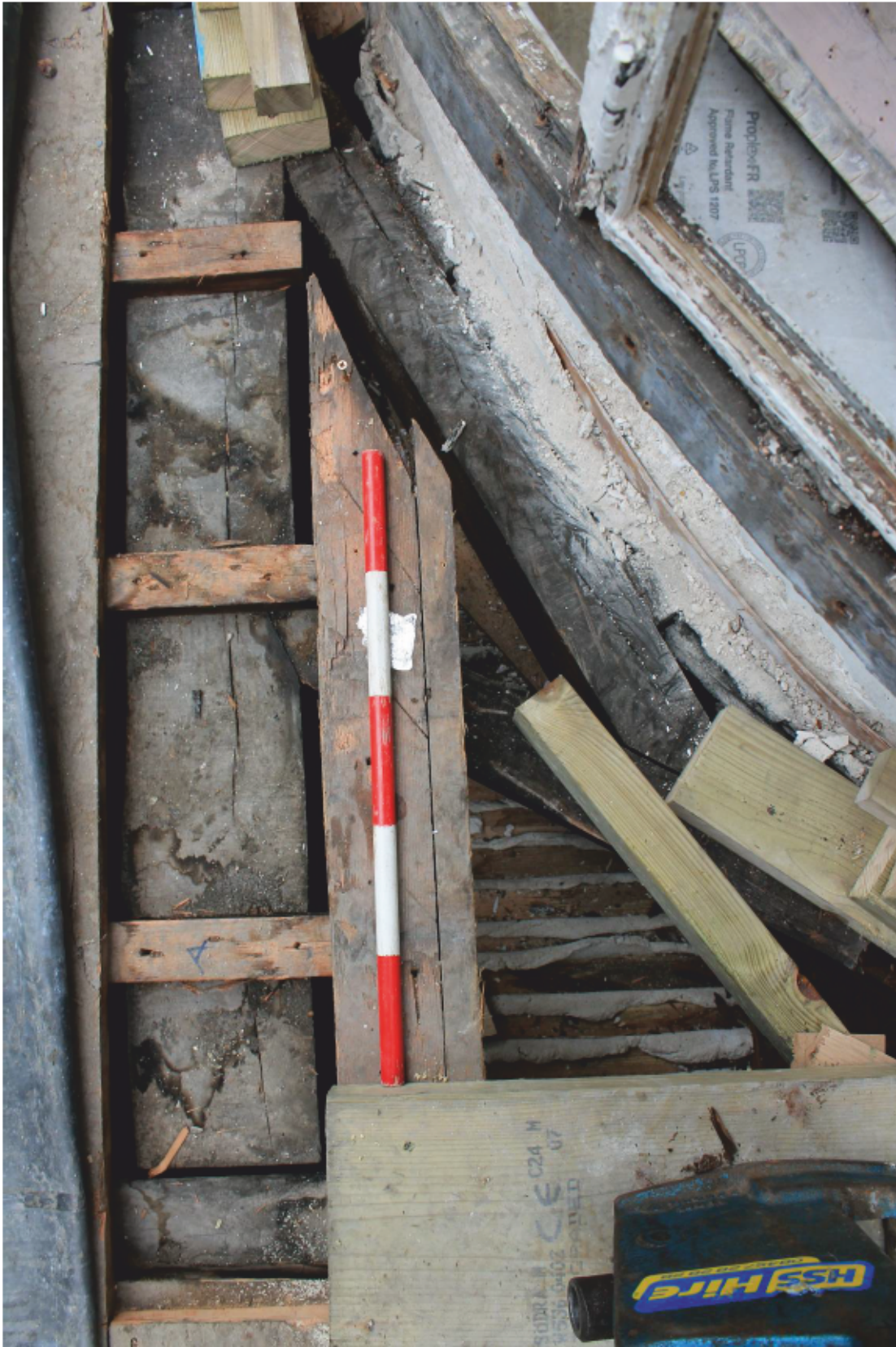
Plate 96 Lantern B: Sub-structure looking east
