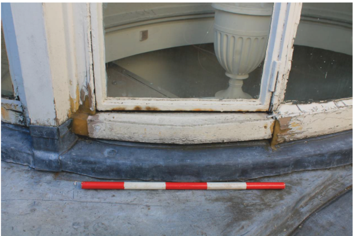
Plate 6 Lantern A: External Repair 3
