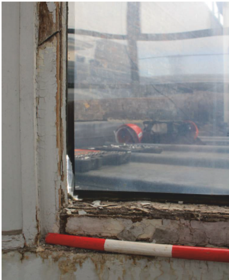
Plate 49 Lantern B: Internal Repair 9
