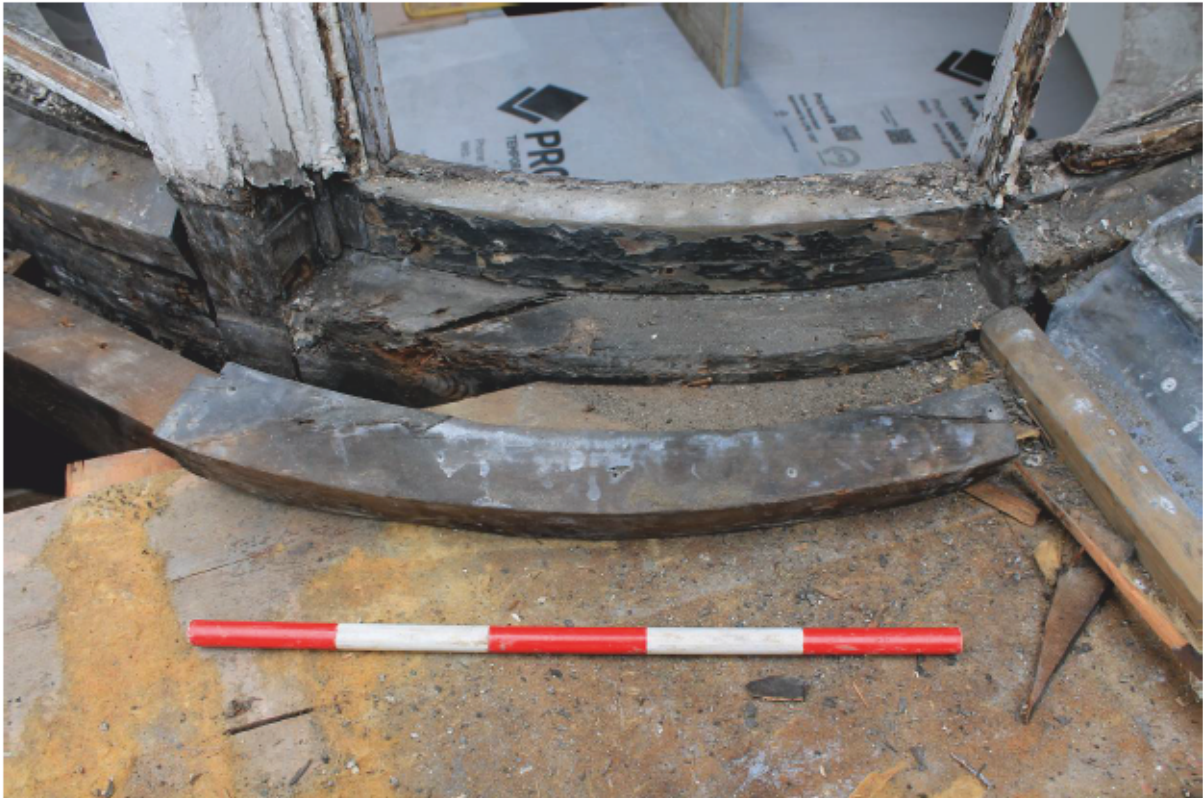
Plate 78 Lantern B: Later sill heightening (removed)
