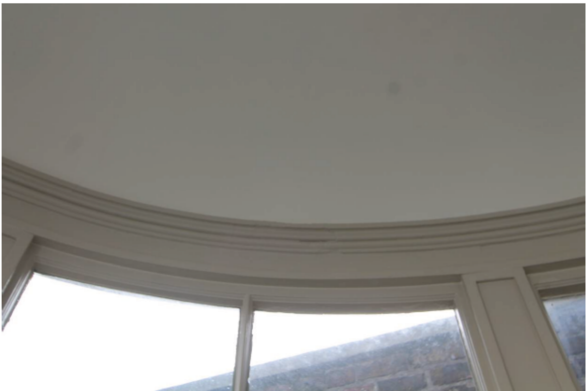
Plate 29 Lantern A: Detail of Cornice
