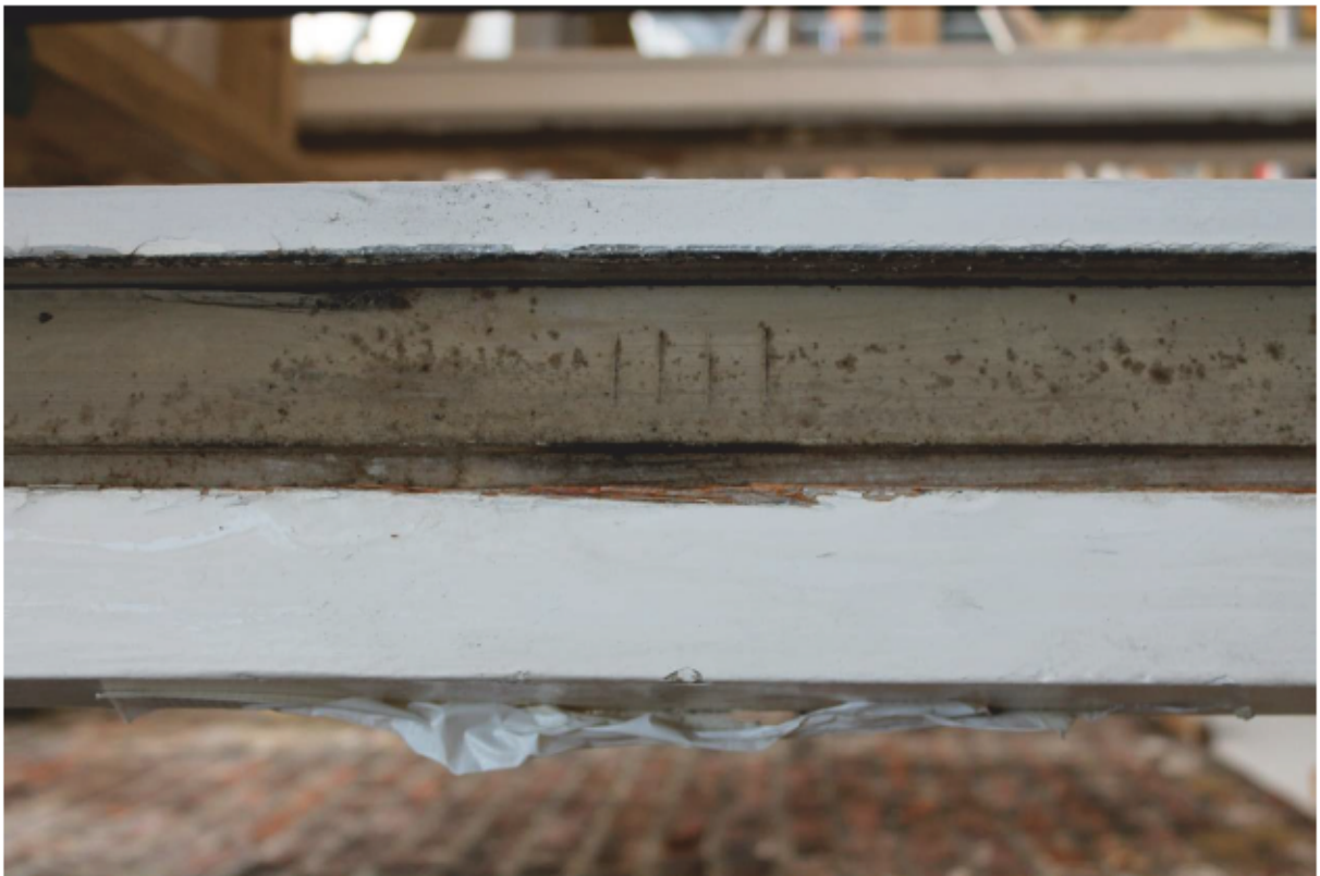
Plate 102 Lantern B: Roman marking to mullion (mid post)
