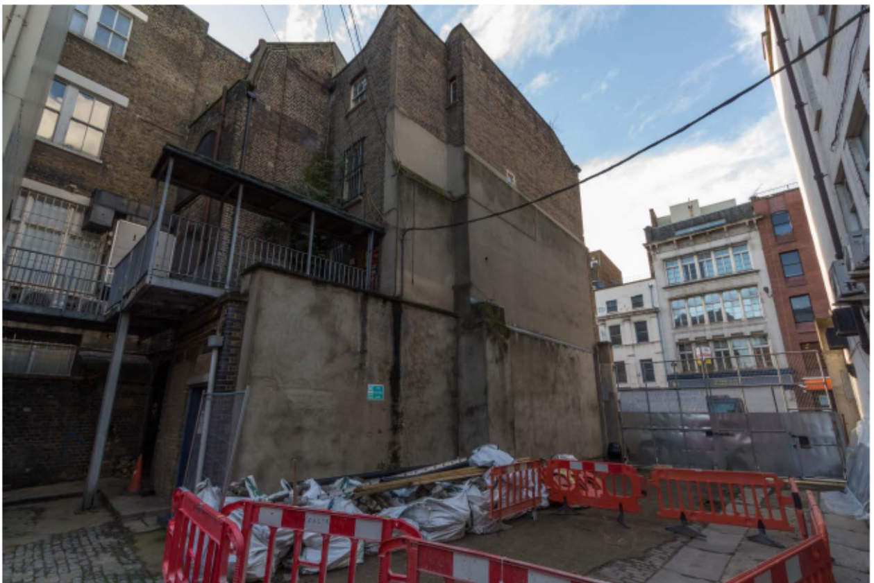
Plate 7 North (side) elevation of no. 141 Borough High Street, looking south-west
