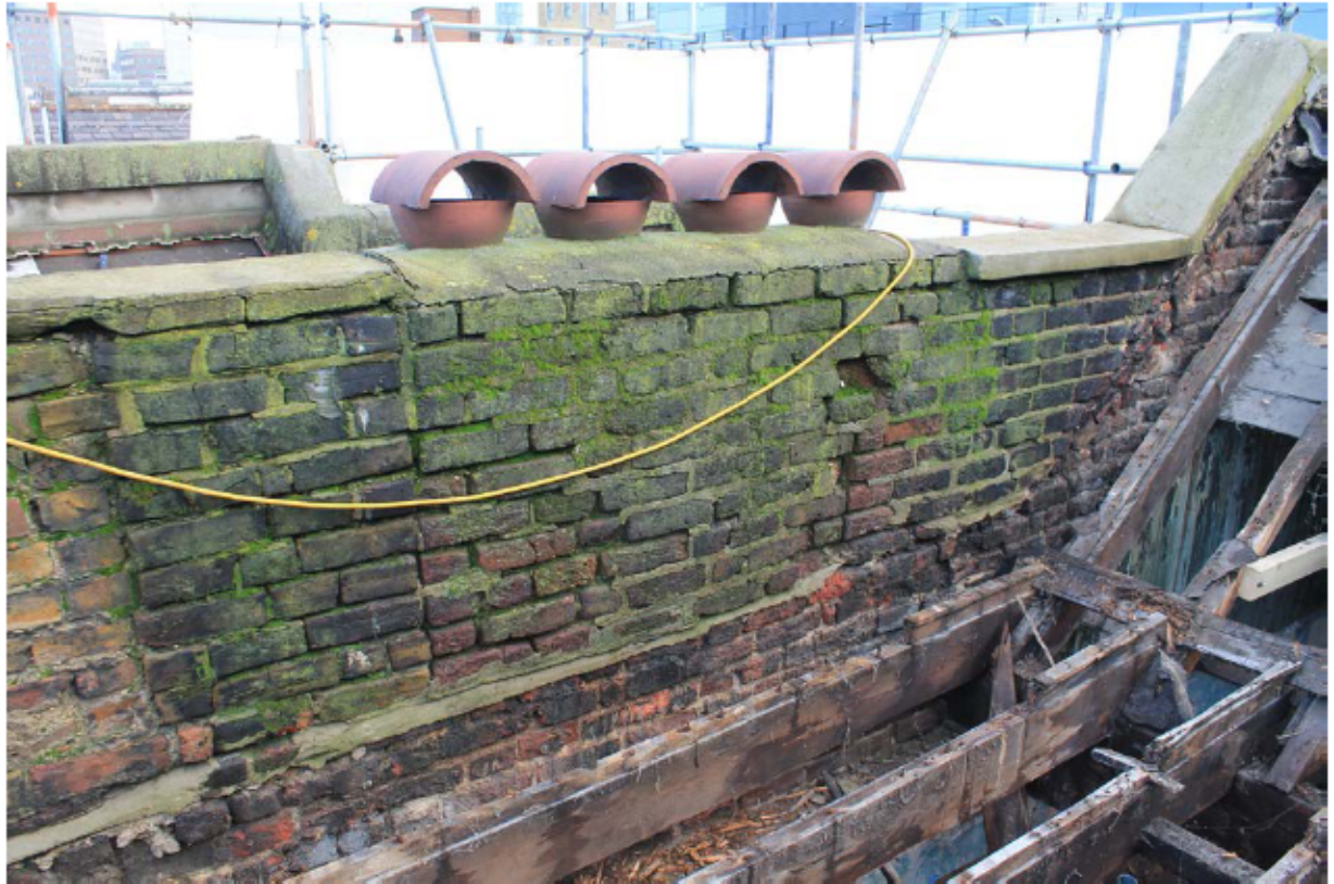
Plate 86: Fire break party wall between nos 141 and 143 Borough High Street during stripping, looking north-east from the roof of no. 143 Borough High Street
