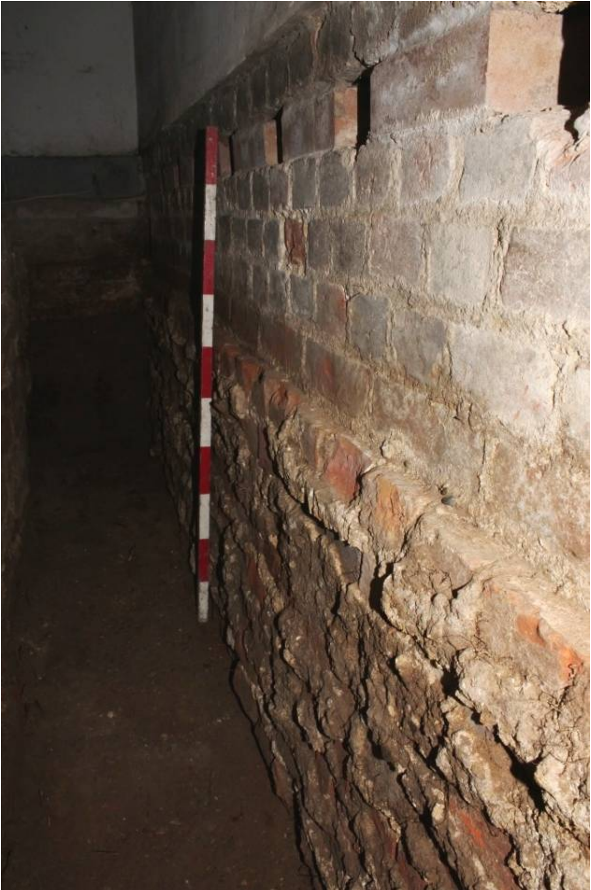
Plate 27 South face of north bath house wall, looking west
