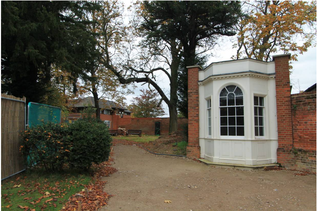
Plate 1 West elevation of the bath house, looking east
