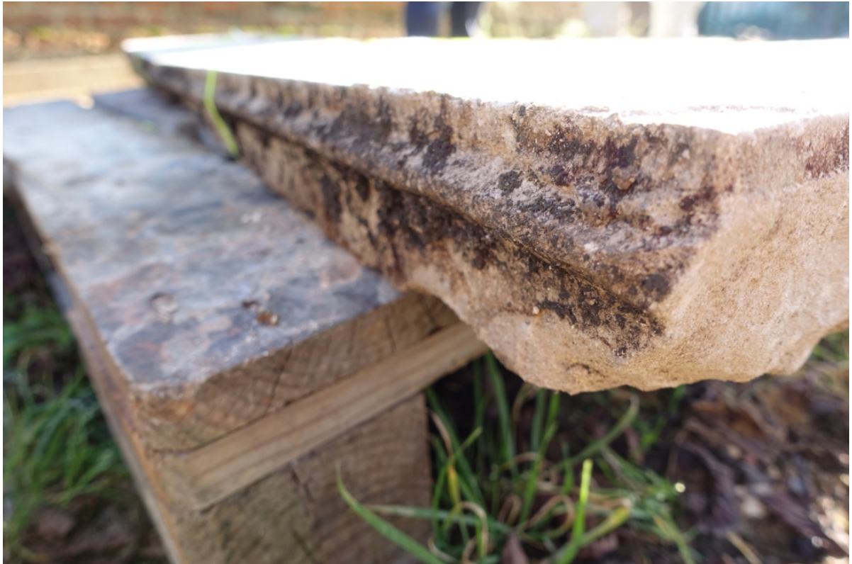
Plate 30 Integral lip or tongue along the edge of an ex-situ Portland Stone slab, which had lined the bath
