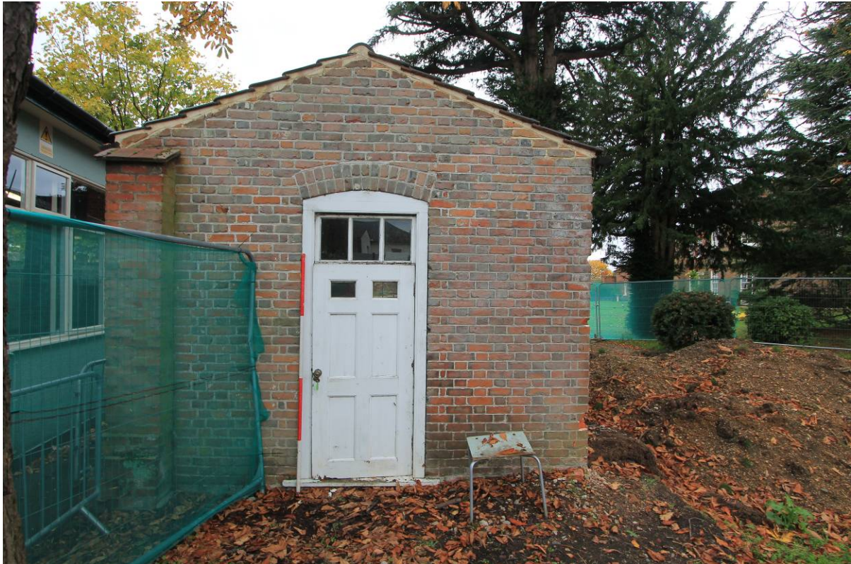
Plate 5 Eastern elevation of the bath house, looking west
