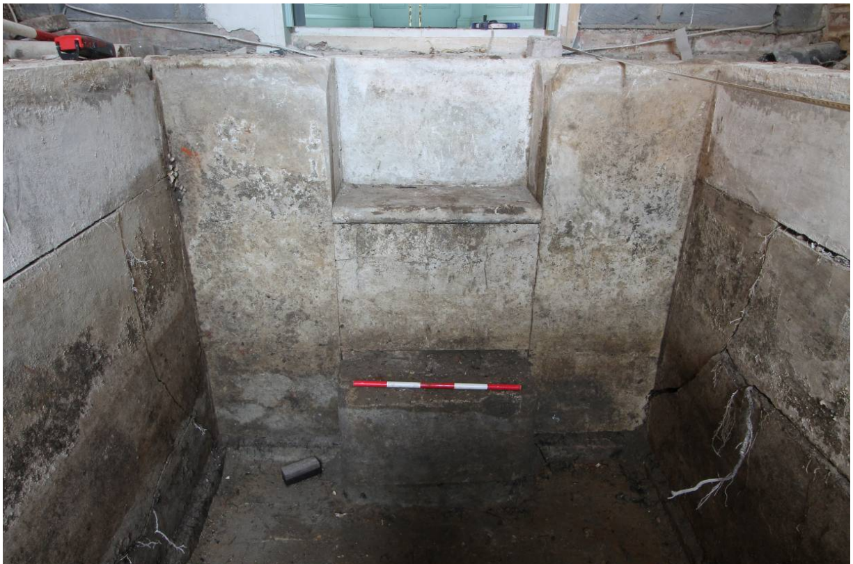
Plate 14 West wall and step into bath, looking west
