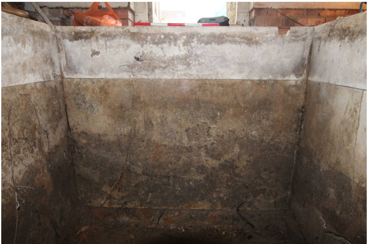
Plate 18 East wall of bath, looking east
