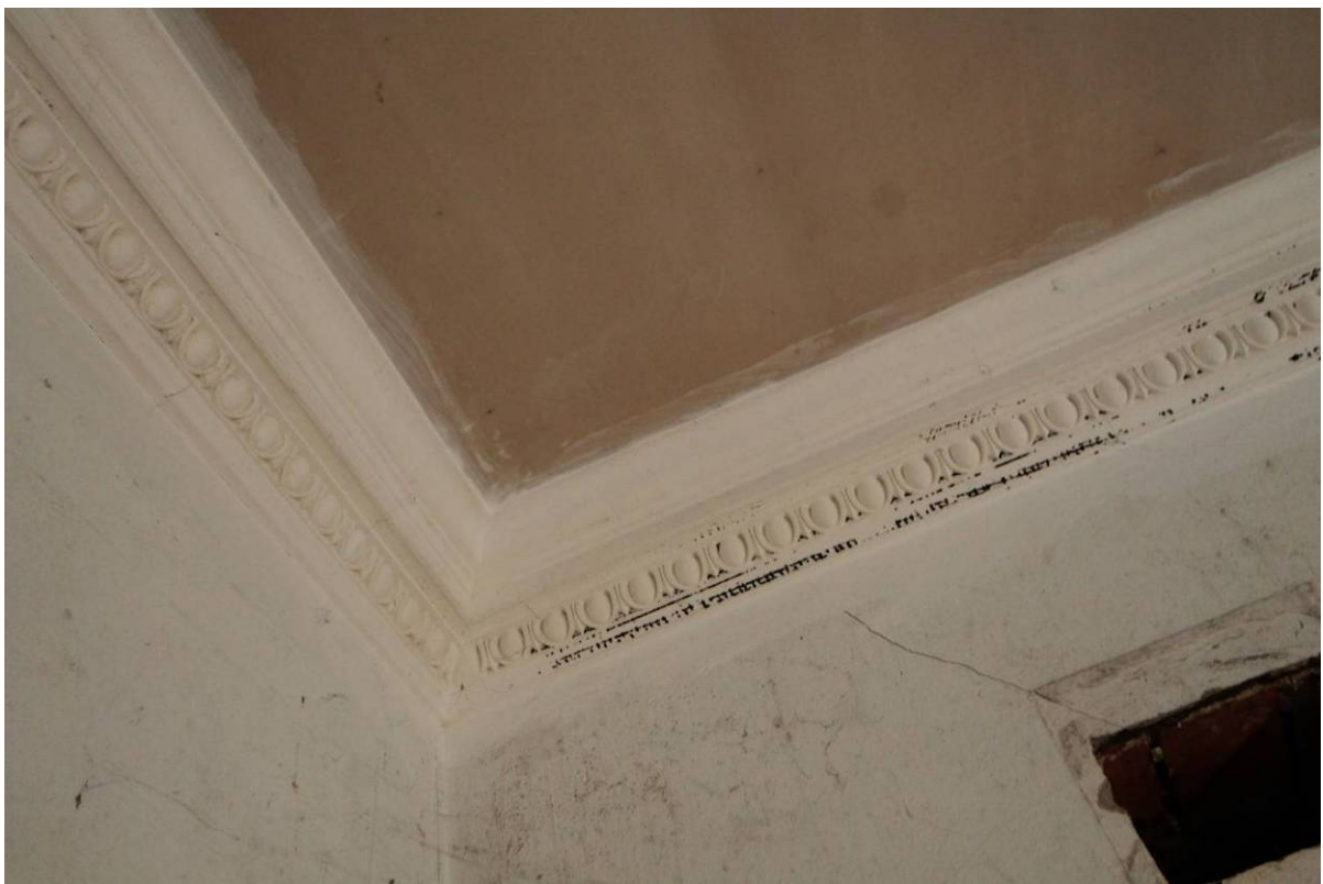
Plate 8 Bathing Room (A) detail of egg and dart cornice, looking south-west
