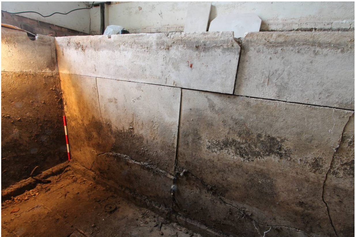
Plate 16 South wall of bath, looking south-east
