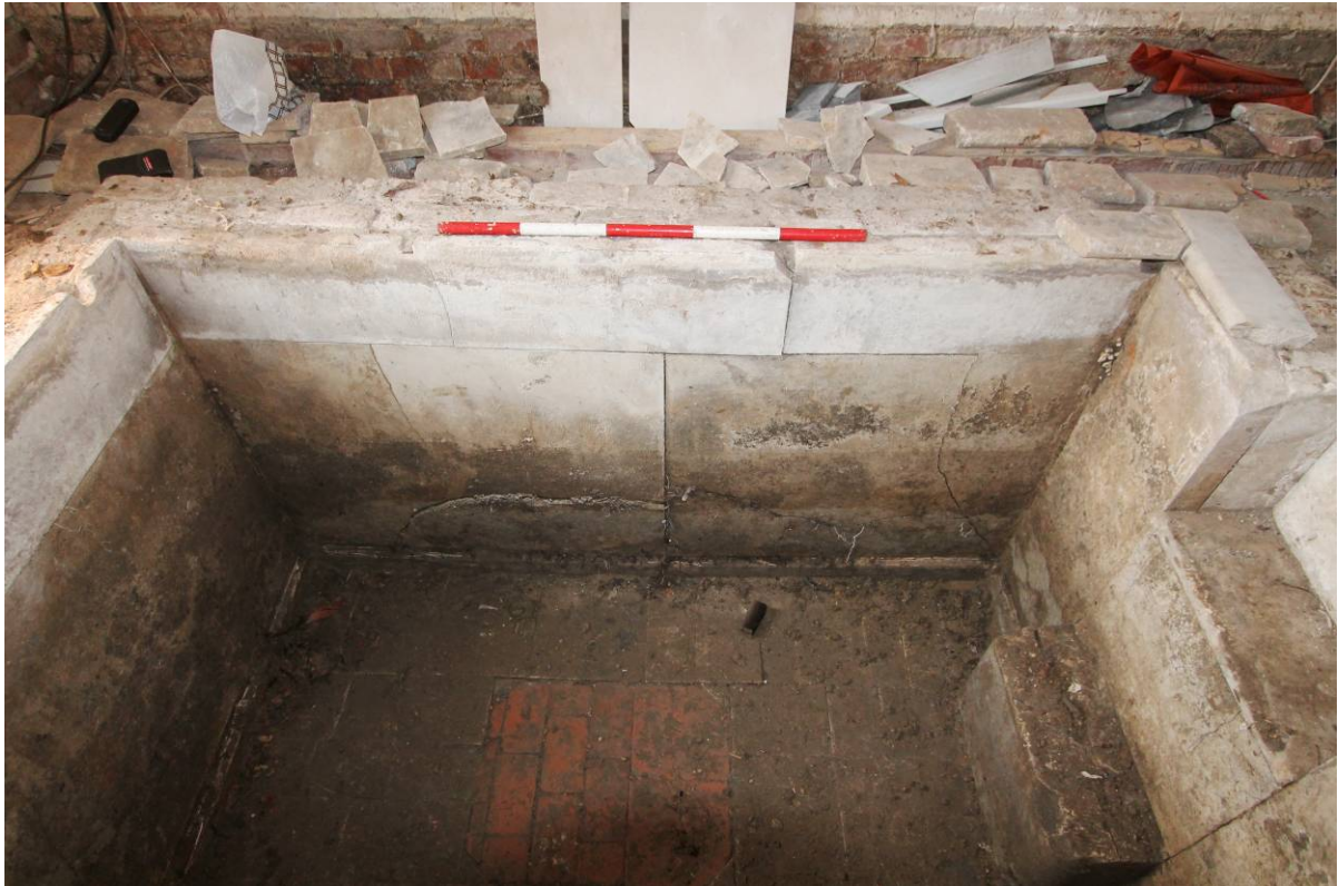
Plate 17 South wall of bath, looking south
