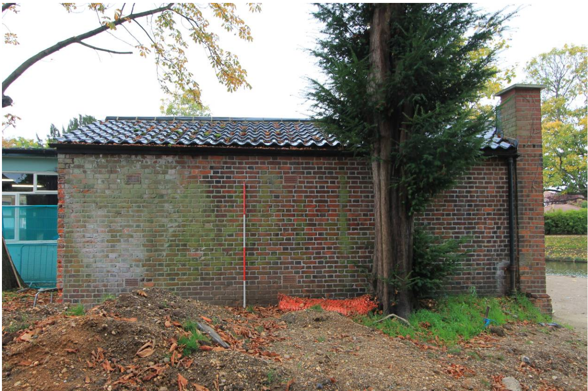
Plate 4 Northern elevation of the bath house, looking south
