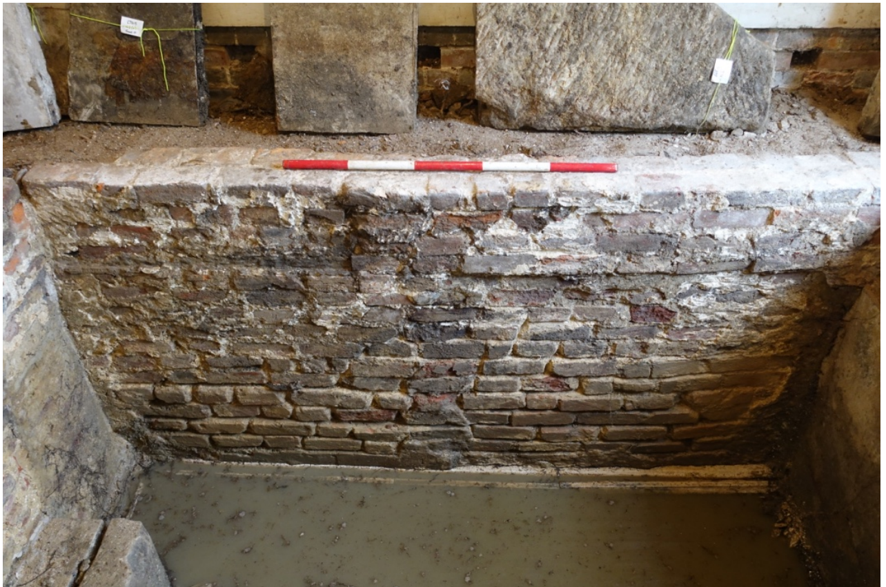
Plate 41 Detail of brick box, looking north
