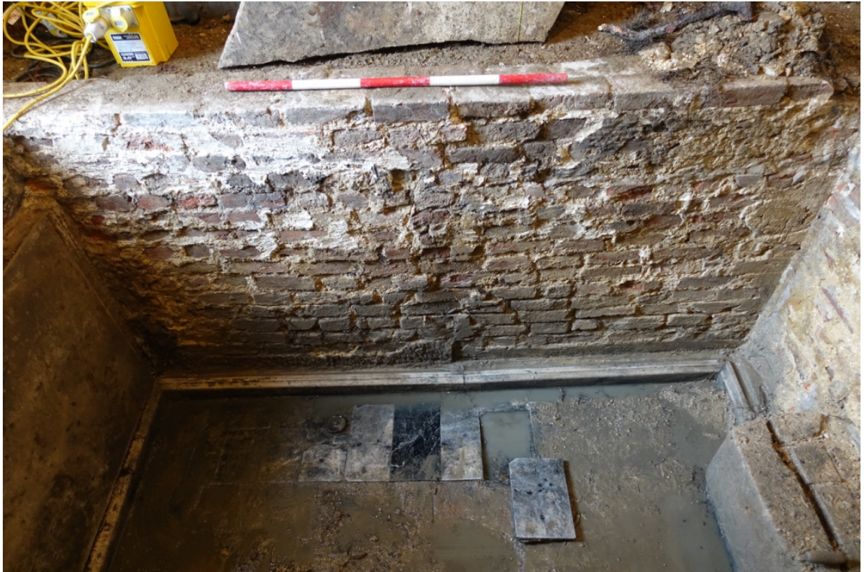
Plate 42 Detail of brick box, looking south
