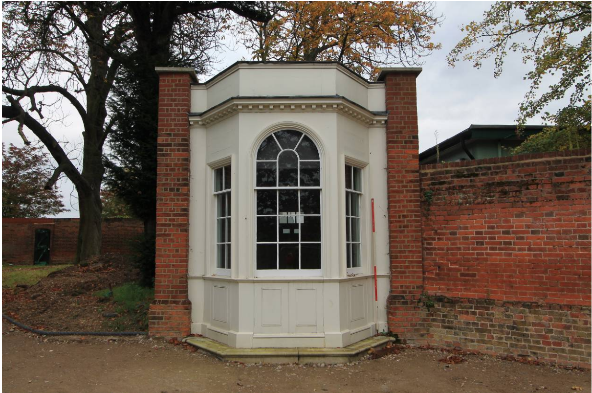
Plate 3 Canted western elevation of the bath house, looking east
