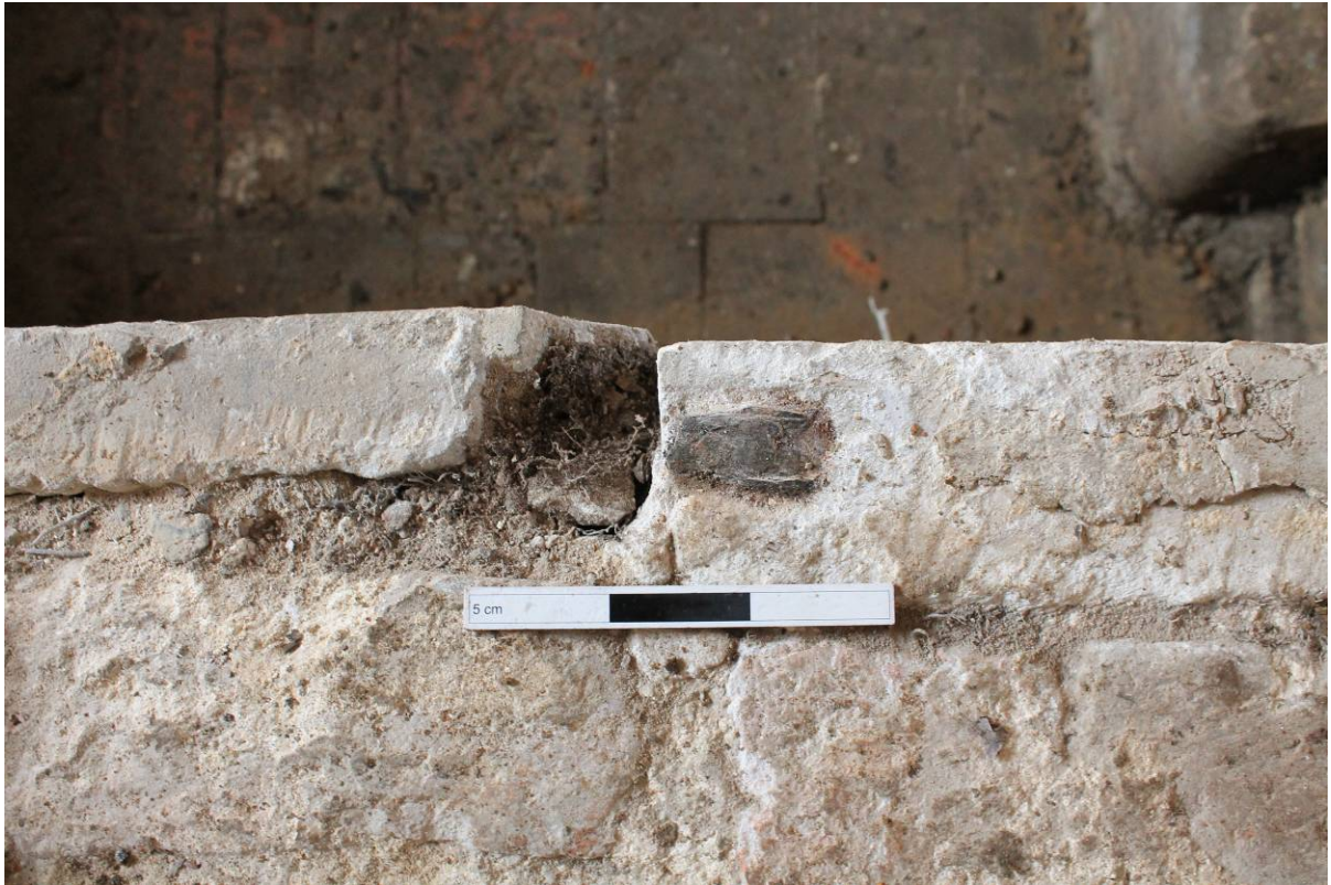
Plate 11 Remains of iron tie or 'staple' between Portland stones in the lining of the bath, looking south
