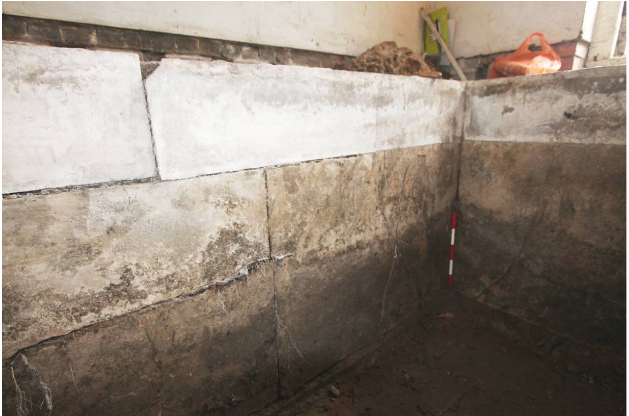
Plate 13 North wall of bath, looking north-east
