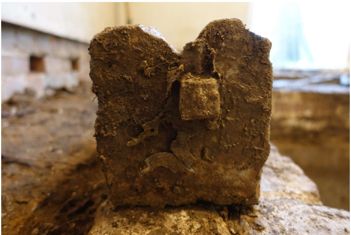
Plate 33 Square locating lead plug in end of plinth
