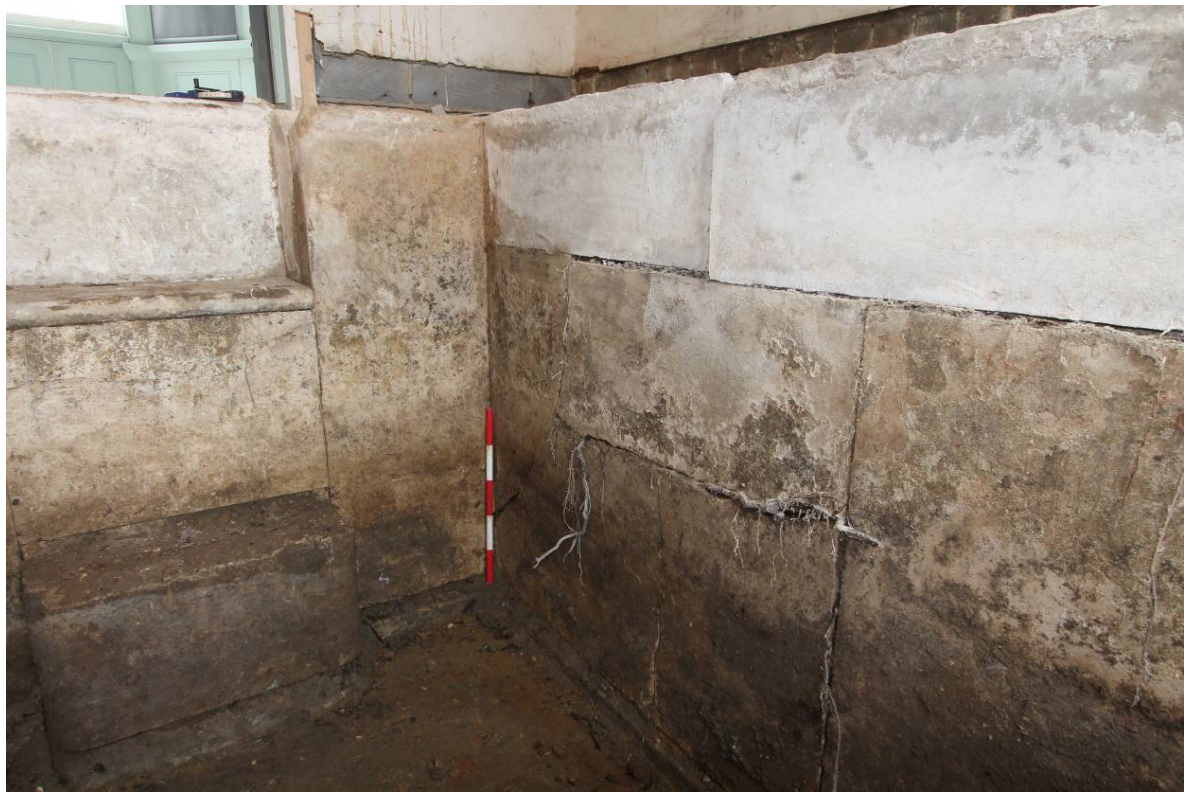
Plate 12 North wall of bath, looking north-west
