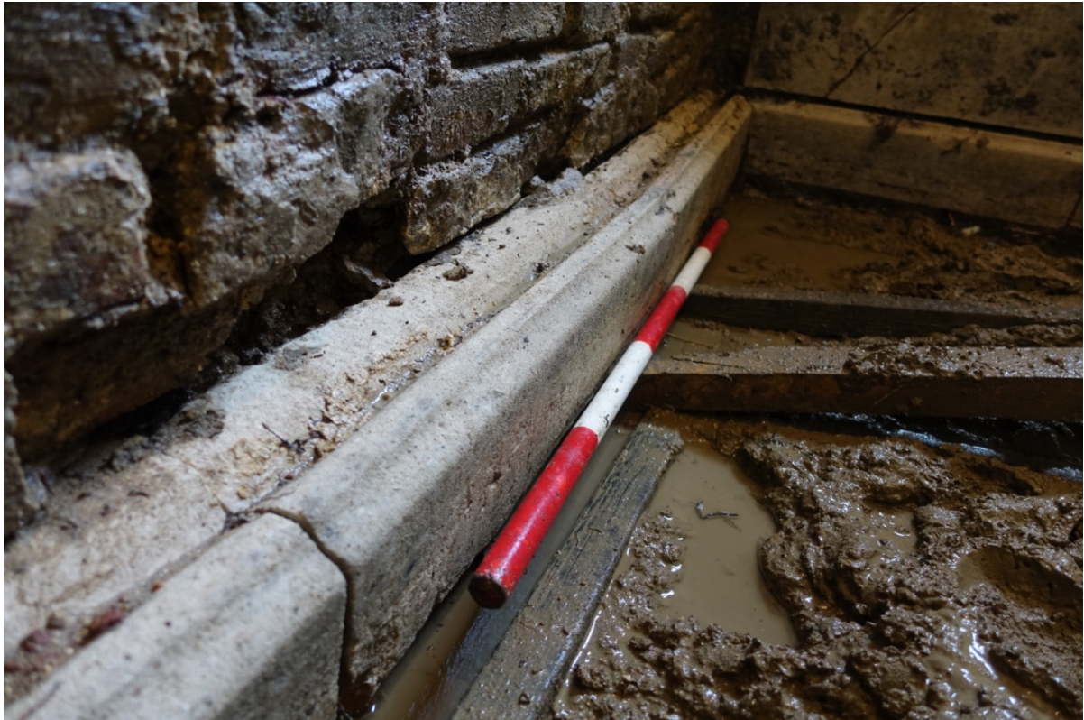
Plate 32 Recess or groove in the top of the plinth to receive stone lining, looking east
