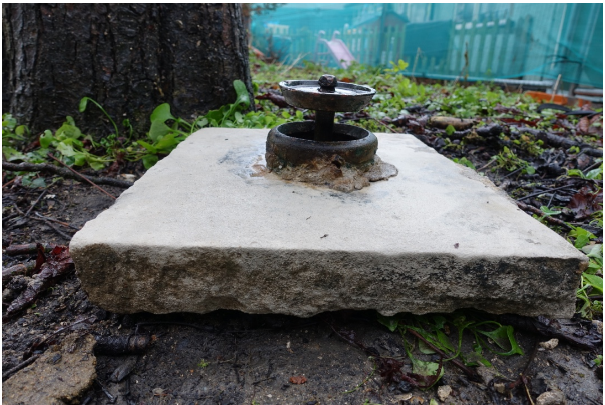
Plate 39 Detail of plug and stone mounting
