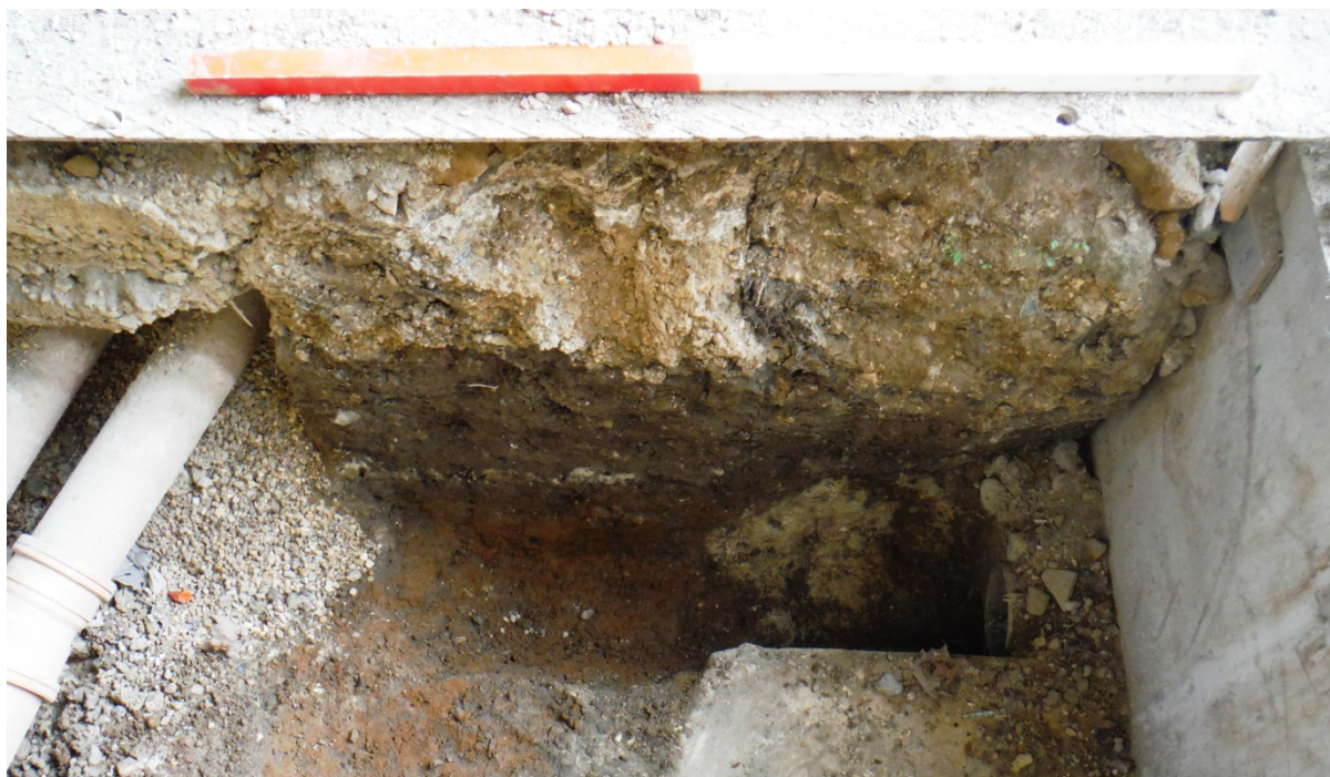
Plate 3: Pit [107], view northeast
