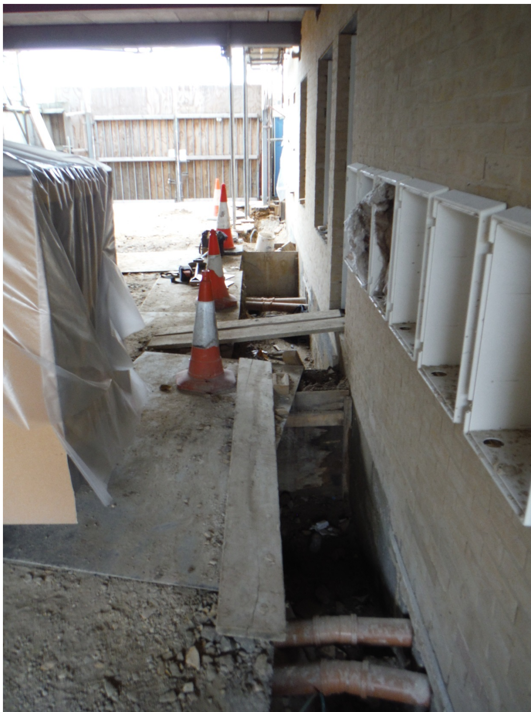
Plate 1: Exposed foundation footing, view southeast
