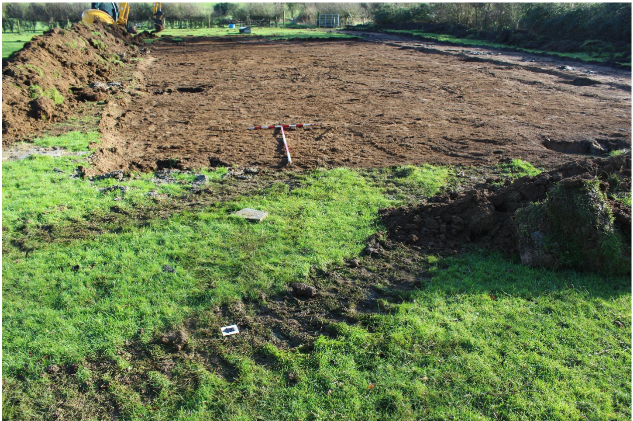
Plate 10: East-southeast facing shot of stripped barn and road area adjacent to barn footings. The subsoil (context 02) has been revealed in the barn footings area and topsoil (context 01) in the road area.
