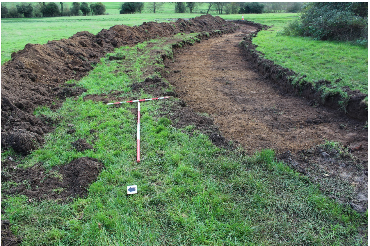
Plate 2: East facing shot of stripped road area.
