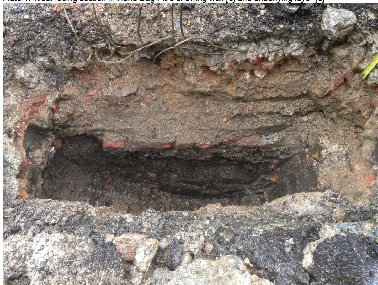
Plate 1: West-facing section in Hand Dug Pit 3 showing wall [6] and underlying layer [5]
