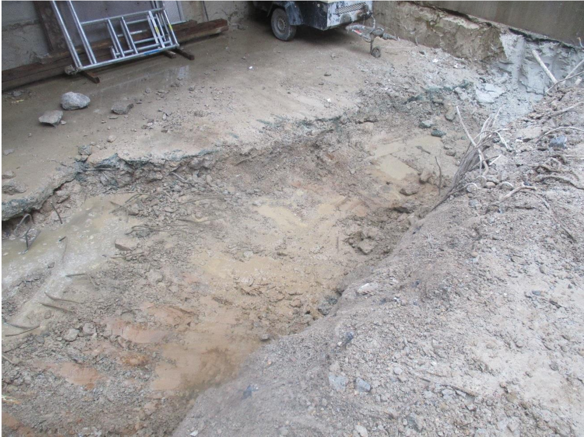
Plate 2: London Clay beneath lower basement slab
