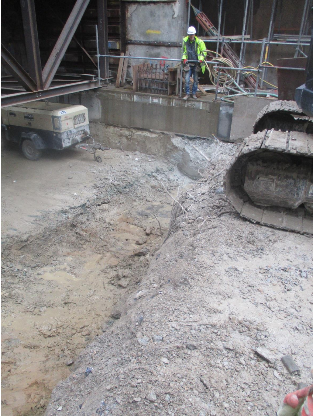
Plate 1: London Clay beneath lower basement slab
