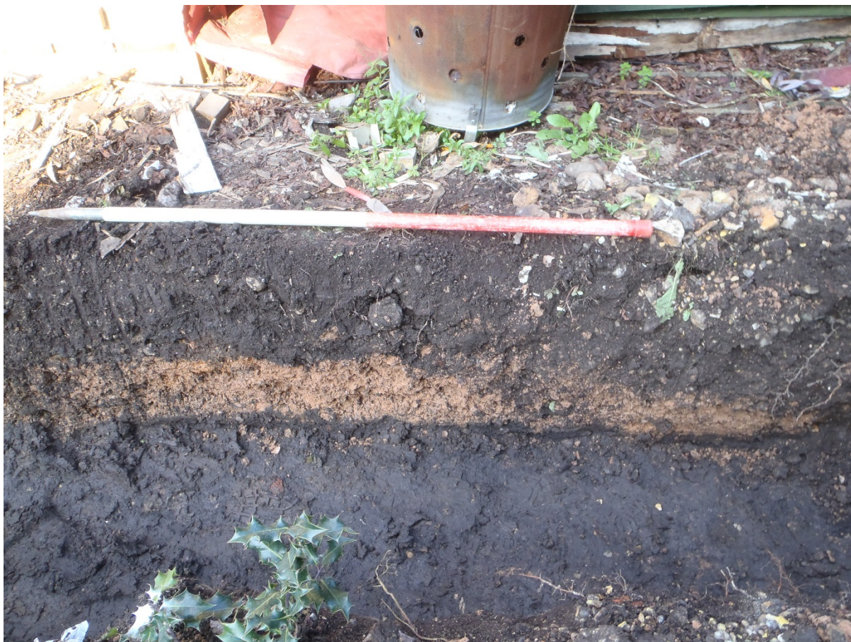
Plate 3: Section of foundation trench, view to north-east.
