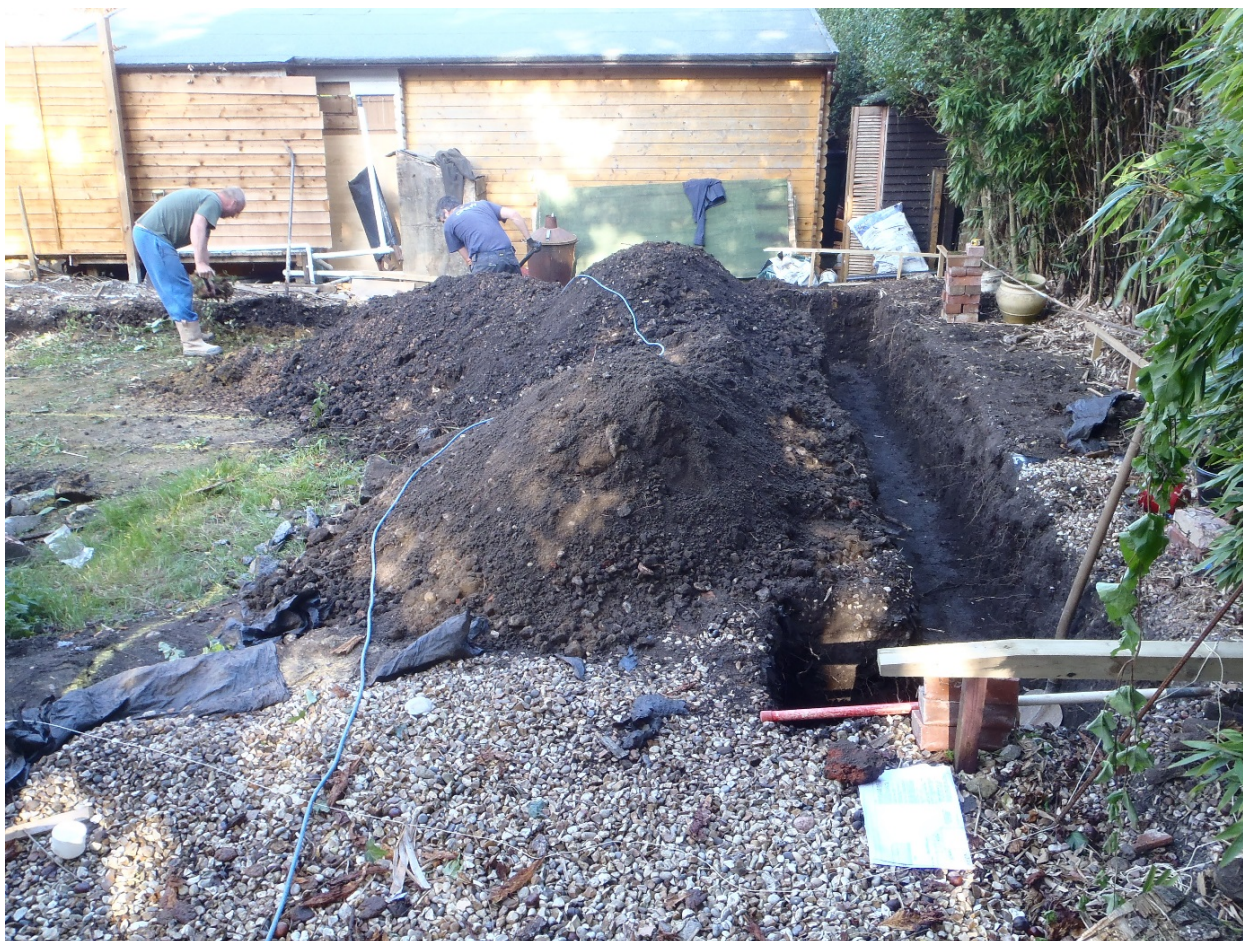
Plate 1: General view to the north-east.
