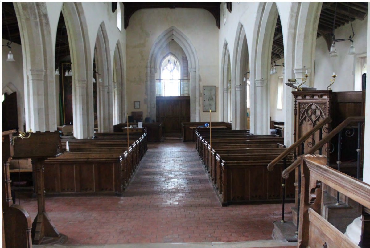
Plate 1: Main Aisle prior to removal of floor or pews
