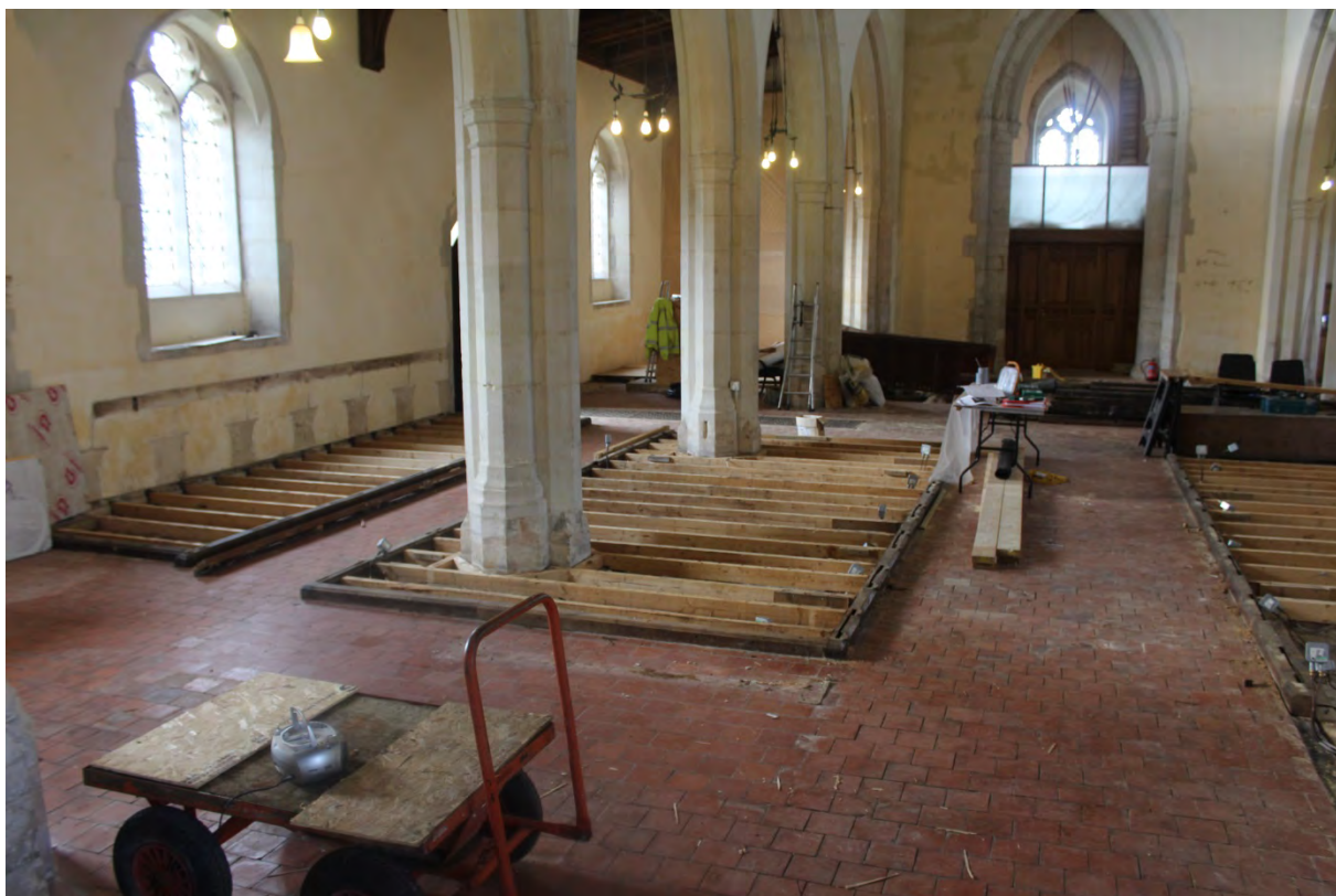
Plate 5: Main and South Aisle during pew removal
