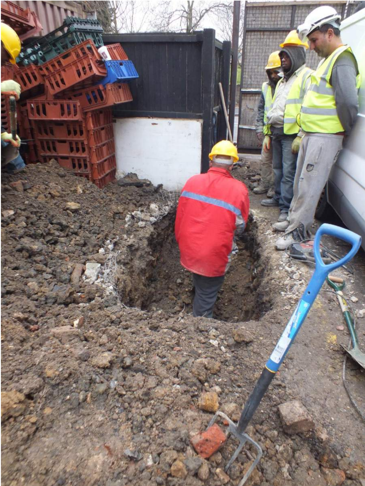
Plate 2: Shot showing excavation of Trench 2, looking west
